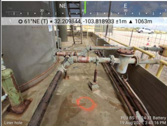
Photograph: 1 Date: 8/19/2025 Description: Hole in Liner before cleaning activities View: Northeast
