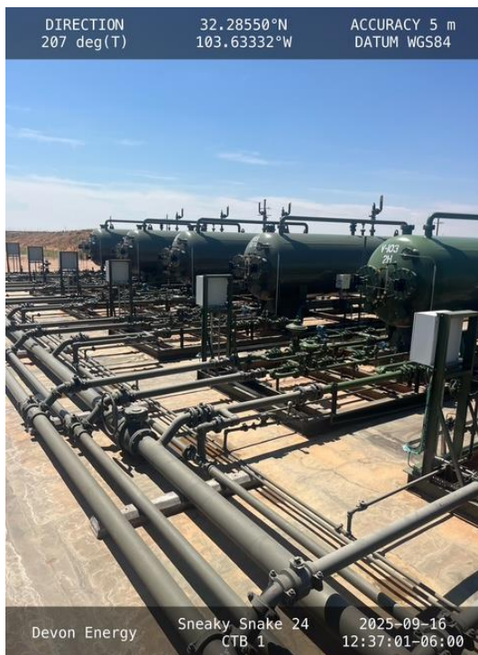
Photo 9 View of containment facing southwest.
