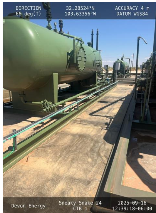
Photo 10 View of containment facing northeast.
