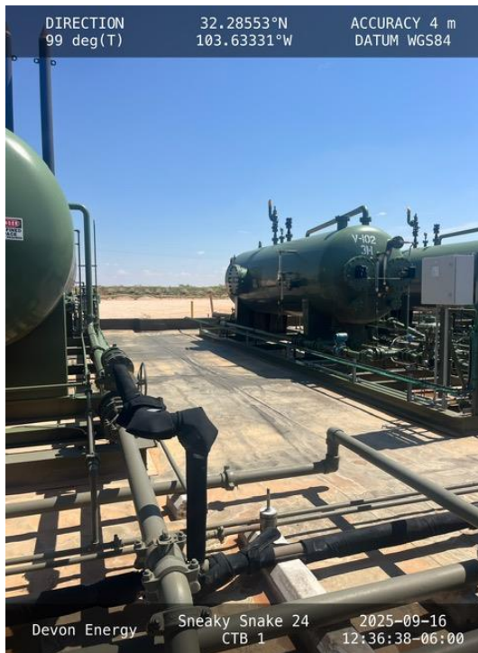
Photo 5 View of containment facing east.
