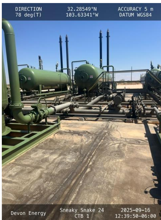
Photo 13 View of containment facing northeast.
