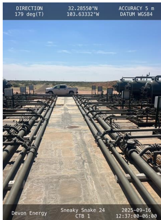
Photo 8 View of containment facing south.
