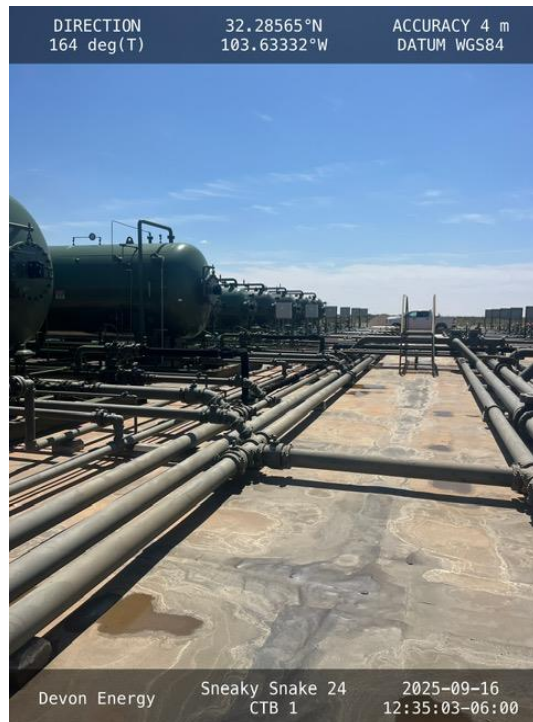
Photo 2 View of containment facing south.
