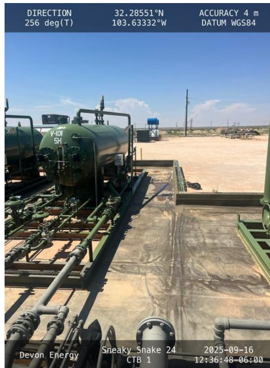
Photo 6 View of containment facing west.
