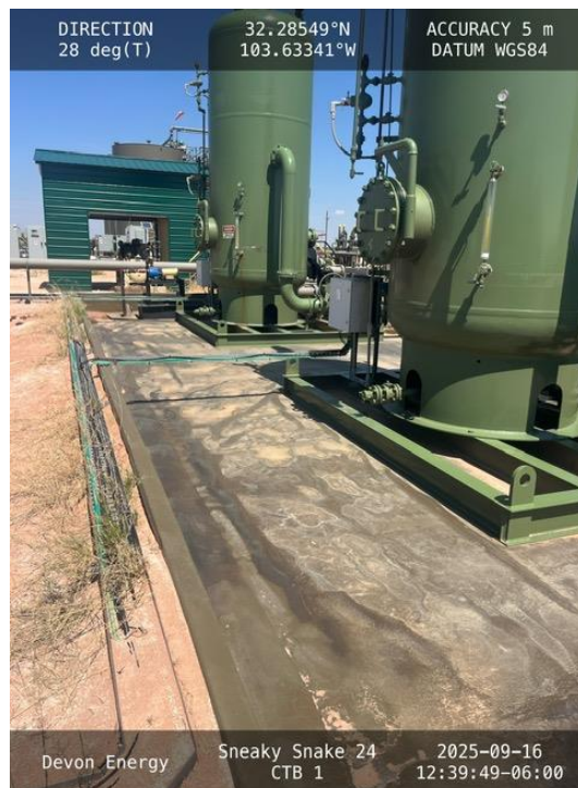
Photo 12 View of containment facing northeast.
