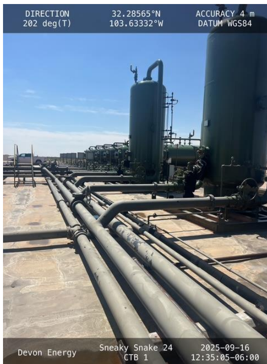
Photo 1 View of containment facing south.
