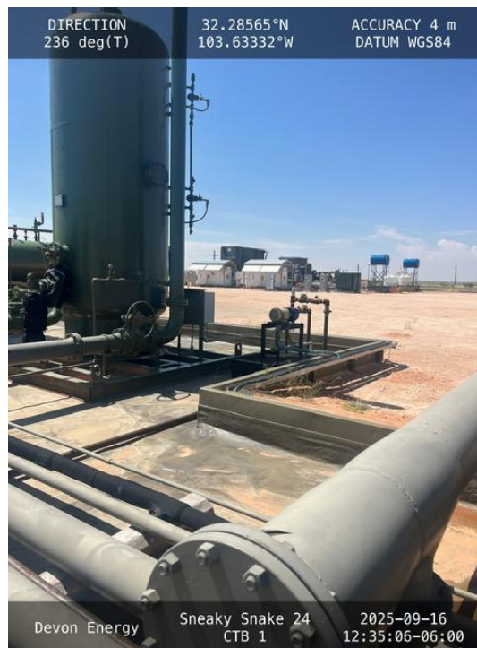
Photo 2 View of containment facing southwest.
