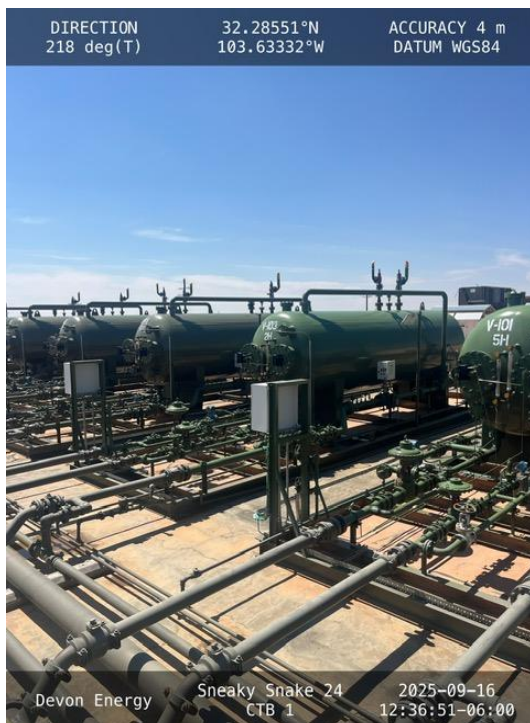
Photo 7 View of containment facing southwest.
