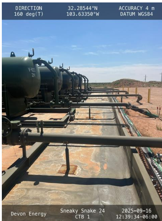
Photo 11 View of containment facing south.
