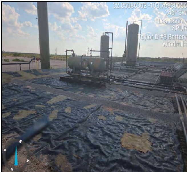
Photo of location taken after windrolls were laid facing southwest.
