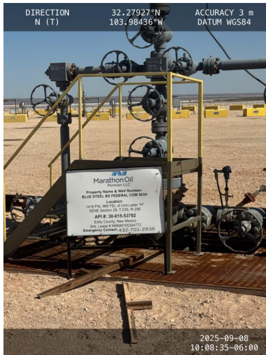
Photo 1 View of Site location.
