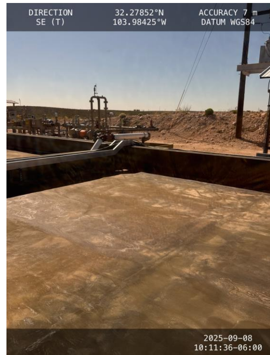
Photo 6 View of southeast corner of containment facing southeast.
