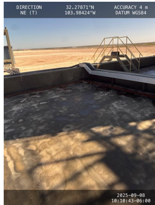
Photo 2 View of northeast corner of containment facing northeast.
