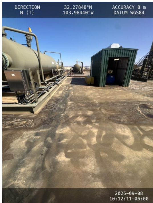
Photo 9 View of central portion of containment facing north.
