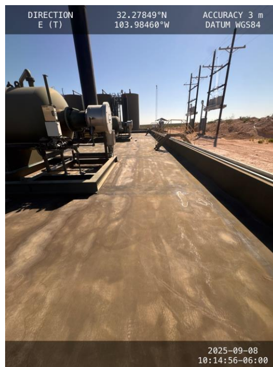
Photo 14 View of southern portion of containment facing east.
