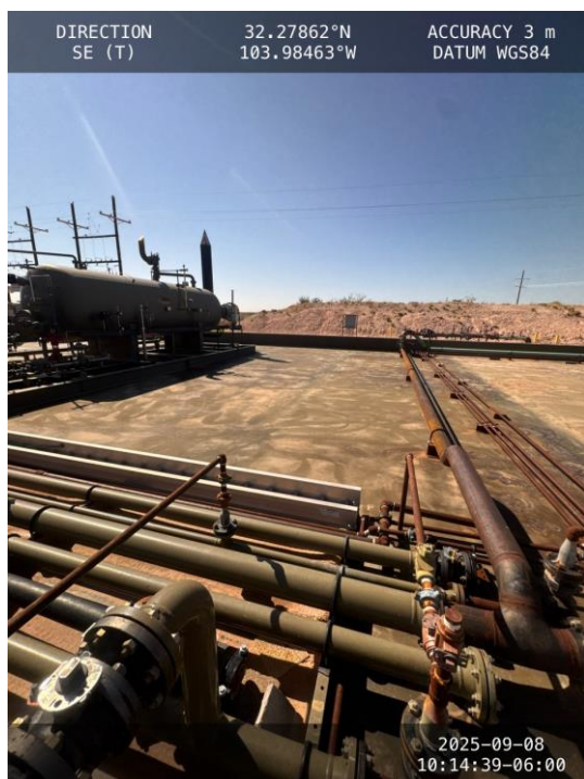
Photo 13 View of central portion of containment facing southeast.
