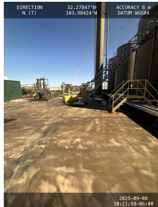
Photo 8 View of eastern portion of containment facing north.
