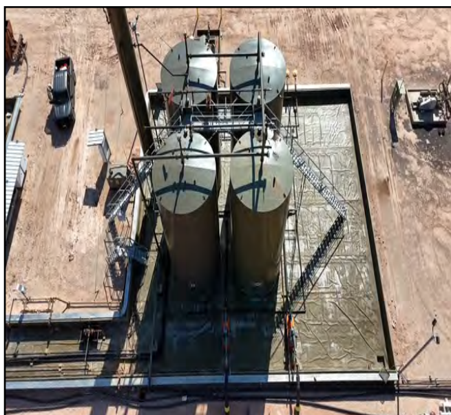
Aerial photos taken before powerwash.
