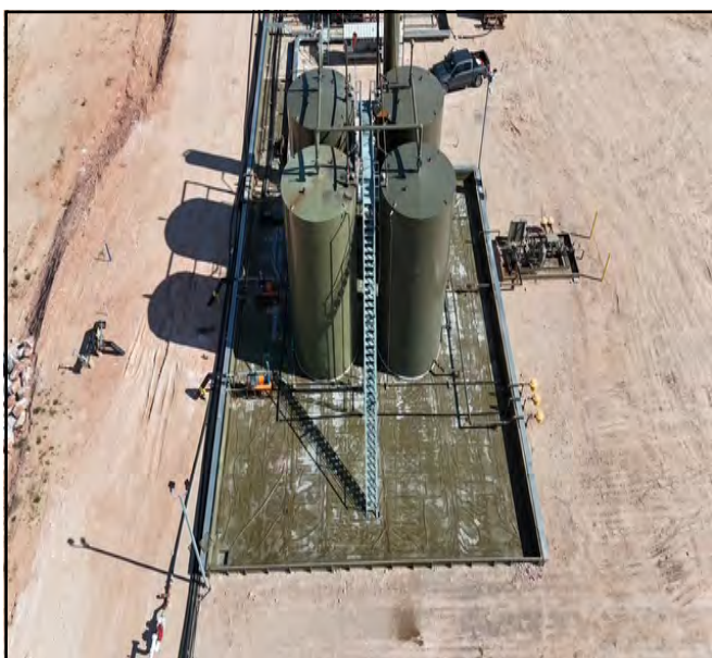
Aerial photos taken before powerwash.
