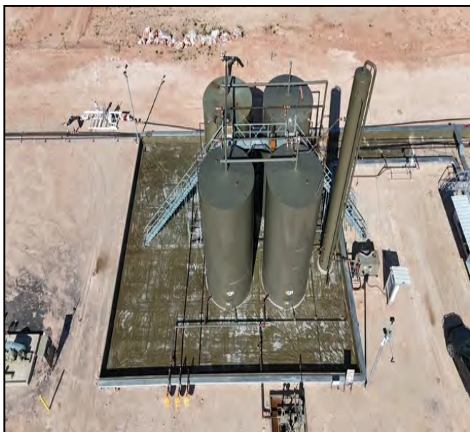
Aerial photos taken before powerwash.
