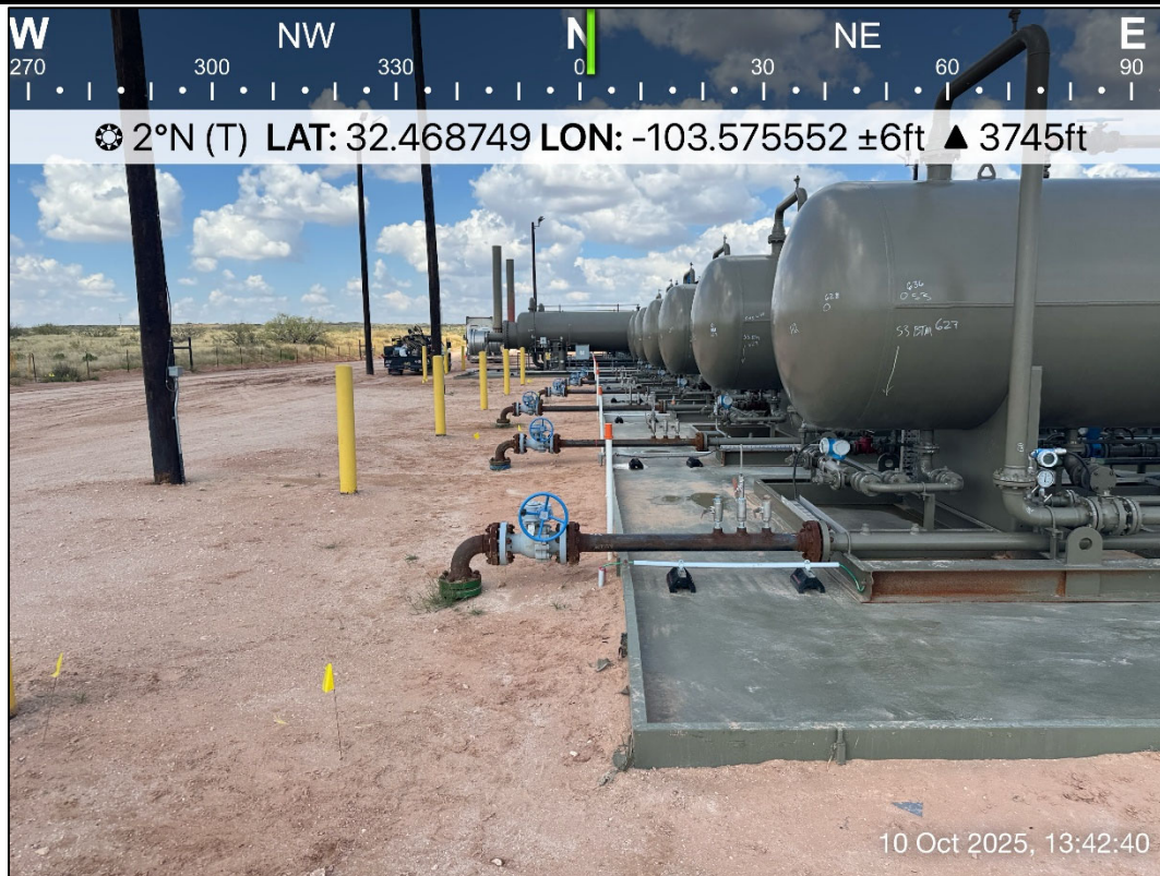
PHOTO 1: Northern view outside of containment during liner inspection activities .10/10/2025
