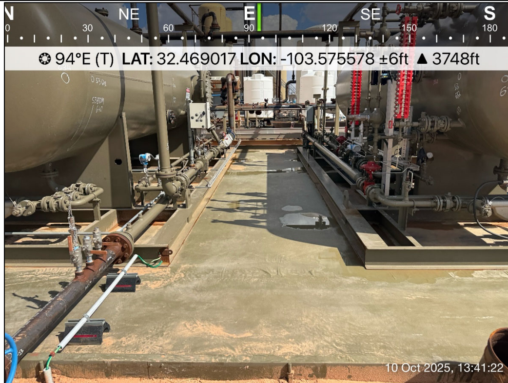
PHOTO 9: Eastern view outside of containment during liner inspection activities following pressure washing. 10/10/2025
