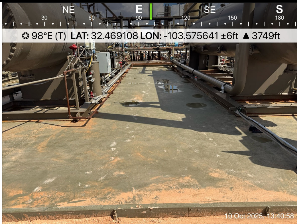
PHOTO 10: Eastern view outside of containment during liner inspection activities following pressure washing. 10/10/2025
