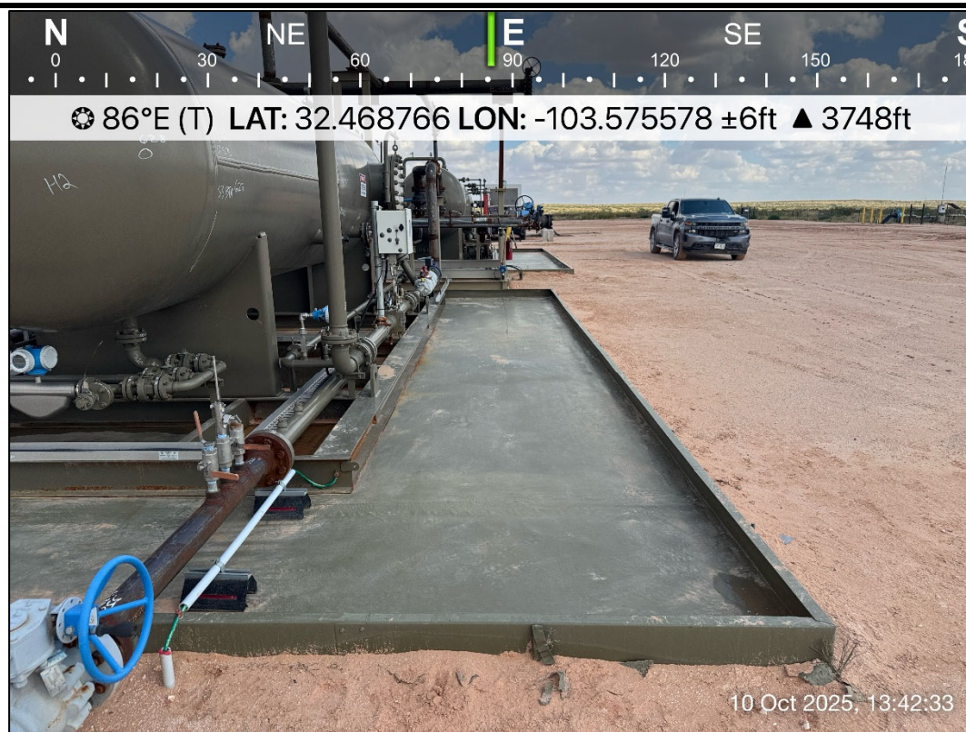
PHOTO 2: Eastern view outside of containment during liner inspection activities. 10/10/2025
