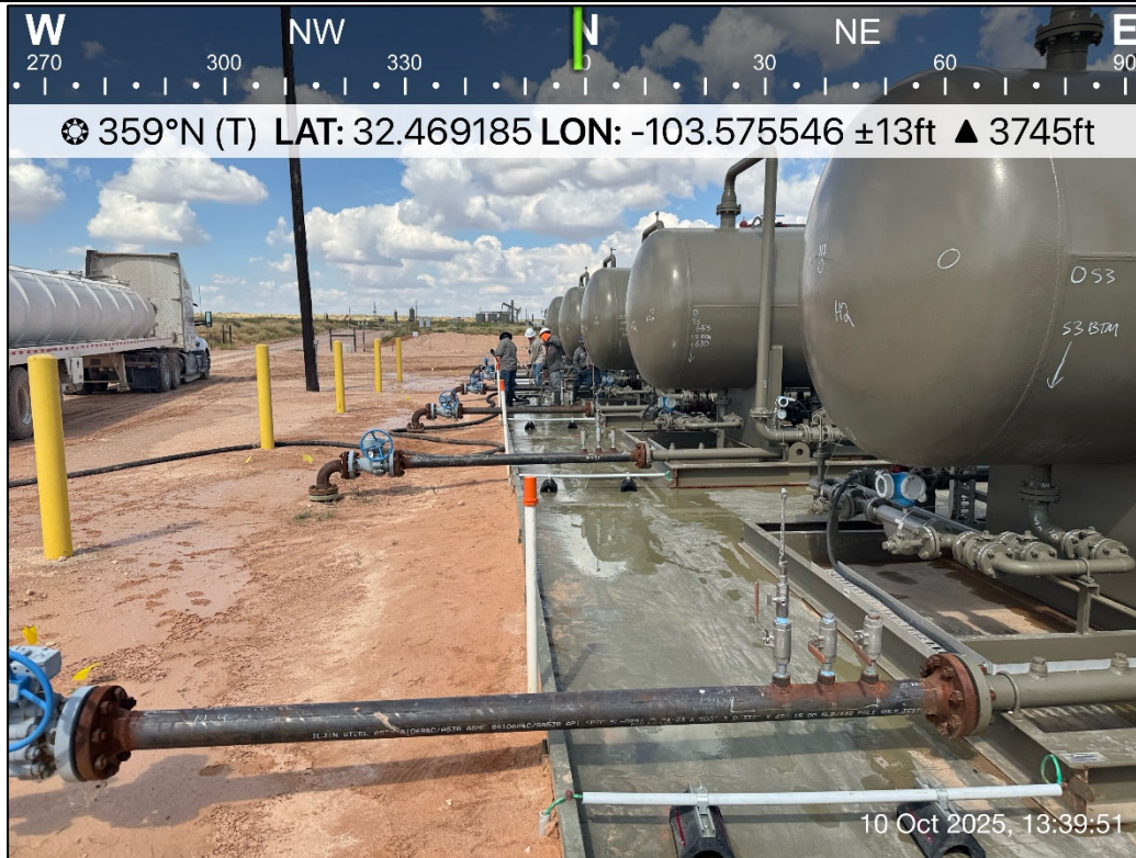
PHOTO 5: Northern view outside of containment during liner inspection activities following pressure washing. 10/10/2025
