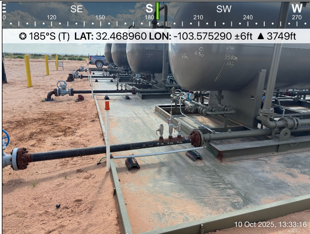
PHOTO 13: Southern view during liner inspection activities. 10/10/2025
