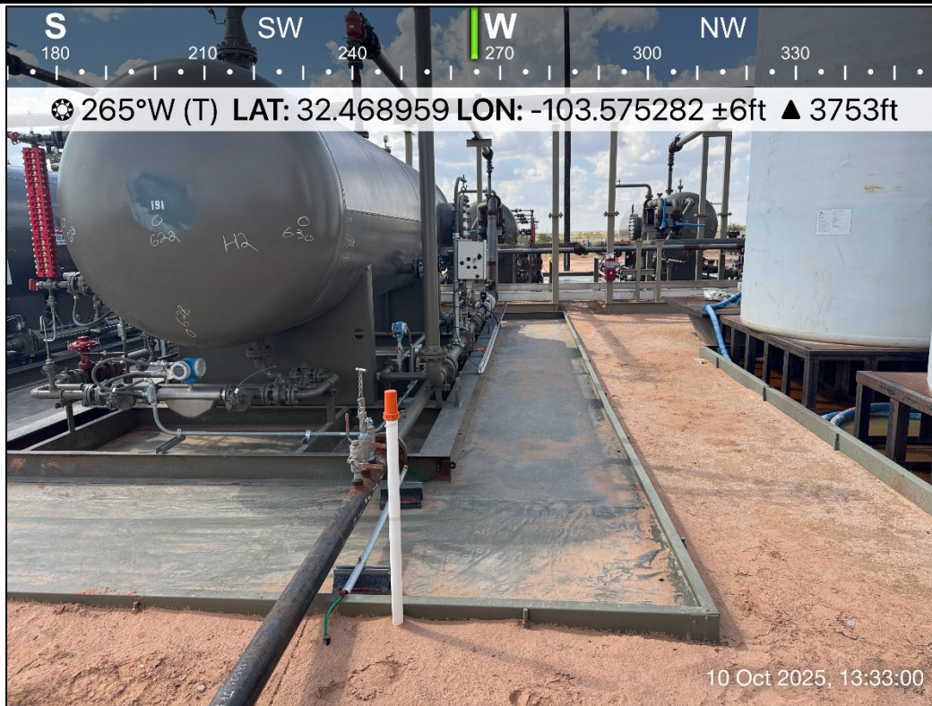
PHOTO 11: Western view during liner inspection activities. 10/10/2025
