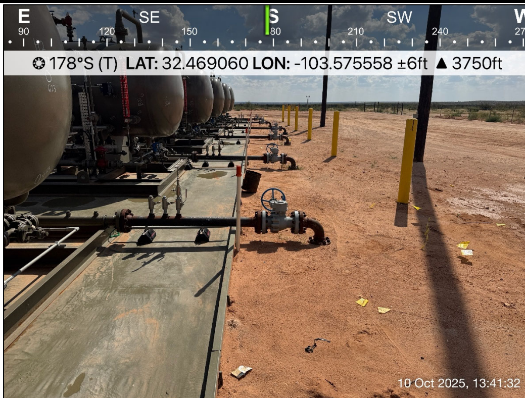
PHOTO 3: Southern view outside of containment during liner inspection activities. 10/10/2025
