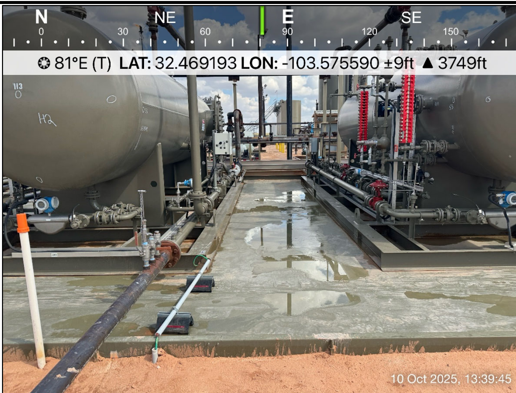
PHOTO 6: Eastern view outside of containment during liner inspection activities following pressure washing. 10/10/2025
