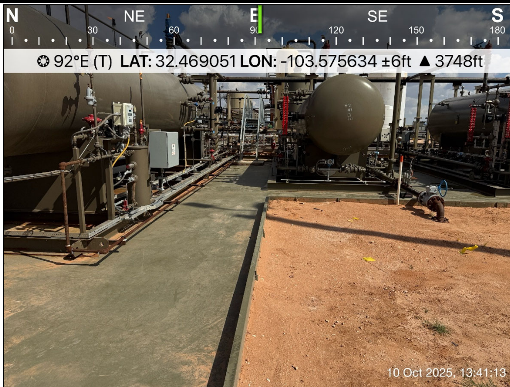
PHOTO 7: Eastern view during liner inspection activities. 10/10/2025
