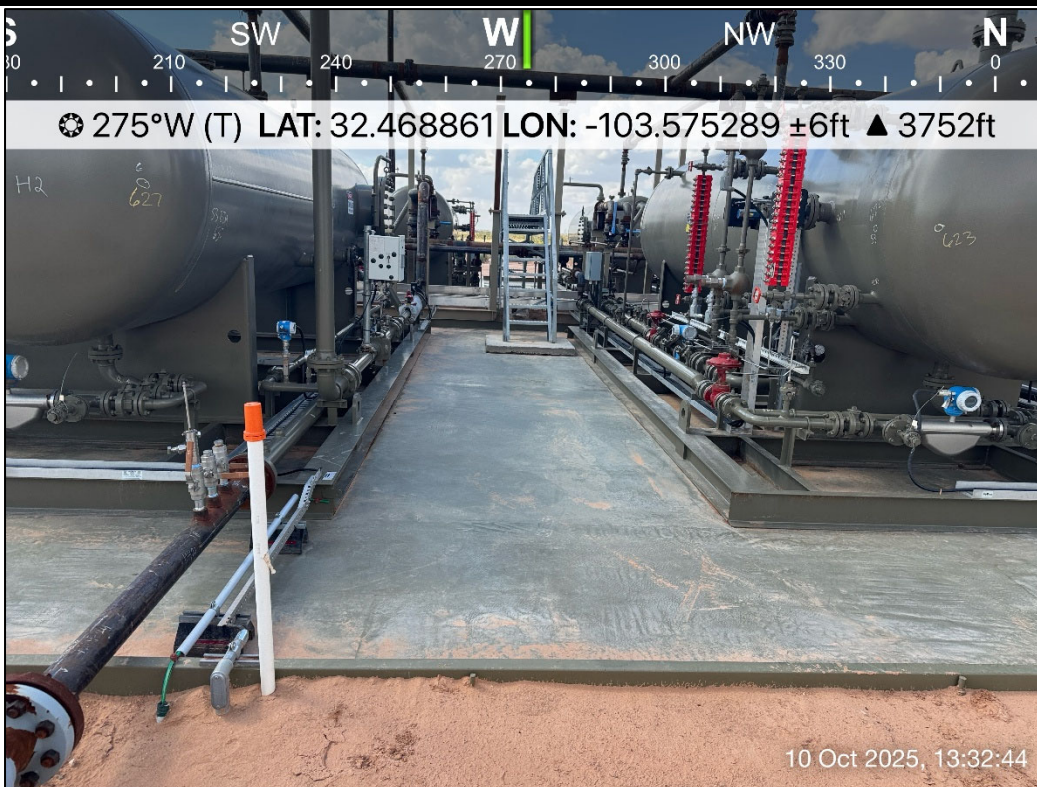
PHOTO 14: Western view during liner inspection activities. 10/10/2025
