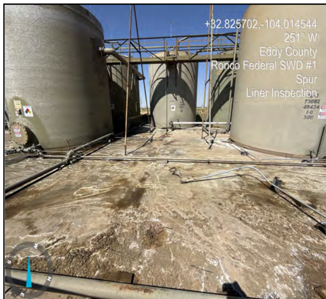
Photo of liner taken during initial liner inspection facing west.
