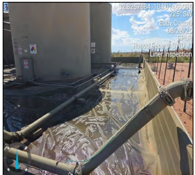
Photo of location taken post power wash facing southwest.
