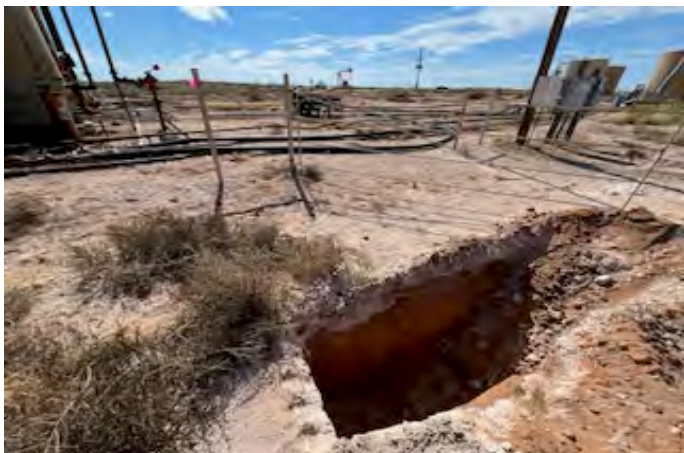
View to SW of test hole TH-21 (10/16/25).
