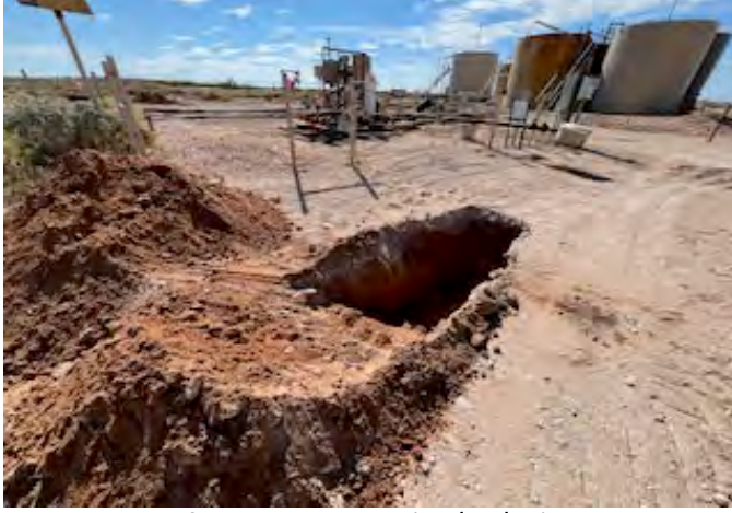
View to SW of test hole TH-23 (10/16/25).
