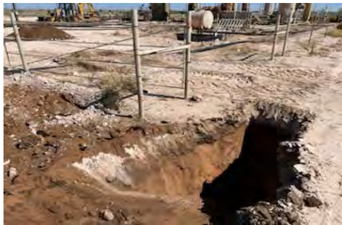
View to NE of test hole TH-17 (10/16/25).
