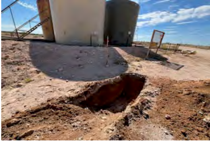
View to SW of test hole TH-31 (10/16/25).
