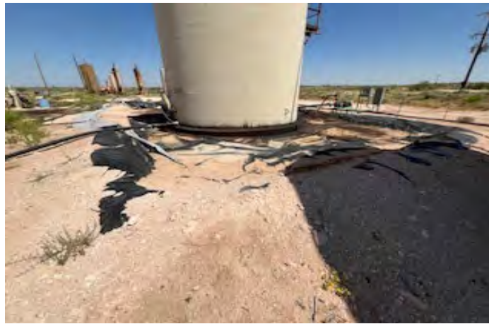
View to E of liner at water tank (8/7/25).
