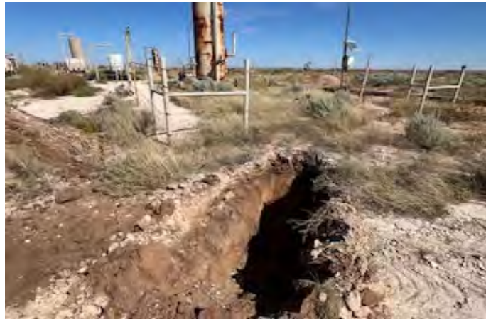
View to NE of test hole TH-14 (10/16/25).
