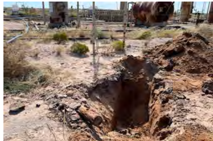
View to S of test hole TH-20 (10/16/25).
