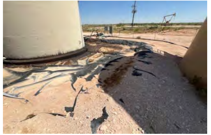
View to S of liner at water tank (8/7/25).
