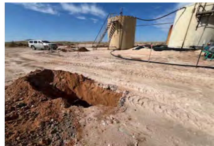
View to NW of test hole TH-28 (10/16/25).
