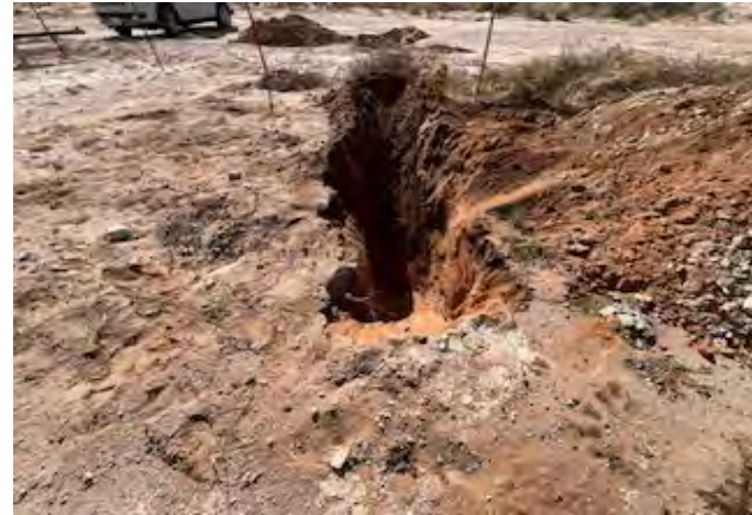
View to SW of test hole TH-30 (10/16/25).
