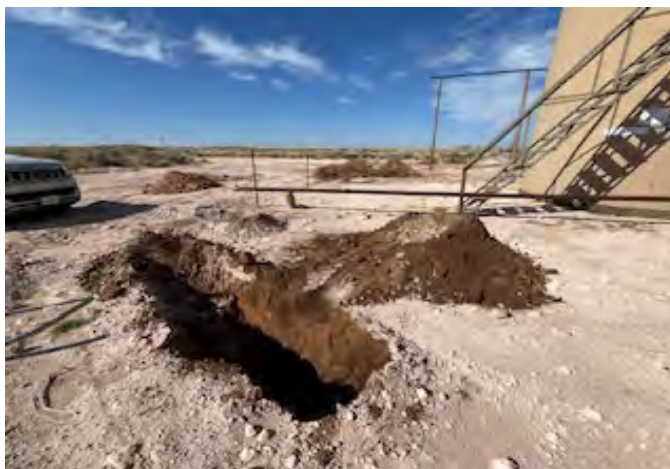
View to NW of test hole TH-29 (10/16/25).
