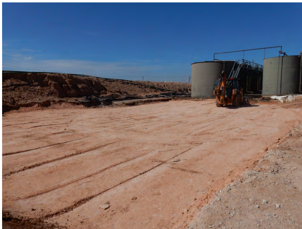
Backfill of Excavation Viewing Southwest, August 22, 2017
