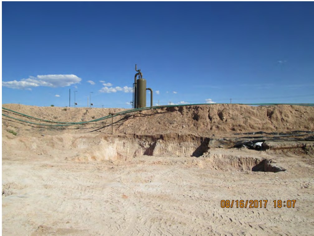
Final Excavation Area Viewing South, August 16, 2017
