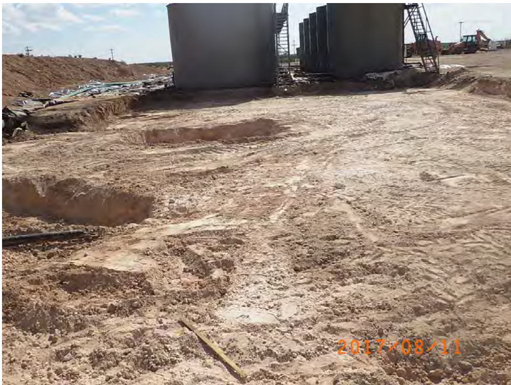
Excavation Area Viewing West, August 11, 17
