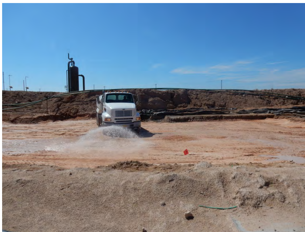
Water Packing of Excavation Viewing South, August 22, 2017
