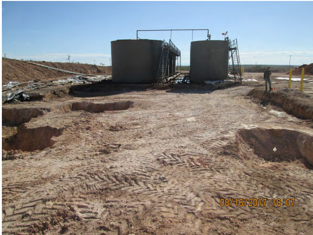
Final Excavation Area Viewing West, August 16, 2017
