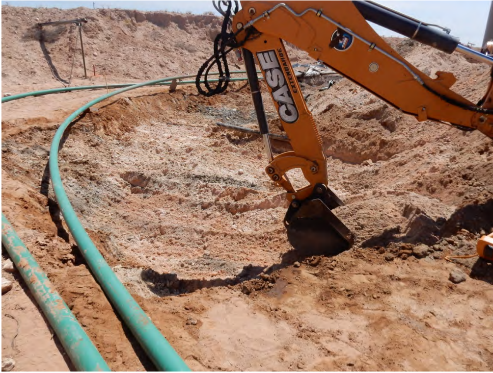
Soil Excavation near DP-7 Viewing Southwest, August 10, 2017
