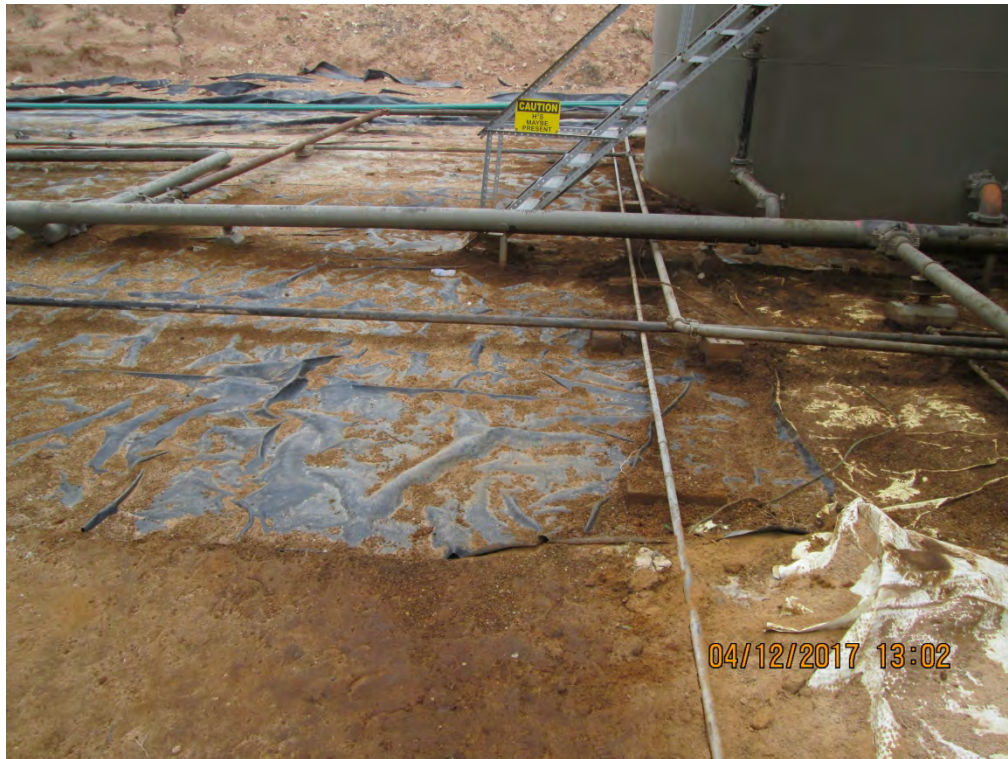
Location Viewing South Prior to Excavation, April 12, 2017
