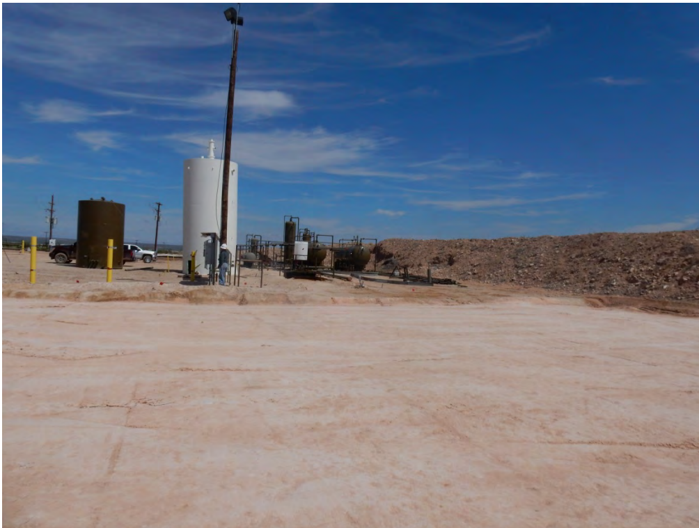
Final Backfill Viewing North, August 23, 2017
