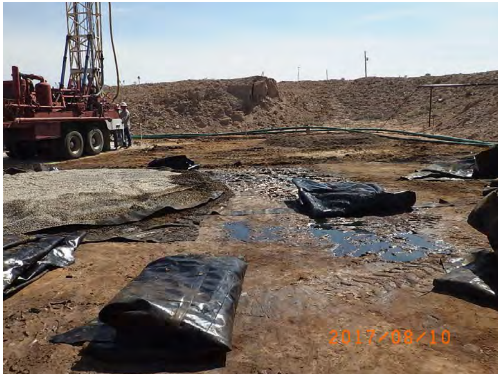
Location Viewing East Prior to Remediation and Chloride Delineation at DP-11, August 10, 2017
