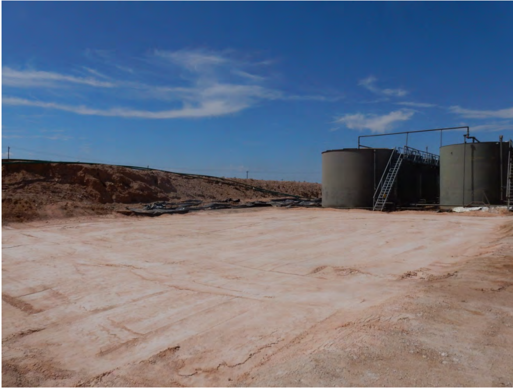
Final Backfill Viewing Southwest, August 23, 2017
