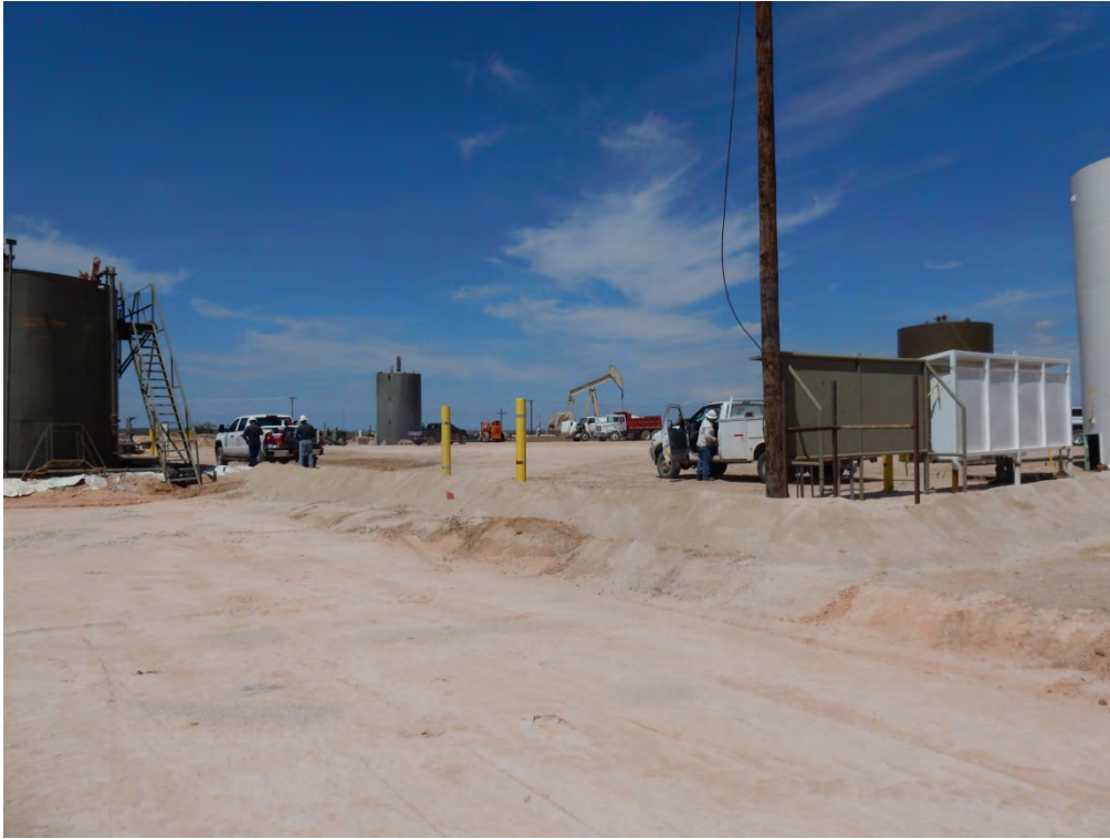
New Firewall Viewing Northwest, August 23, 2017
