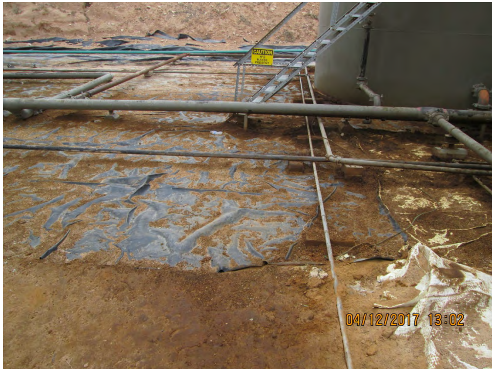
Location Viewing South Prior to Excavation, April 12, 2017
