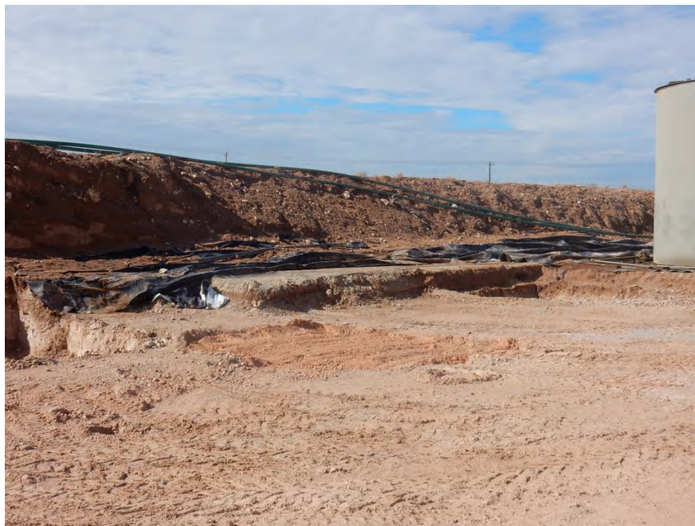
Backfill of Excavation Viewing Southwest, August 21, 2017
