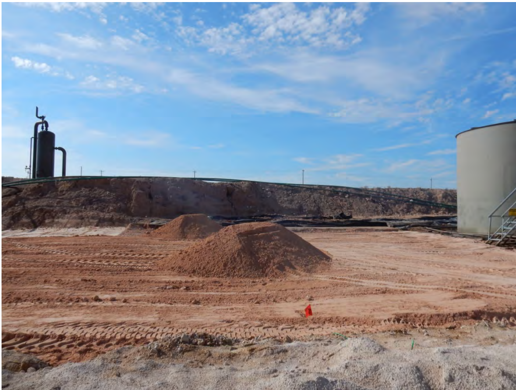
Backfill of Excavation Viewing South, August 23, 2017
