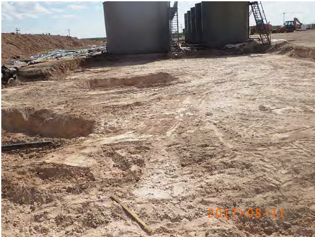
Excavation Area Viewing West, August 11, 17
