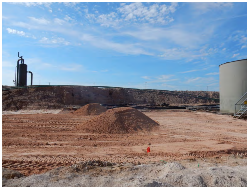
Backfill of Excavation Viewing South, August 23, 2017
