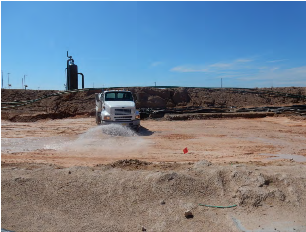
Water Packing of Excavation Viewing South, August 22, 2017
