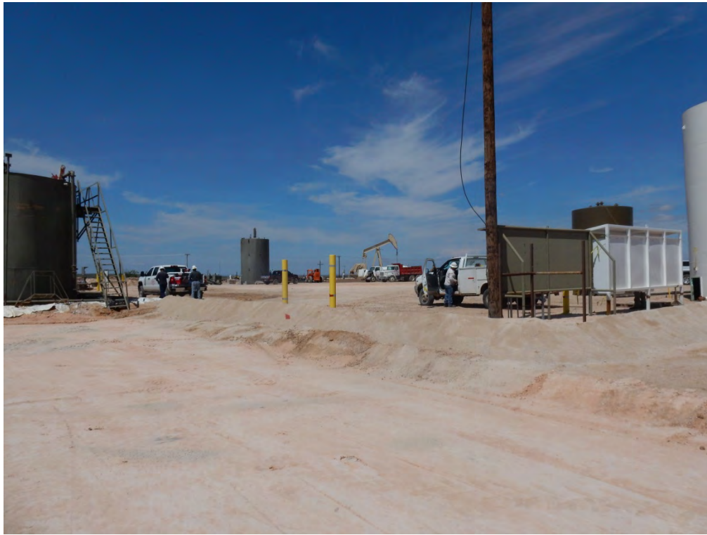
New Firewall Viewing Northwest, August 23, 2017
