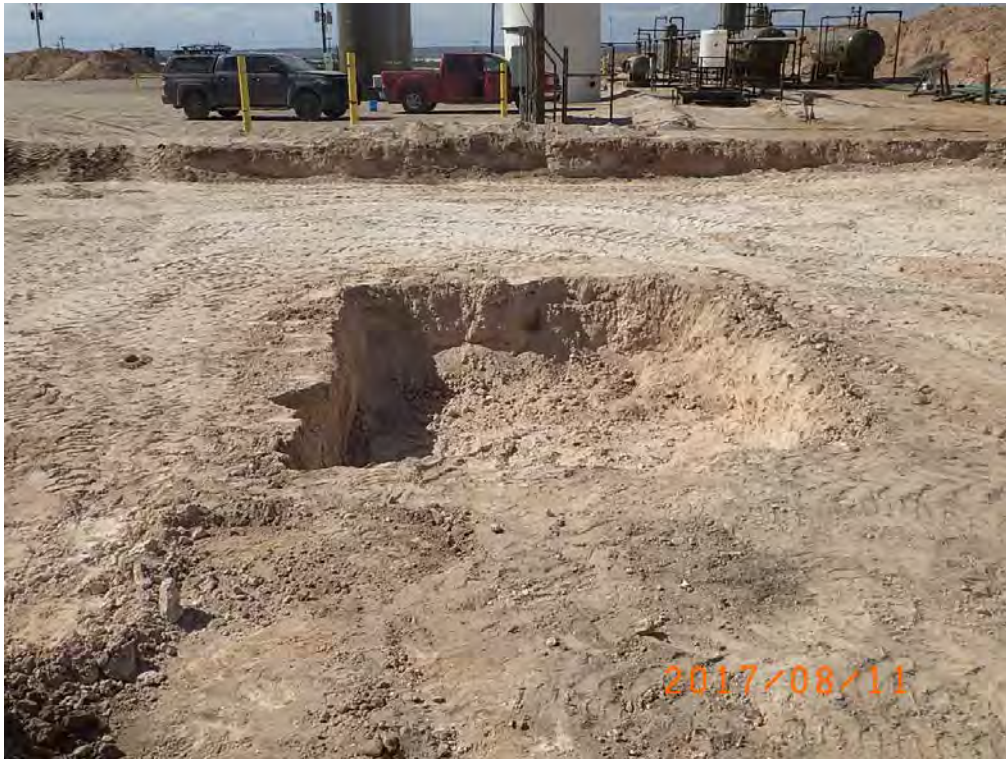
Soil Excavation at S-15 Viewing North, August 11, 2017
