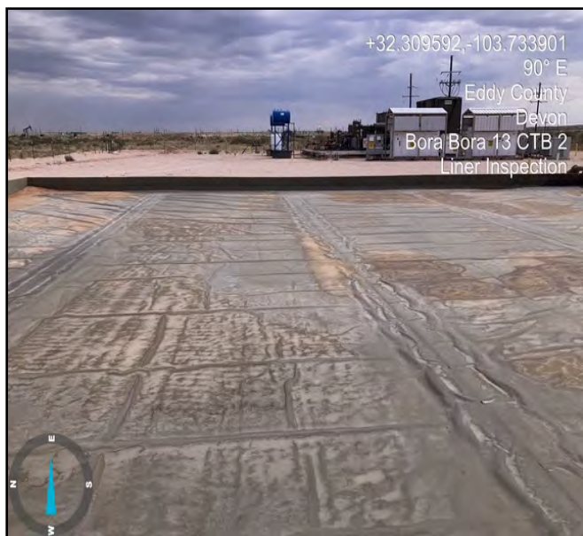
Photo of liner inspection post pressure washing facing east.
