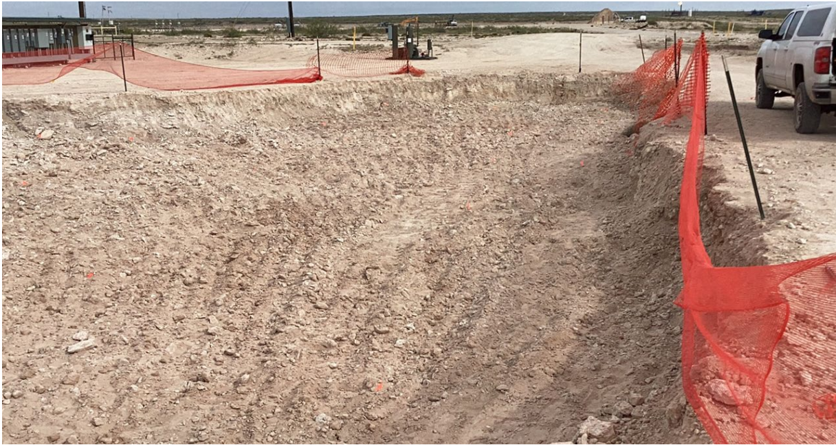
Photo 7 View to the east at the eastern portion of the remedial excavation following over-excavation activities.
