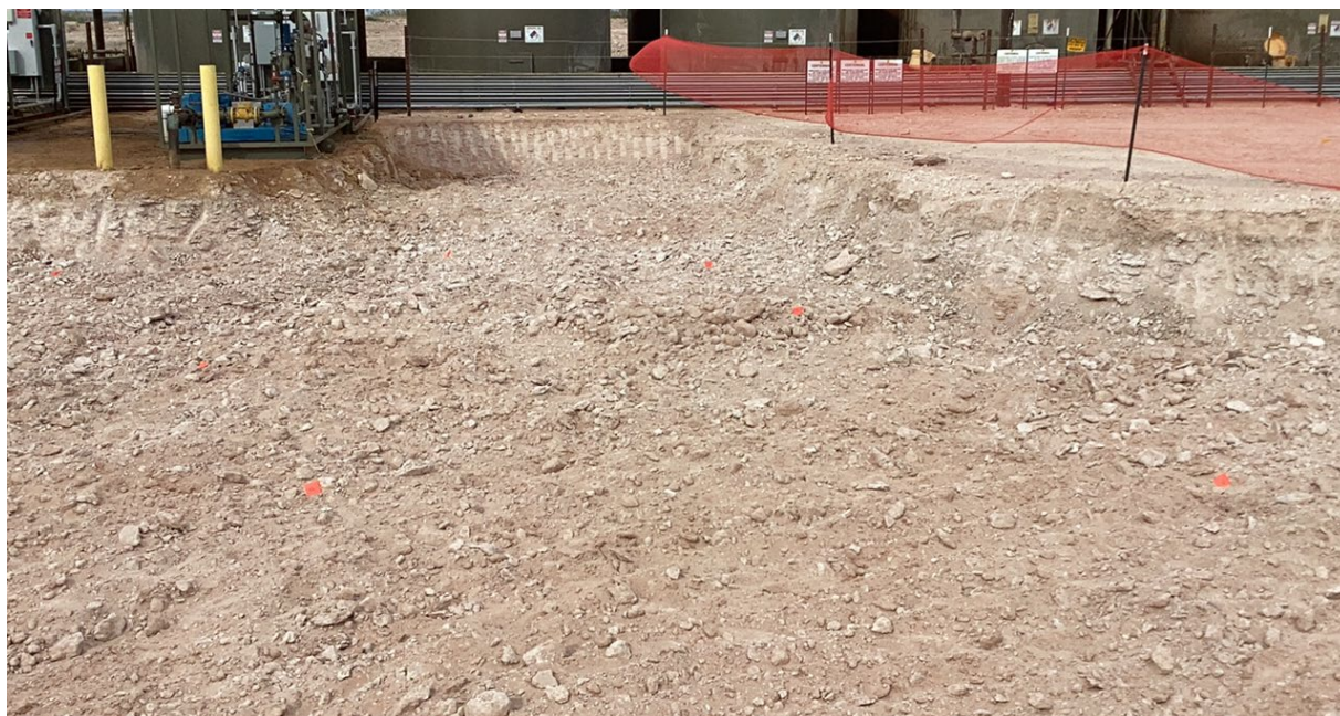
Photo 6 View to the north at the eastern portion of the remedial excavation following over-excavation activities.
