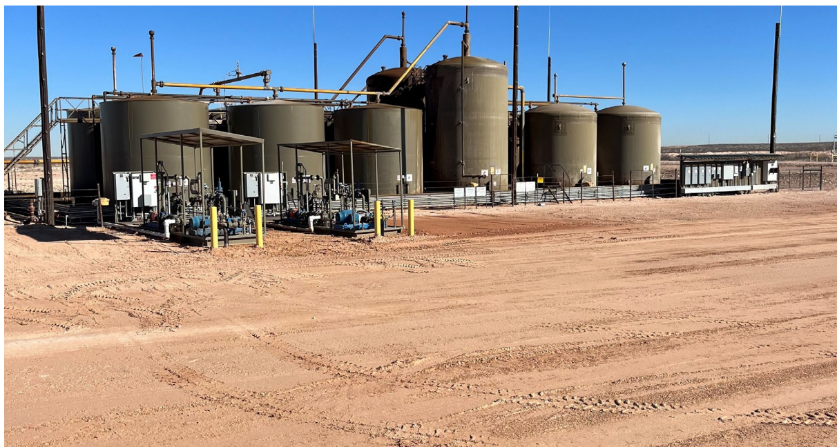
Photo 10 View to the northeast following backfill and site restoration activities.
