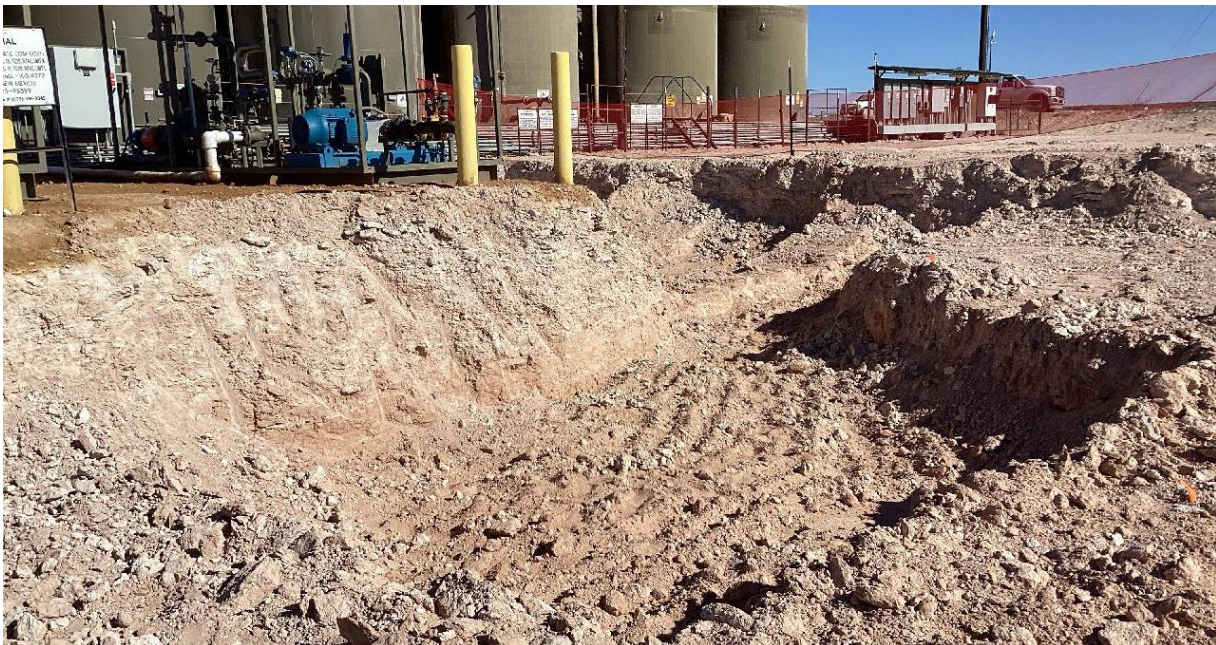
Photo 8 View to the northeast following additional over-excavation activities.
