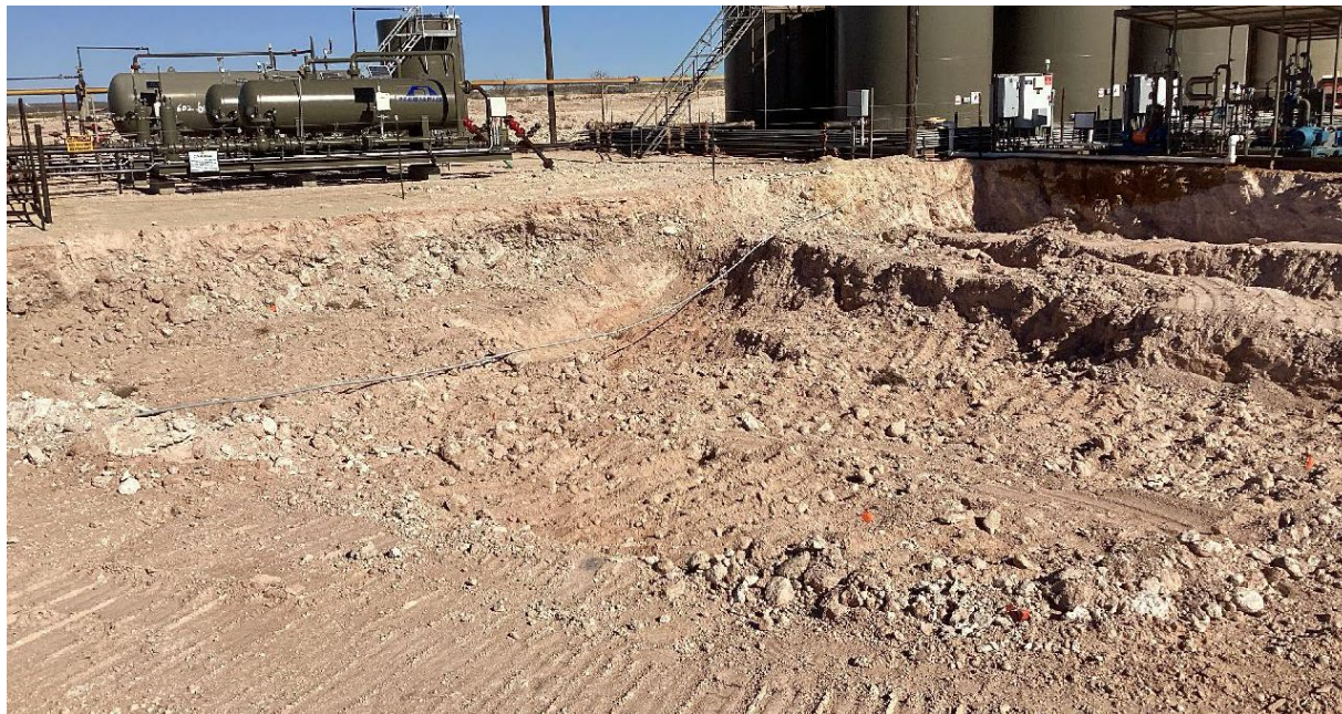
Photo 9 View to the northeast following additional over-excavation activities.
