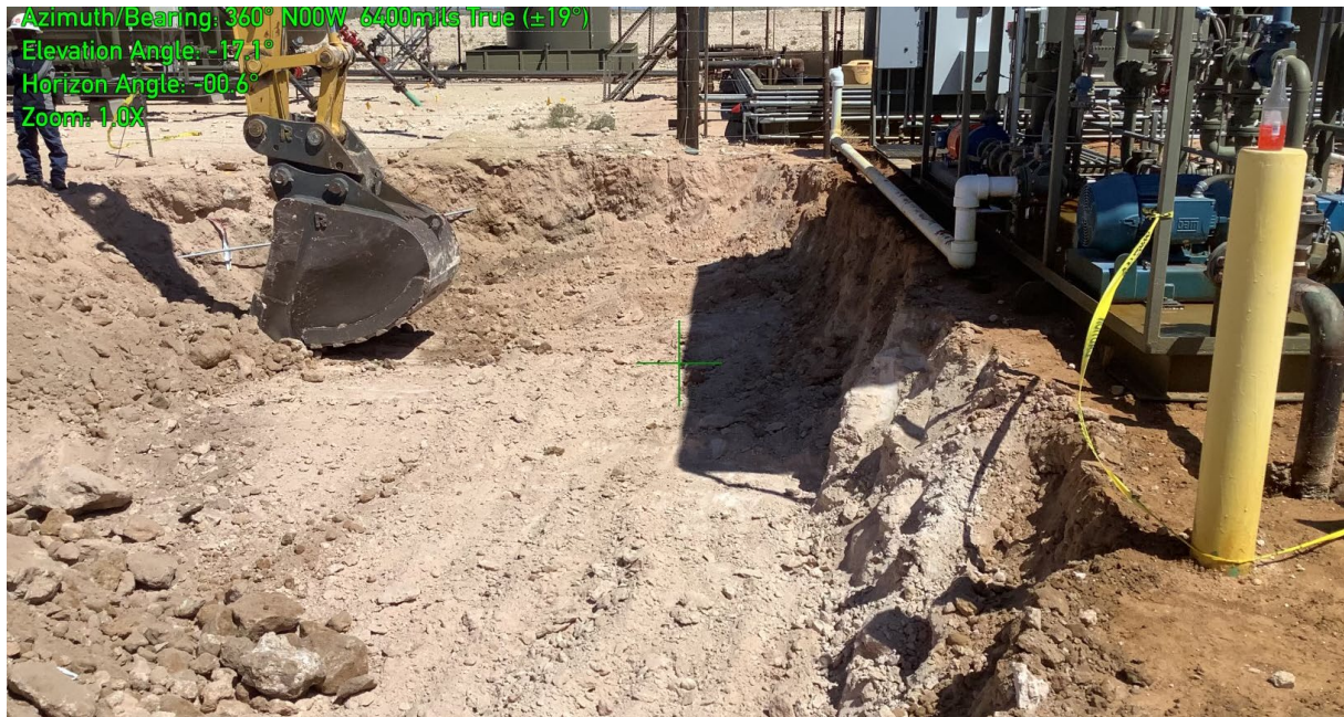
Photo 3 View of the LACT Units during remedial excavation activities.
