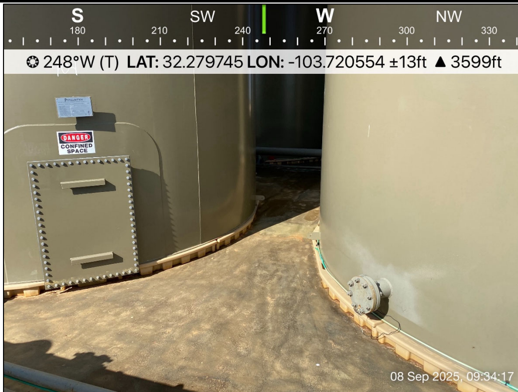
PHOTO 19: Southwestern view during liner inspection activities. 9/8/2025
