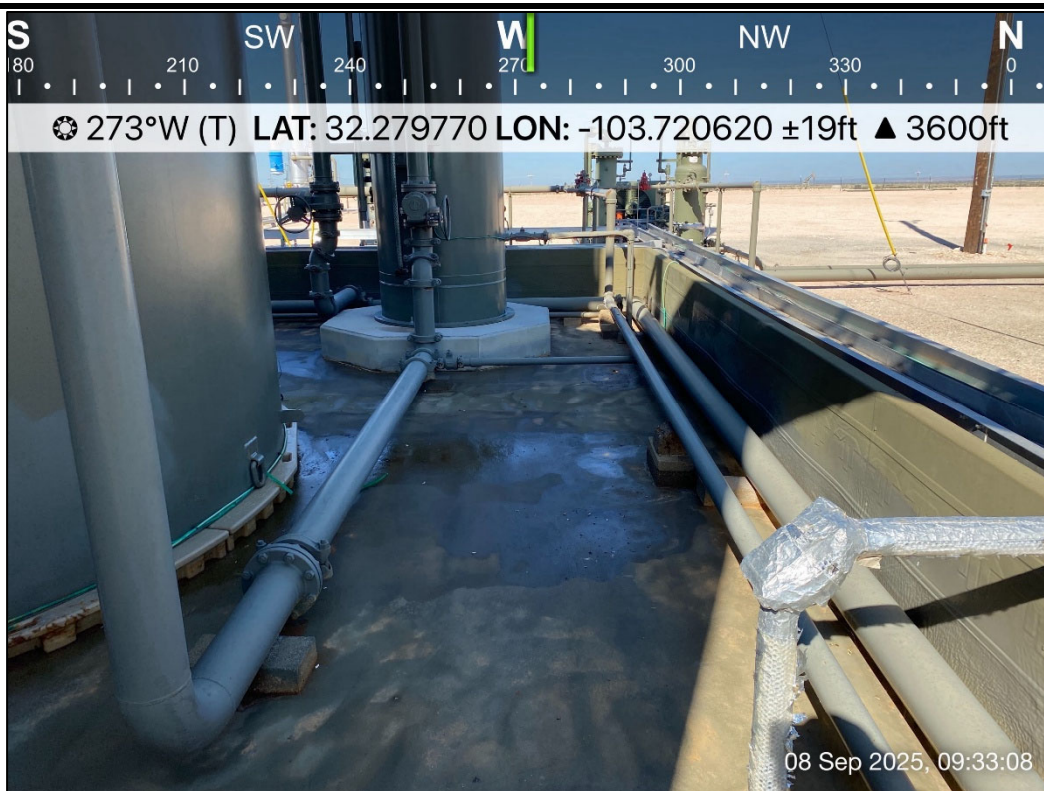
PHOTO 14: Western view during liner inspection activities. 9/8/2025
