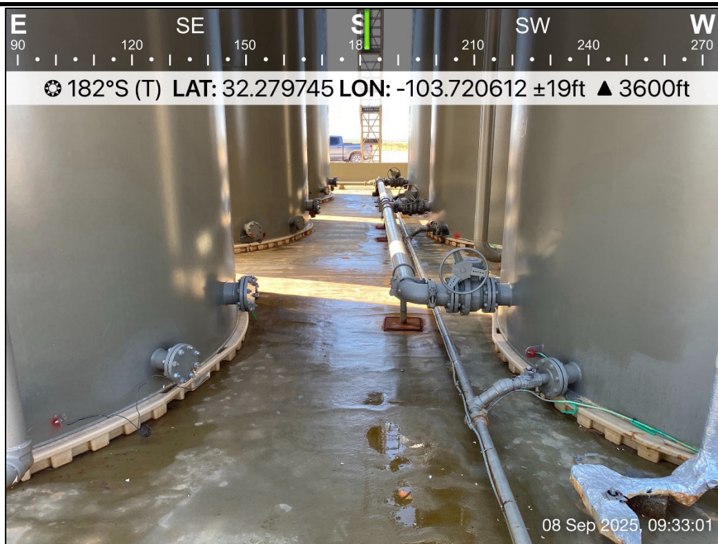
PHOTO 16: Southern view during liner inspection activities. 9/8/2025
