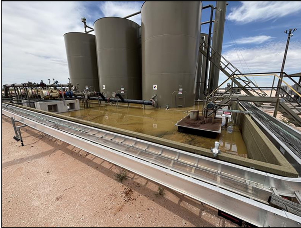
PHOTO 1: Northwestern view during initial site assessment activities. 5/27/2025
