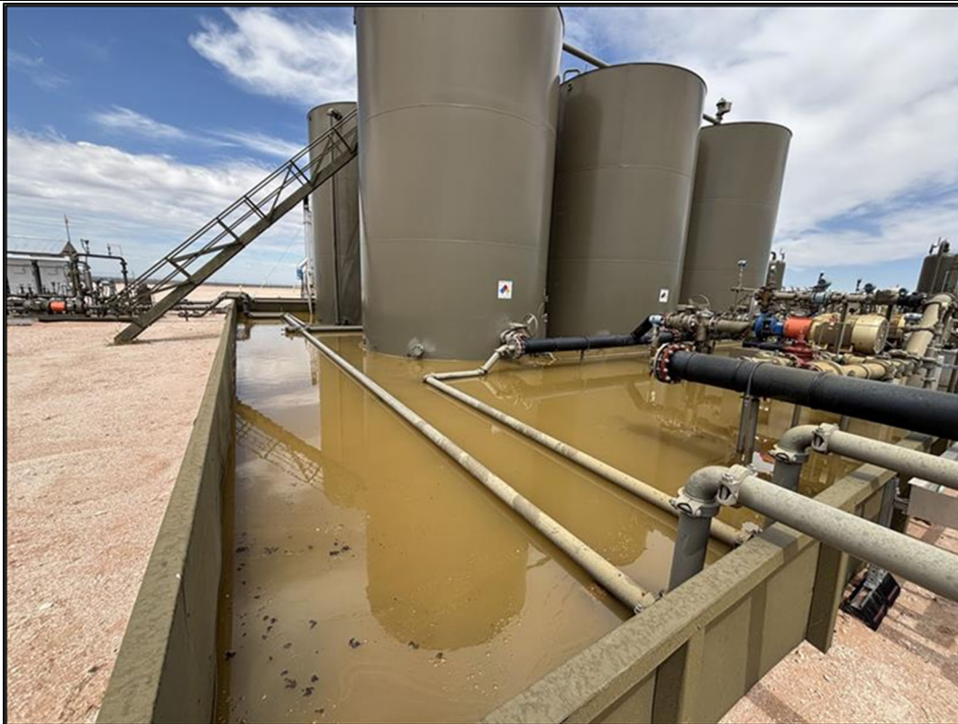
PHOTO 2: Northeastern view during initial site assessment activities. 5/27/2025
