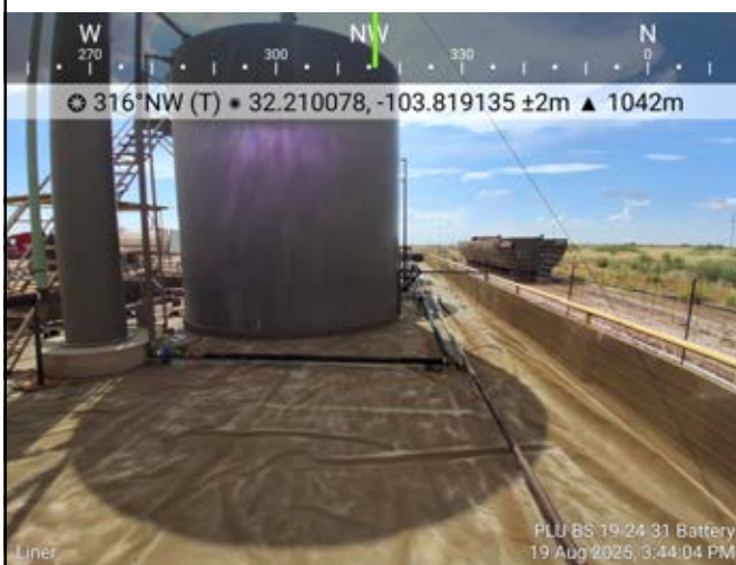
Photograph: 2 Date: 8/19/2025 Description: Liner before cleaning and repairs View: Northwest
