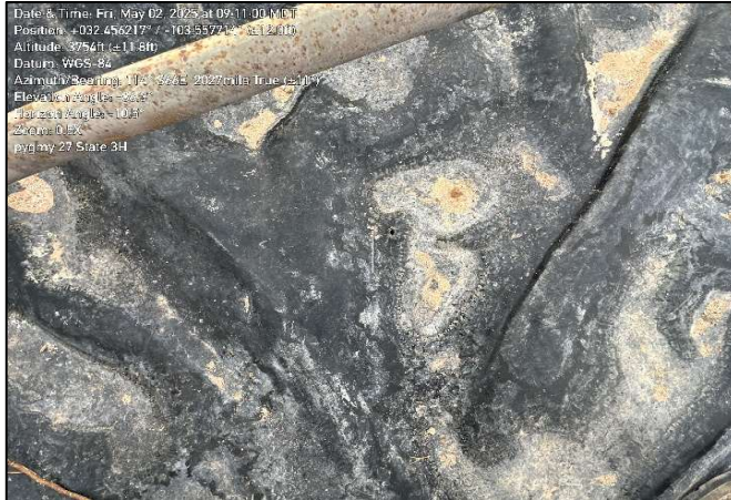
Photograph: 5 Date: 05/02/2025 Description: Compromised liner View: Southeast
