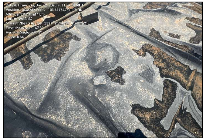
Photograph: 14 Date: 06/12/2025 Description: Patched liner View: Southeast
