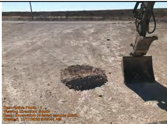
Excavation of failed sample point.
