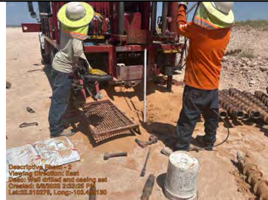
Well drilled and casing set
