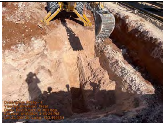
Test trench at 10ft bgs.
