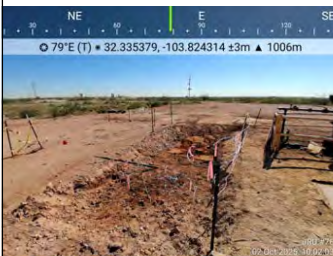
Photograph: 16 Date: 10/2/2025 Description: Excavation activities near FS03 and SW03 View: East
