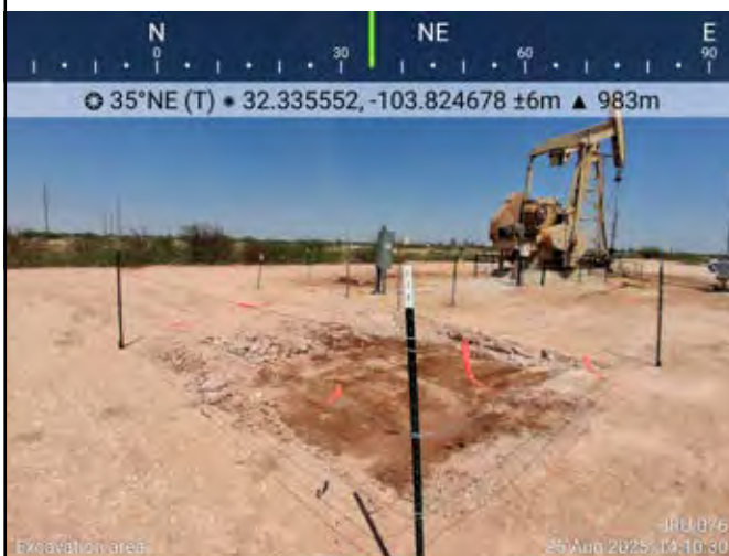
Photograph: 12 Date: 8/25/2025 Description: Excavation activities near FS01 and SW01 View: Northeast
