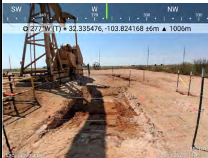
Photograph: 13 Date: 8/25/2025 Description: Excavation activities near FS02 and SW02 View: West
