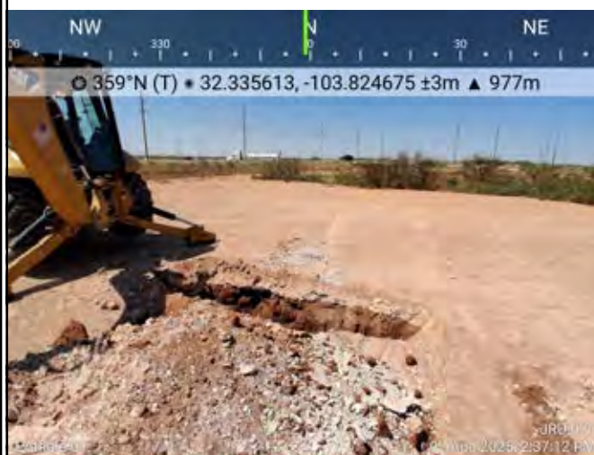
Photograph: 6 Date: 8/7/2025 Description: Additional delineation activities near SS01/PH01 View: North
