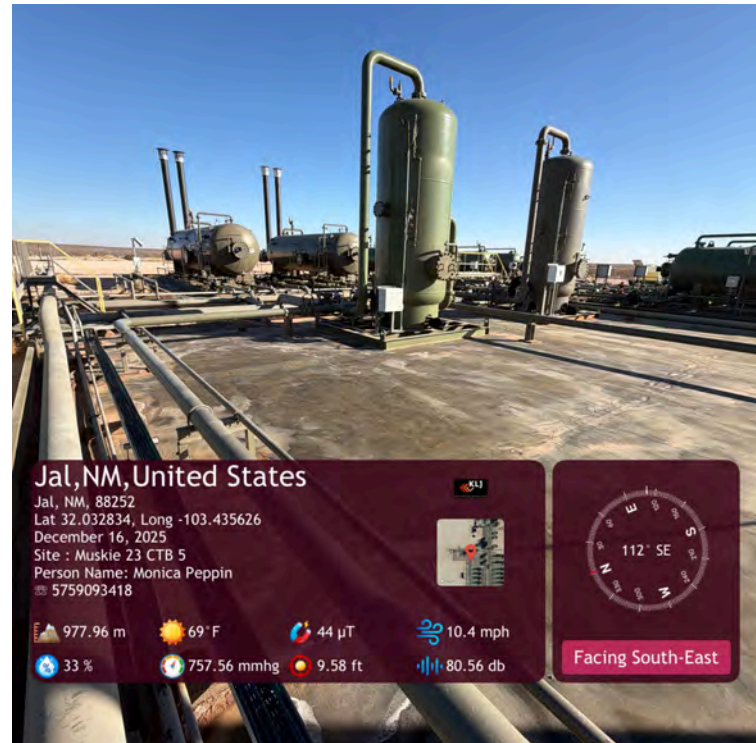
Liner in open area of separator containment.
