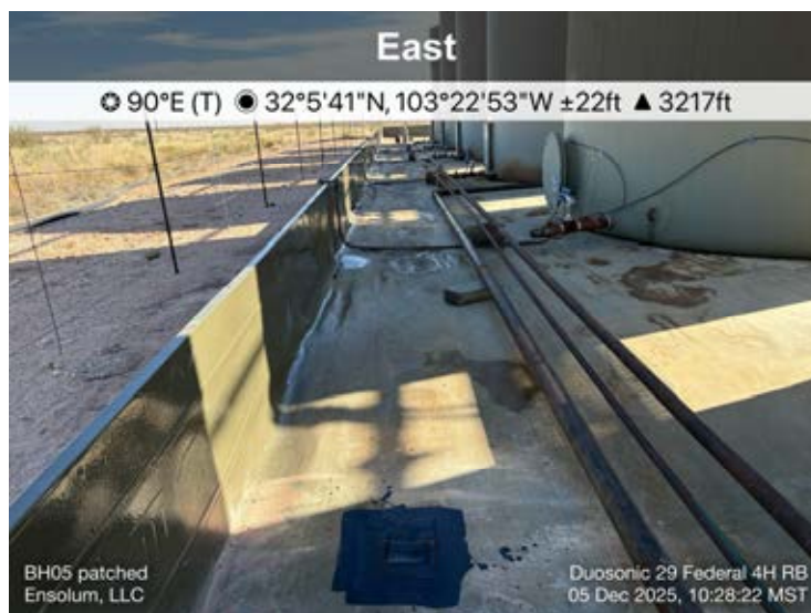
Photograph: 20 Description: Liner patched
