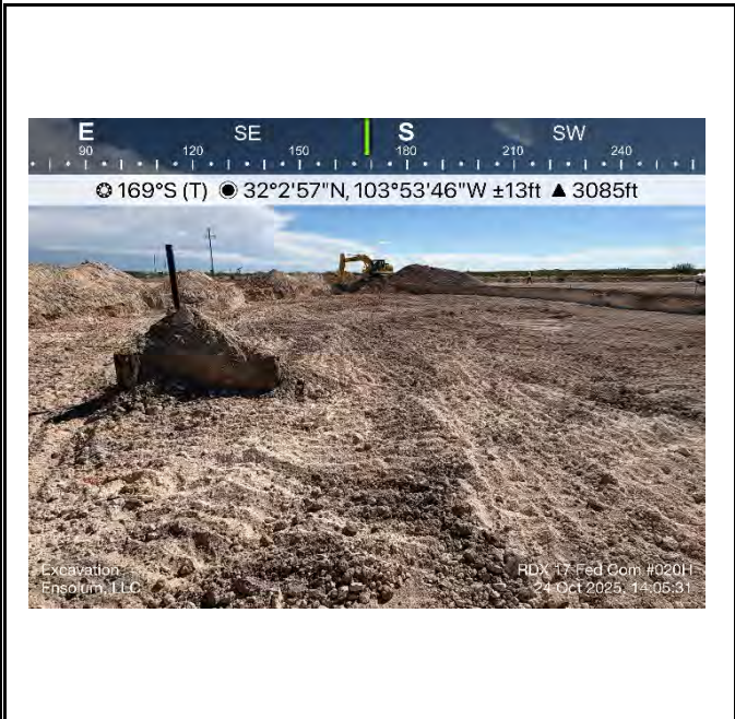
Photograph 19 Date: 10/24/2025 Description: Excavation (nAB1706053151) View: South
