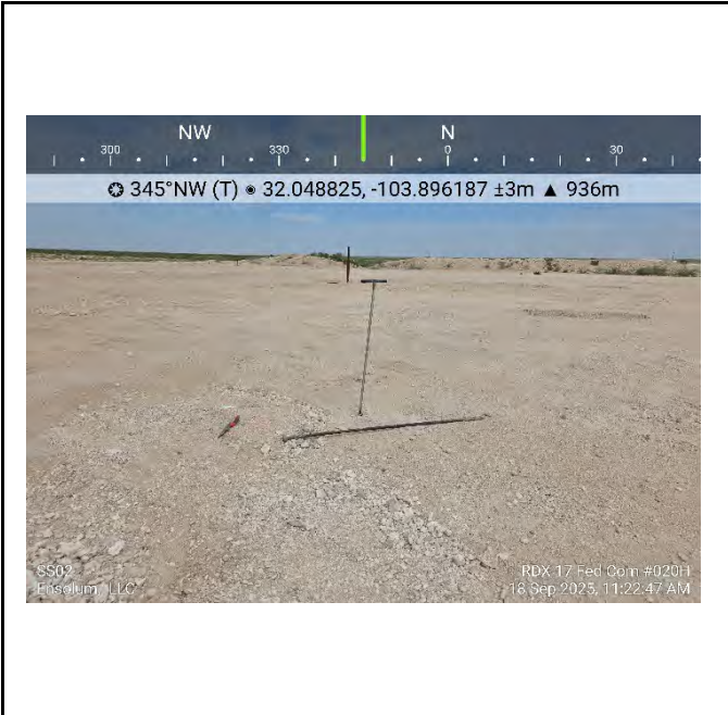
Photograph 6 Date: 9/18/2025 Description: Delineation View: North
