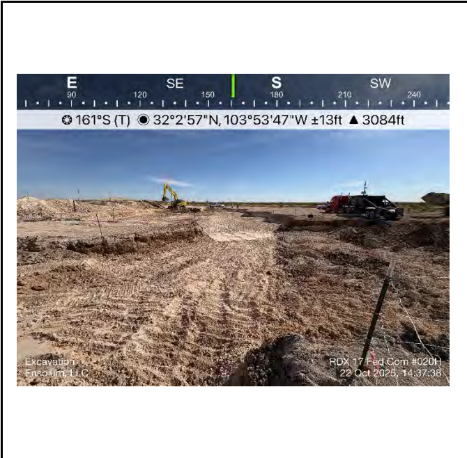
Photograph 14 Date: 10/22/2025 Description: Excavation (nAB1706053151) View: South
