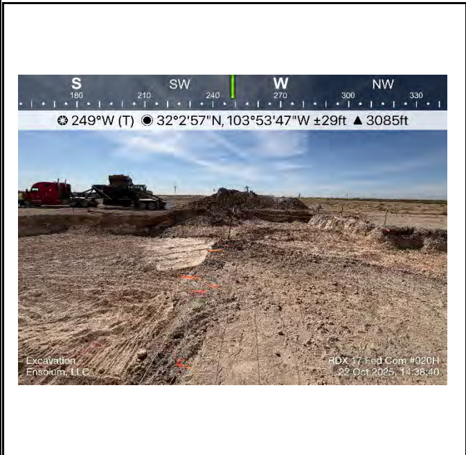
Photograph 15 Date: 10/22/2025 Description: Excavation (nAB1706053151) View: Southwest
