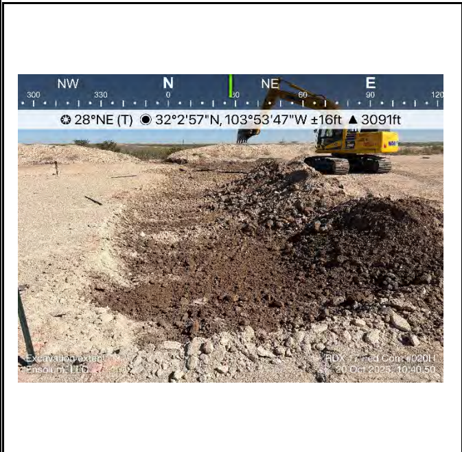
Photograph 7 Date: 10/20/2025 Description: Excavation (nAB1706053151) View: Northeast
