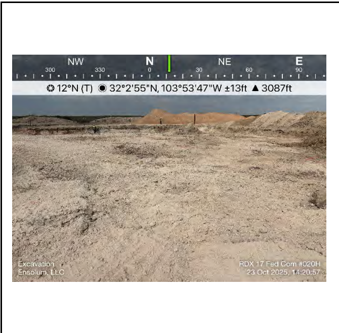
Photograph 16 Date: 10/23/2025 Description: Excavation (nAB1706053151) View: North
