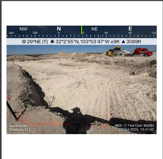
Photograph 13 Date: 10/22/2025 Description: Excavation (nAB1706053151) View: Northeast
