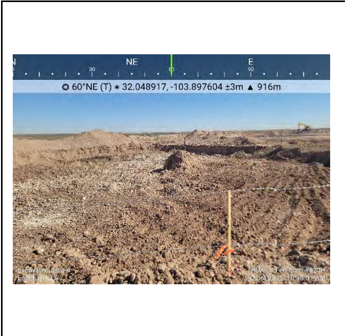
Photograph 26 Date: 10/30/2025 Description: Excavation (nAB1422341439) View: Northeast
