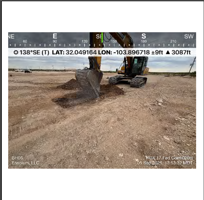
Photograph 5 Date: 9/5/2025 Description: Delineation View: Southeast
