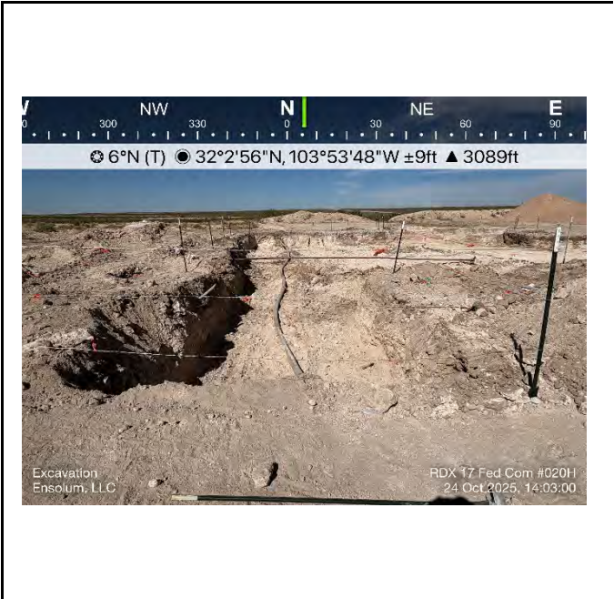
Photograph 18 Date: 10/24/2025 Description: Excavation (nAB1706053151) View: North
