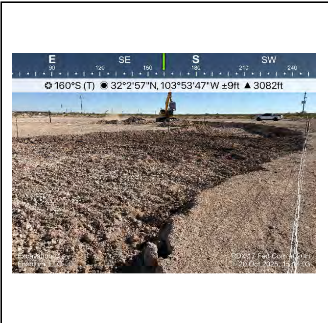
Photograph 8 Date: 10/20/2025 Description: Excavation (nAB1706053151) View: South
