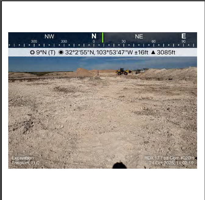
Photograph 17 Date: 10/24/2025 Description: Excavation (nAB1706053151) View: North
