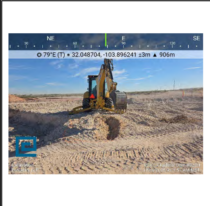
Photograph 27 Date: 11/13/2025 Description: FS97 Excavation (nAB1706053151) View: East
