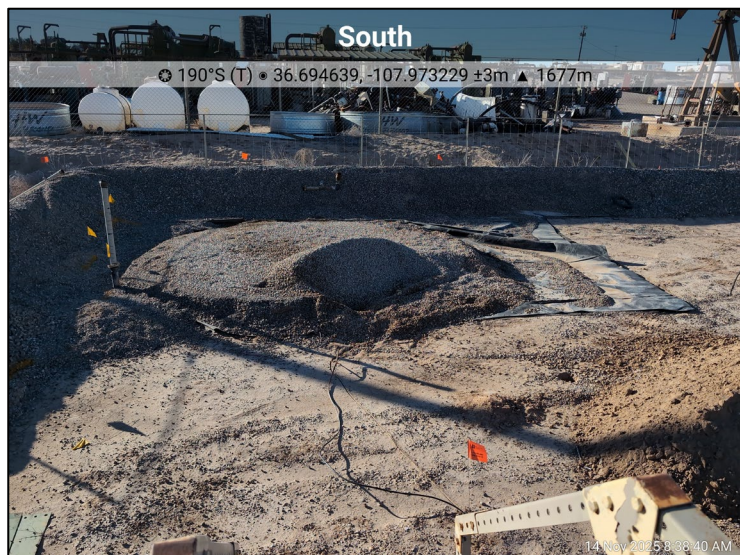
Photograph: 9 Date: 11/14/2025 Description: Release footprint under AST prior to excavation View: South
