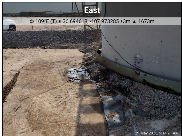
Photograph: 2 Date: 05/29/2025 Description: Release point and soil staining View: East
