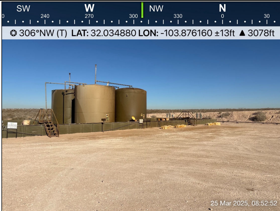
PHOTO 2: Northwestern view during initial site assessment activities. 3/25/2025
