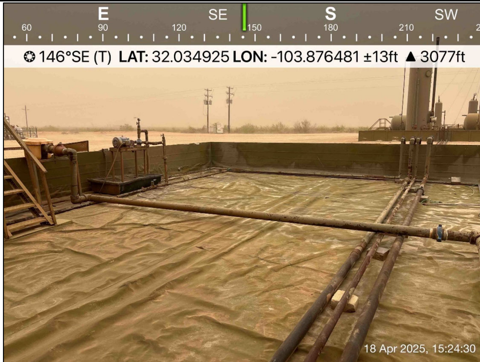
PHOTO 8: Southeastern view during liner inspection activities. 4/18/2025
