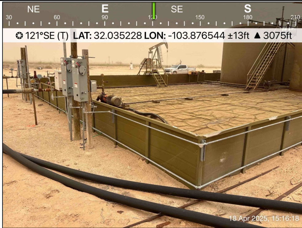
PHOTO 3: Southeastern view outside of the containment during liner inspection activities. 4/18/2025
