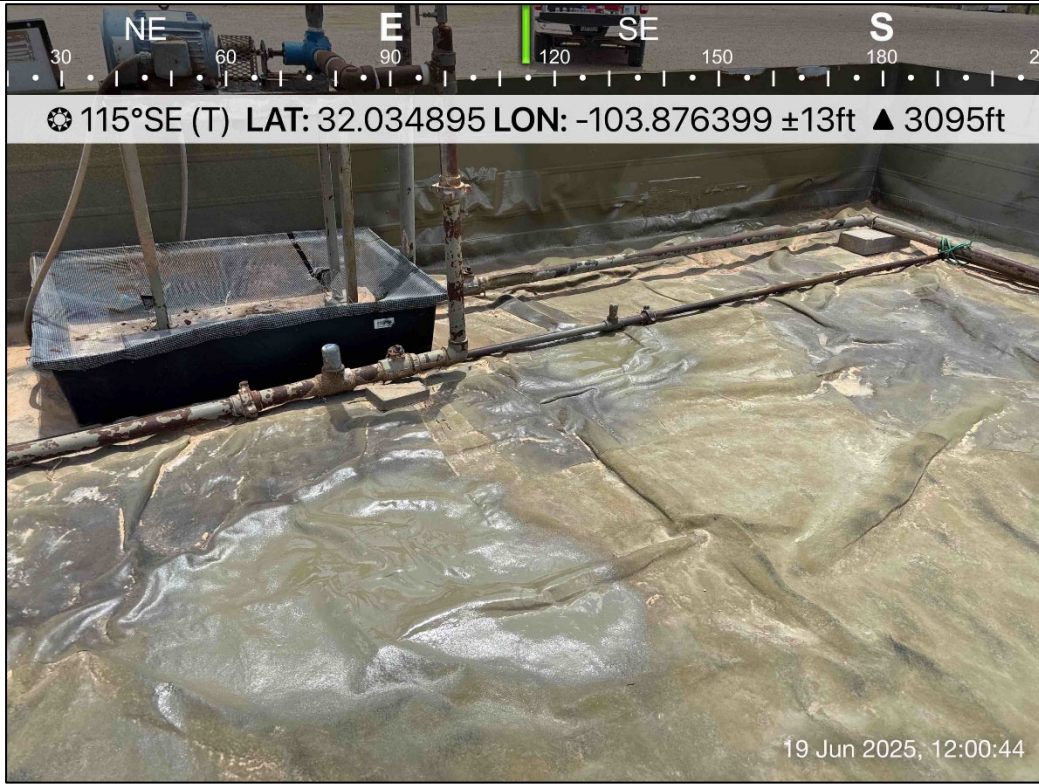
PHOTO 15: Southeastern view following liner repairs. 6/19/2025
