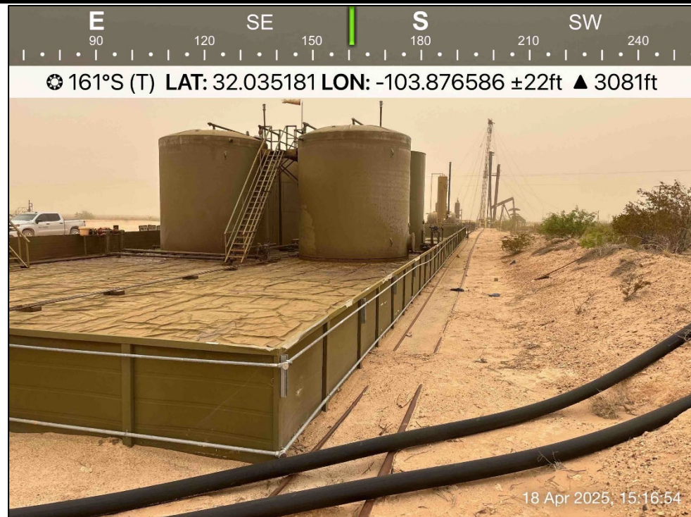
PHOTO 4: Southeastern view outside of the containment during liner inspection activities. 4/18/2025
