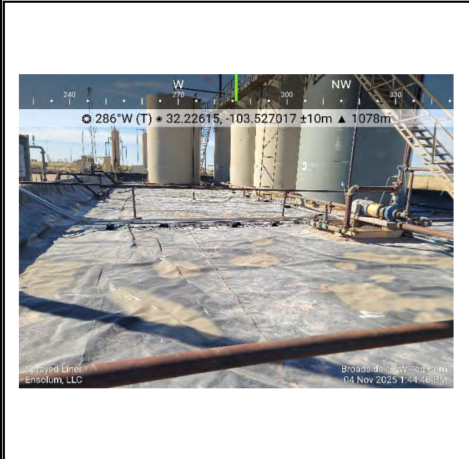
Photograph 39 Date: 11/4/2025 Description: Liner repair (nAPP2524743023) View: West
