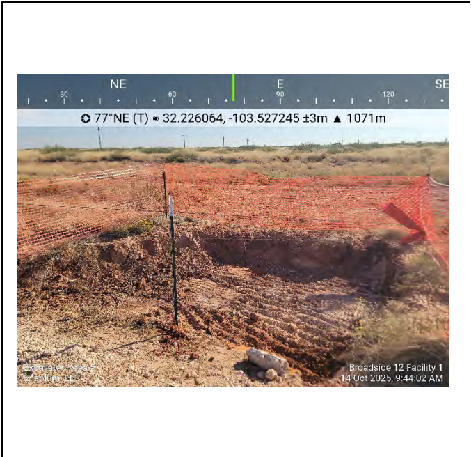
Photograph 24 Date: 10/14/2025 Description: Excavation (nAPP2519539659) View: East
