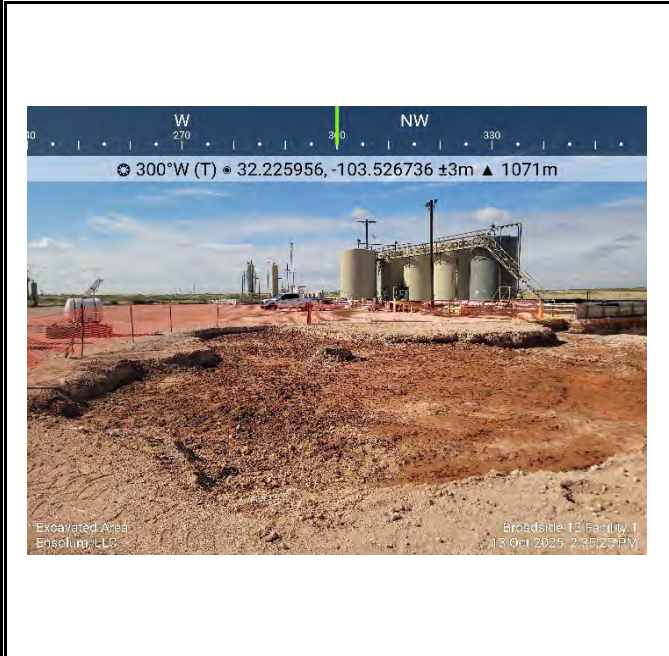
Photograph 23 Date: 10/13/2025 Description: Excavation (nAPP2519539659) View: Northwest
