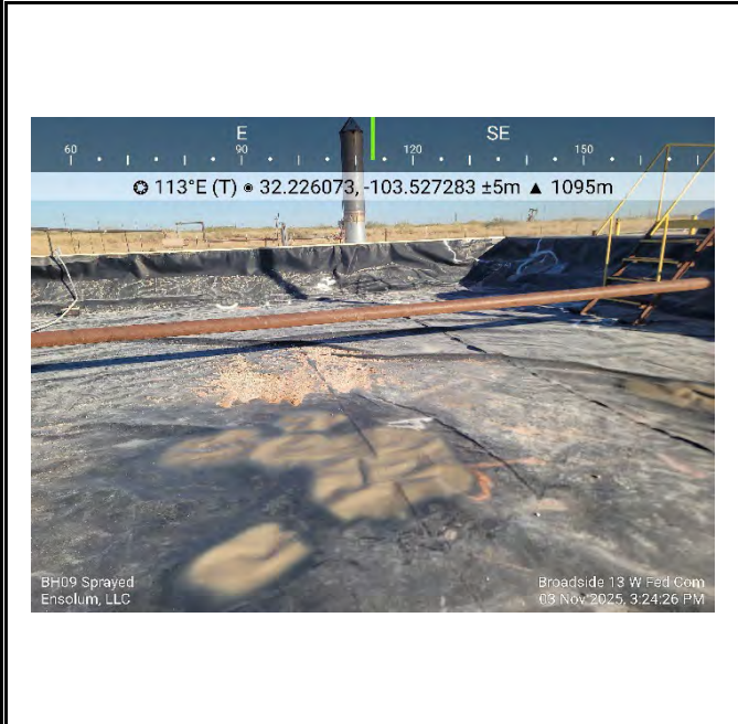
Photograph 37 Date: 11/3/2025 Description: Liner repair (nAPP2524743023) View: Southeast
