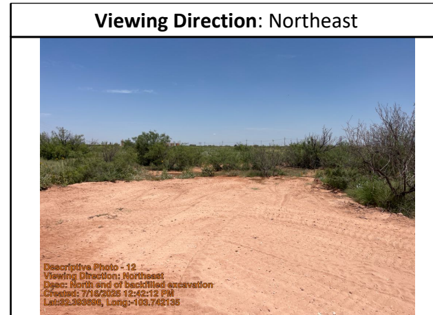
North end of backfilled excavation
