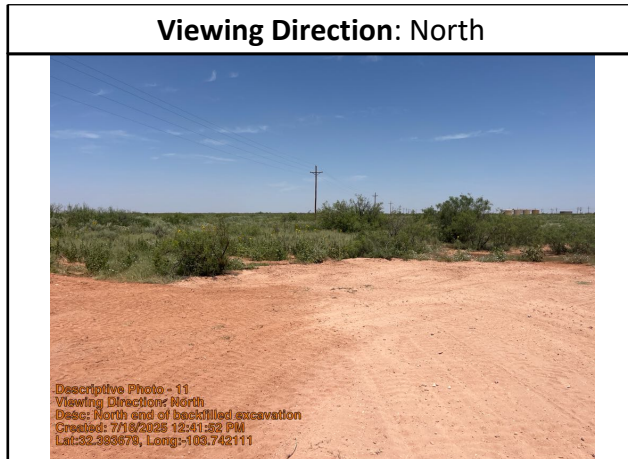
North end of backfilled excavation
