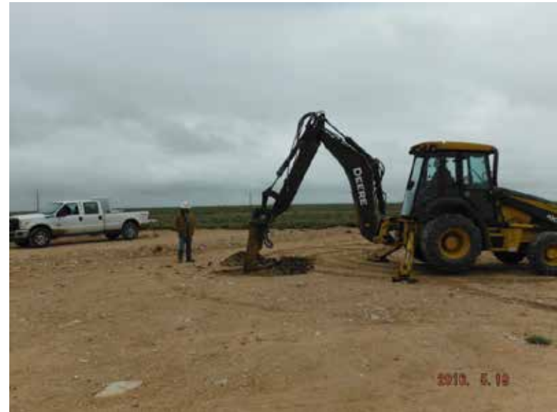
Hammer hoe vertical 1, facing north east
