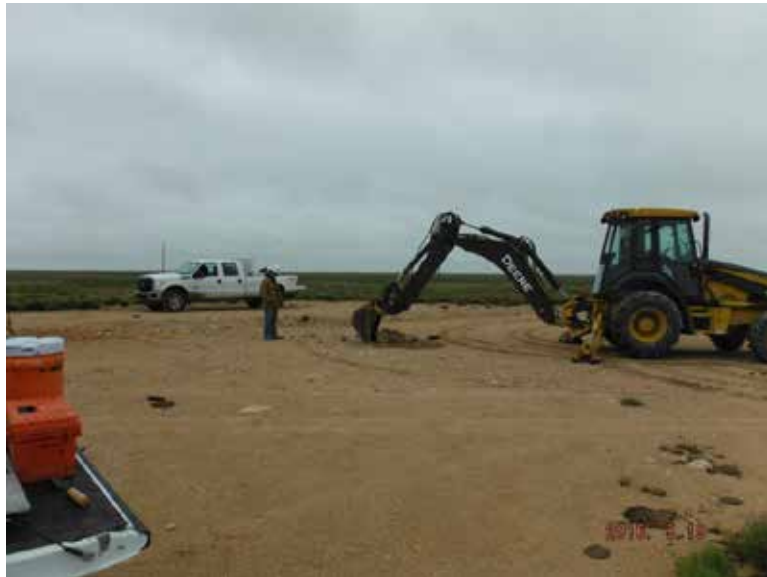
Excavating vertical 1, facing north east
