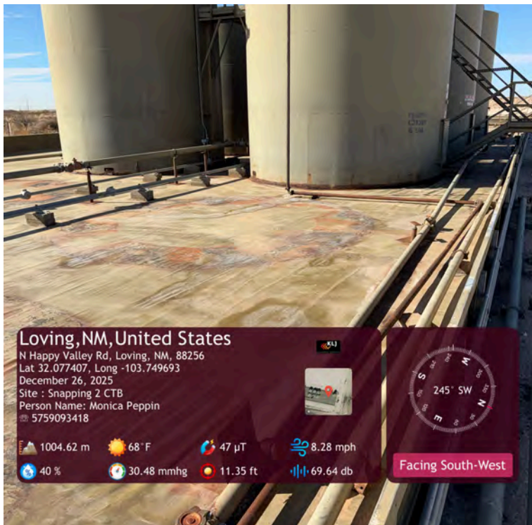
East area of containment.
