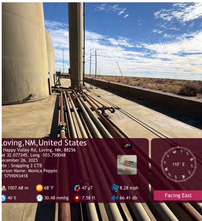
East view from west wall.
