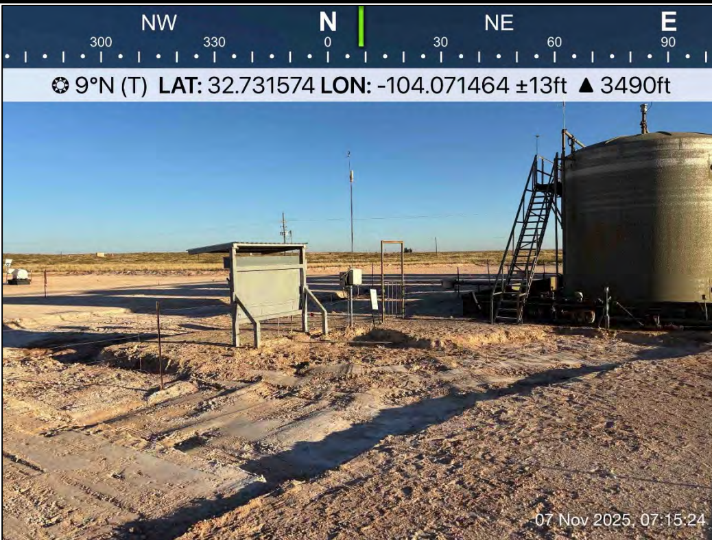
PHOTO 12: Northern view of excavation extent. 11/7/2025
