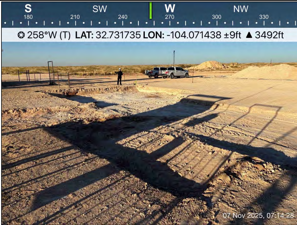
PHOTO 11: Southwestern view of excavation extent. 11/7/2025
