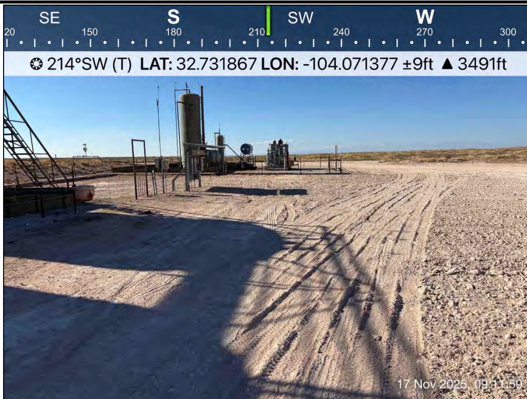
PHOTO 14: Southwestern view following restoration activities. 11/17/2025
