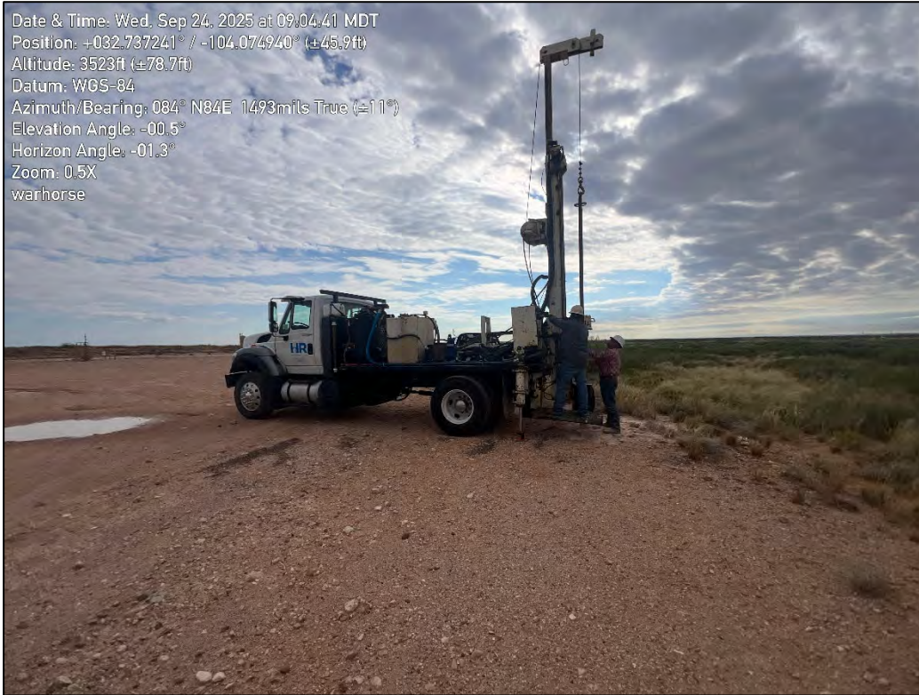
PHOTO 9: Northeastern view during temporary DTW drilling activities. 9/24/2025
