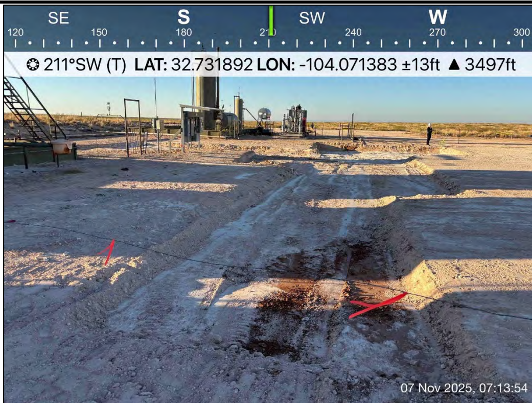
PHOTO 10: Southwestern view of excavation extent. 11/7/2025
