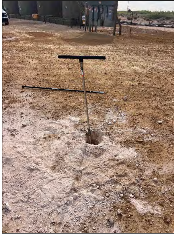
PHOTO 5: Northeastern view of borehole during delineation activities. 5/1/2025
