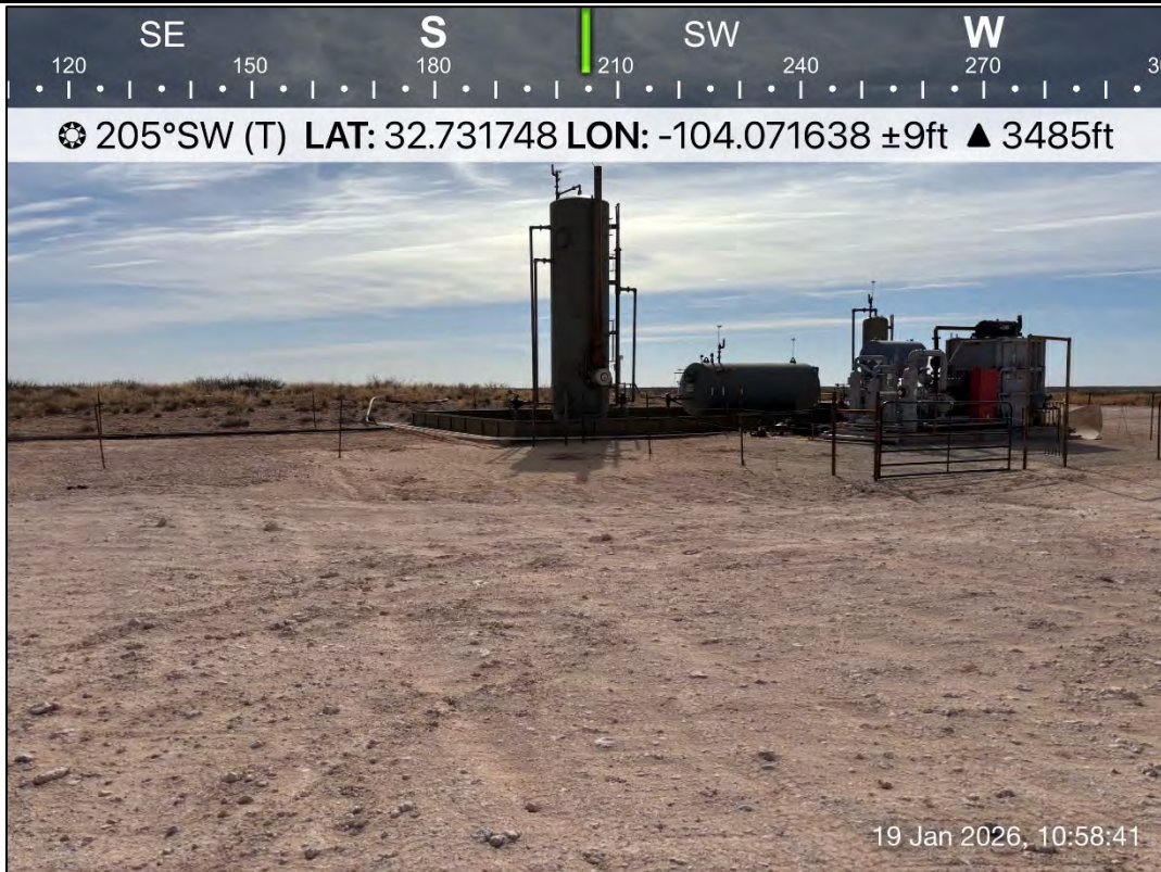
PHOTO 1: Southwestern view during confirmation sampling activities. 1/19/2026
