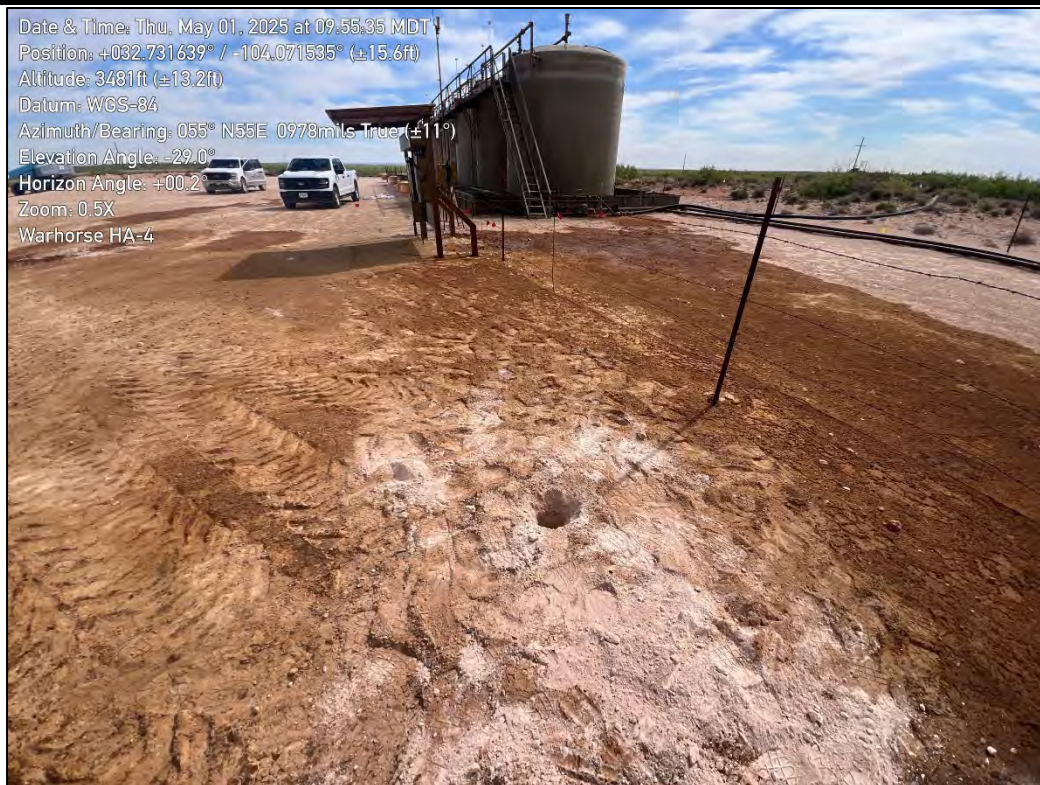
PHOTO 8: Northeastern view of borehole during delineation activities. 5/1/2025
