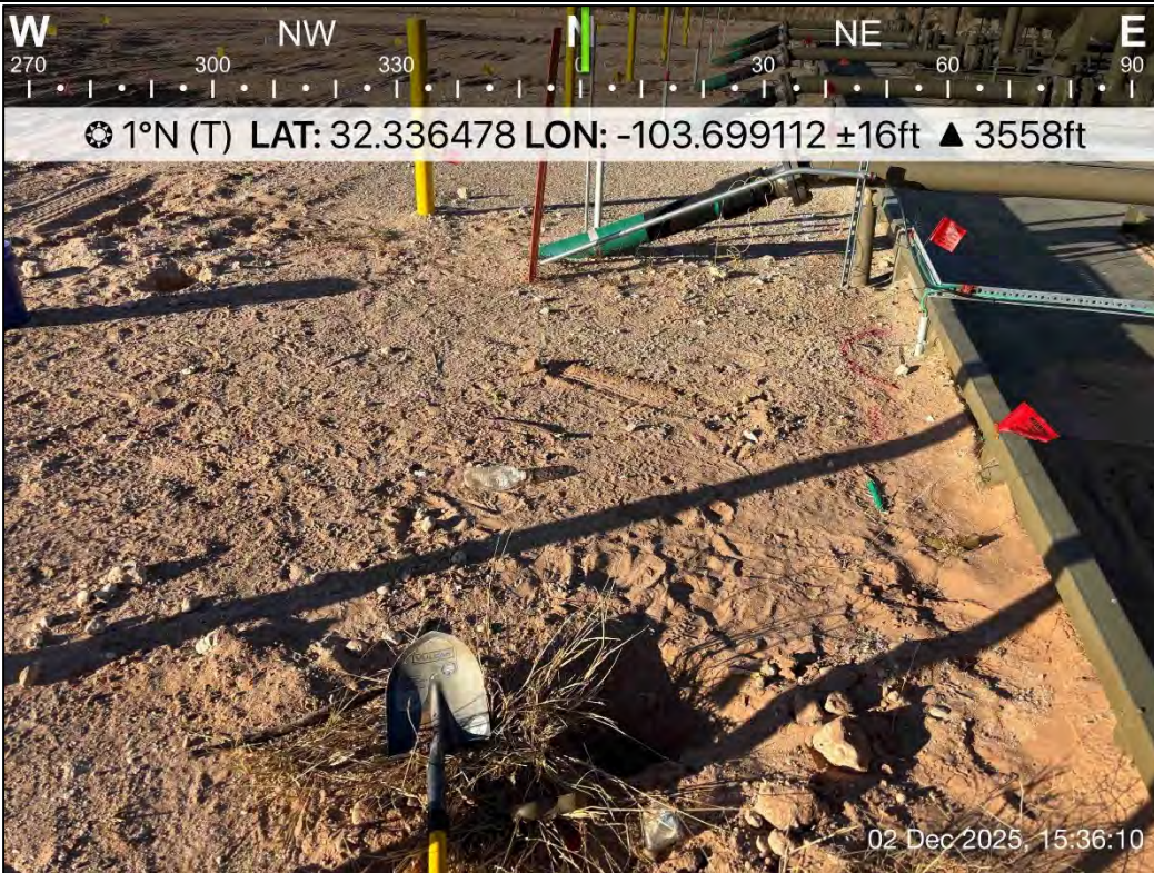
PHOTO 4: Northern view during additional delineation activities. 12/02/2025
