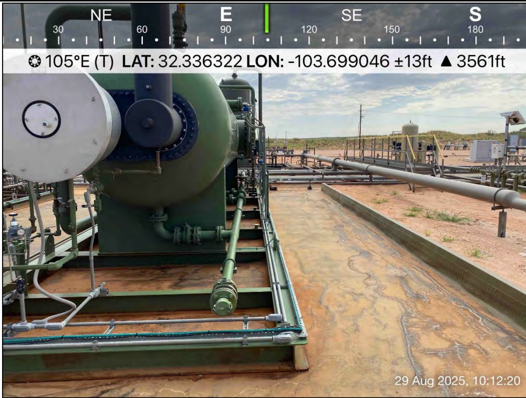
PHOTO 17: Southeastern view during liner inspection activities. 8/29/2025
