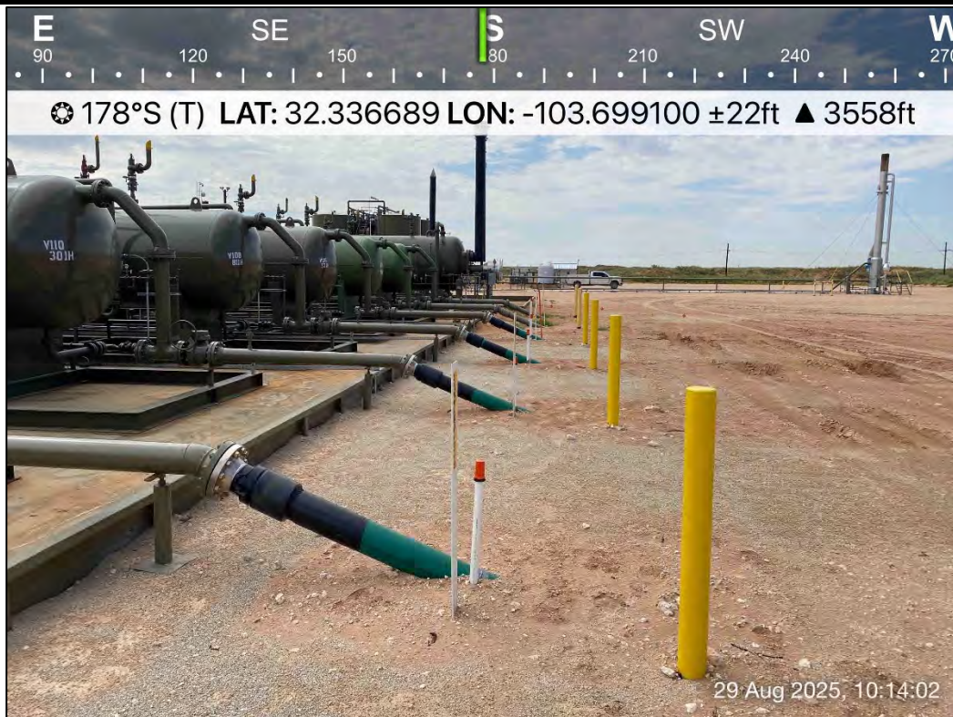
PHOTO 10: Southwestern view outside of containment during liner inspection activities. 8/29/2025
