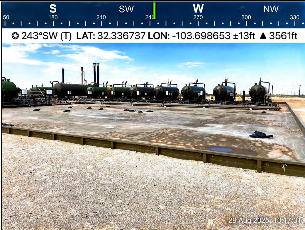
PHOTO 21: Southwestern view of new construction. 8/29/2025
