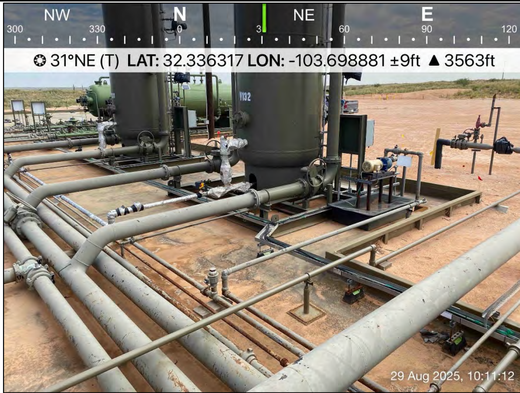
PHOTO 15: Northeastern view during liner inspection activities. 8/29/2025
