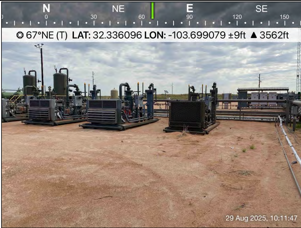
PHOTO 7: Northeastern view outside of containment during liner inspection activities. 8/29/2025
