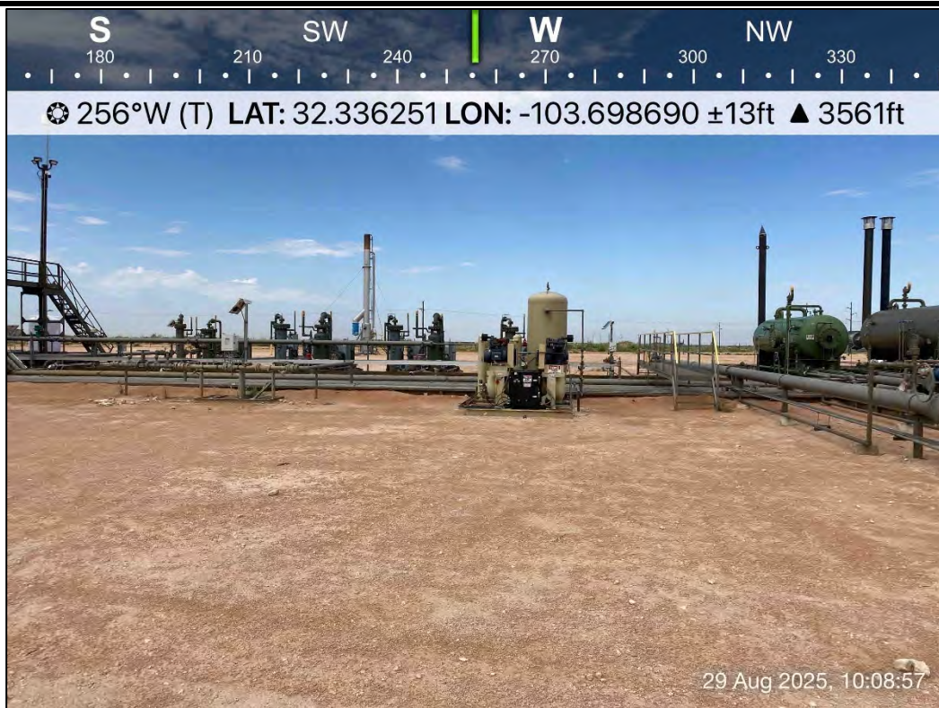
PHOTO 6: Southwestern view outside of containment during liner inspection activities. 8/29/2025
