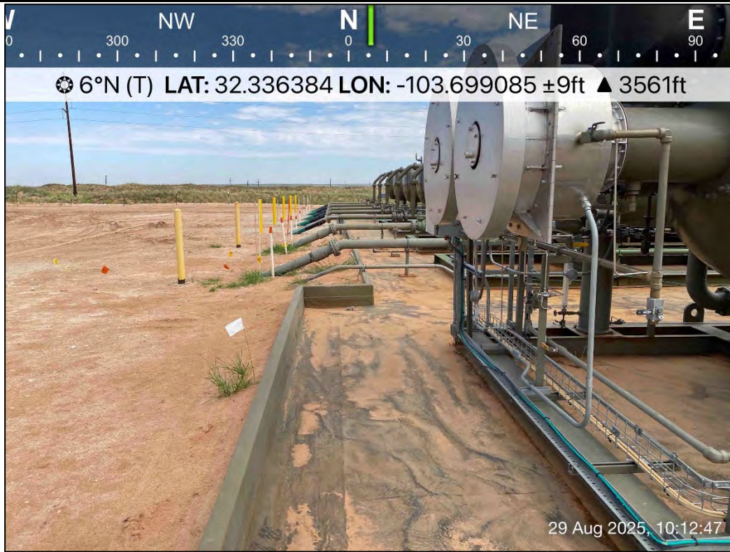
PHOTO 13: Northeastern view during liner inspection activities. 8/29/2025
