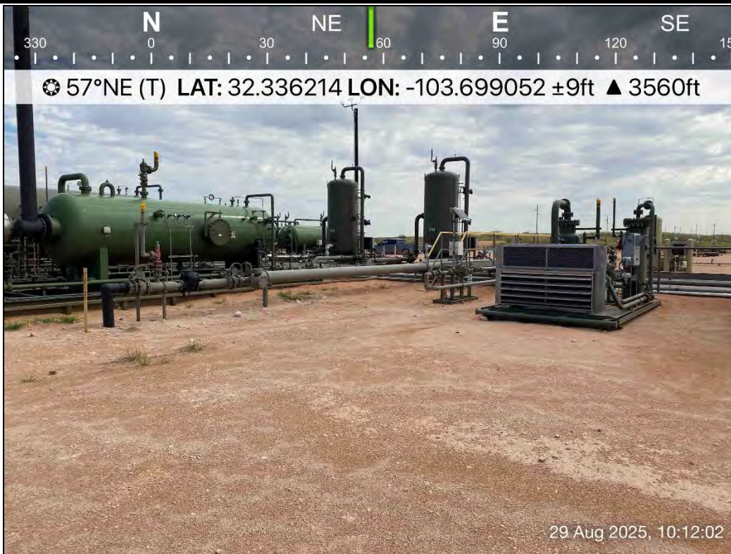
PHOTO 8: Northeastern view outside of containment during liner inspection activities. 8/29/2025
