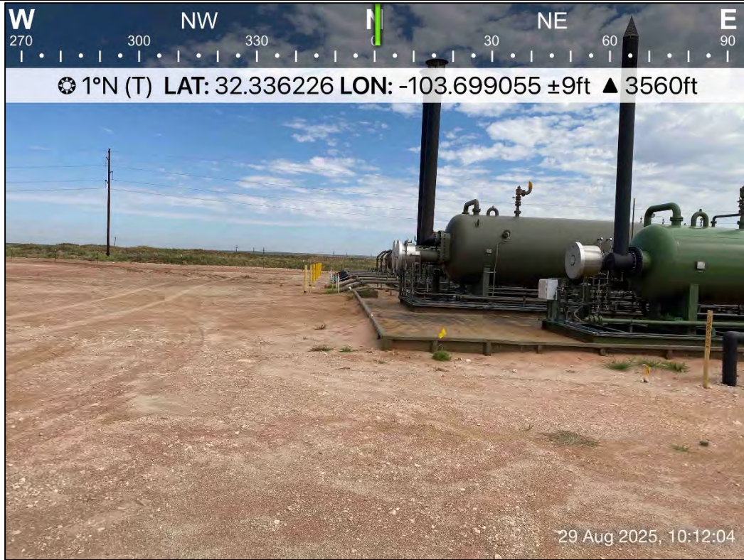
PHOTO 9: Northern view outside of containment during liner inspection activities. 8/29/2025
