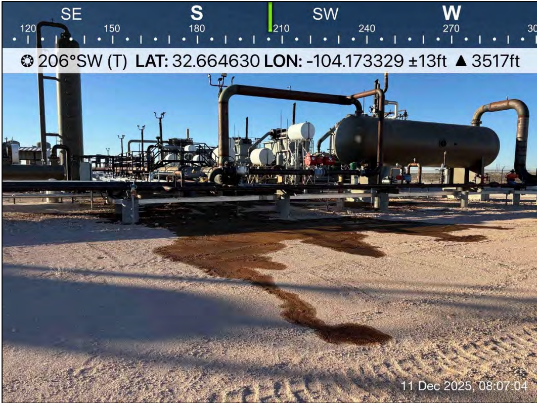
PHOTO 2: Southwestern view during initial site assessment activities. 12/11/2025
