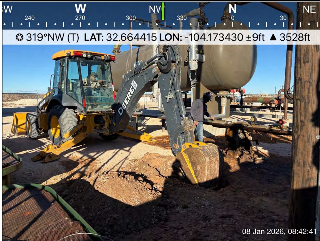
PHOTO 6: Northwestern view during additional delineation activities. 1/08/2026
