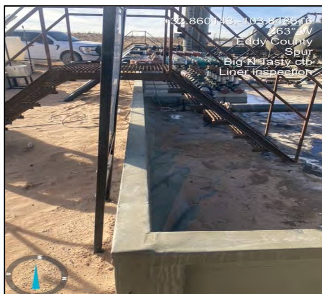
Photo of liner taken prior to power washing facing West.
