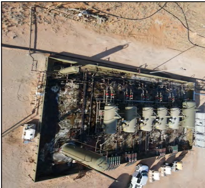
Aerial photos prior to powerwash.
