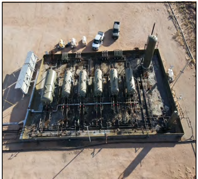
Aerial photos prior to powerwash.
