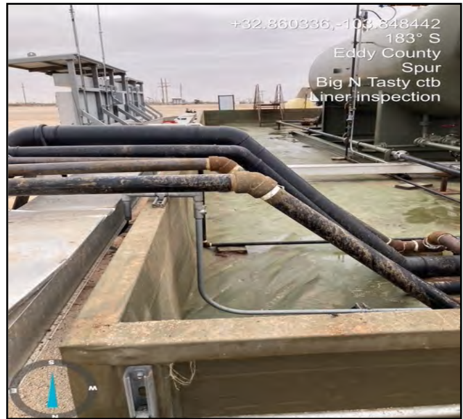
Photo taken pursuant to power washing facing South.
