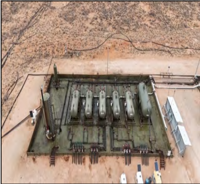
Aerial photo of location post power wash.
