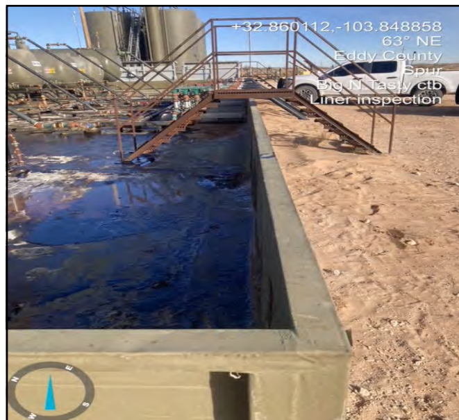
Photo of liner taken prior to power washing facing Northeast.
