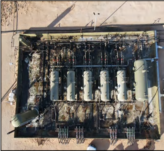
Aerial photos prior to powerwash.
