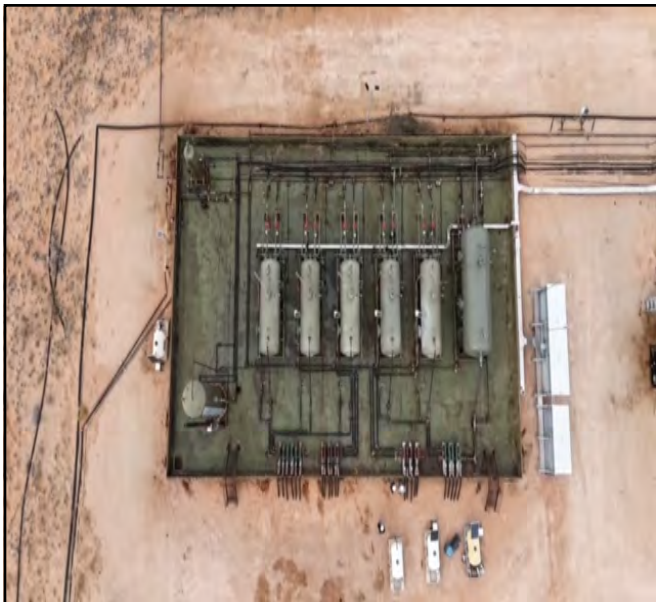
Aerial photo of location post power wash.
