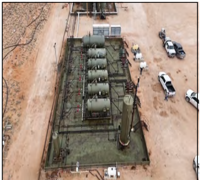
Aerial photo of location post power wash.
