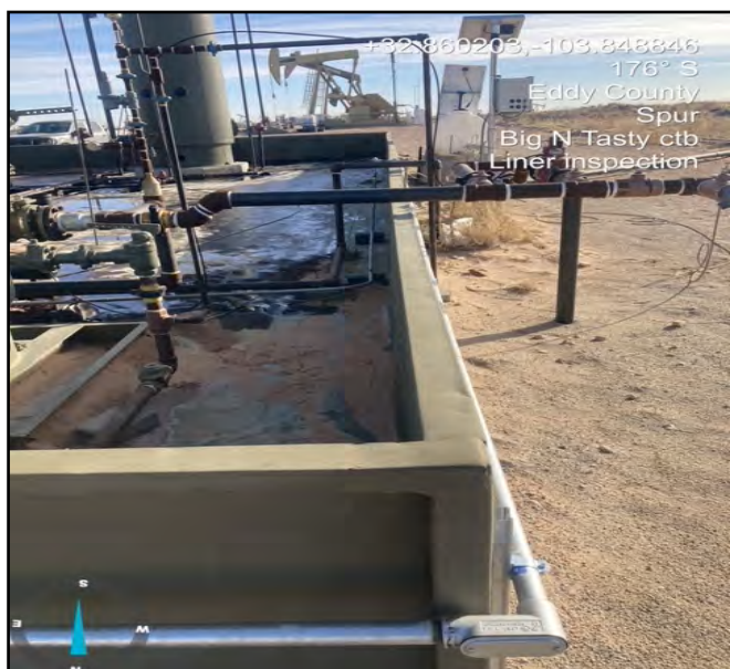
Photo of liner taken prior to power washing facing South.
