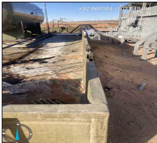
Photo of liner taken prior to power washing facing North.
