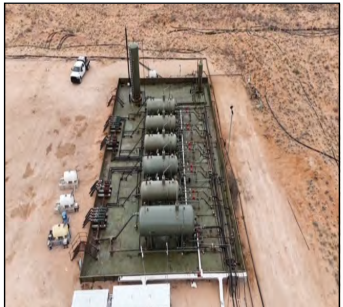
Aerial photo of location post power wash.
