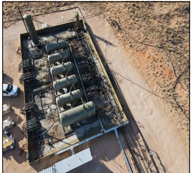
Aerial photos prior to powerwash.
