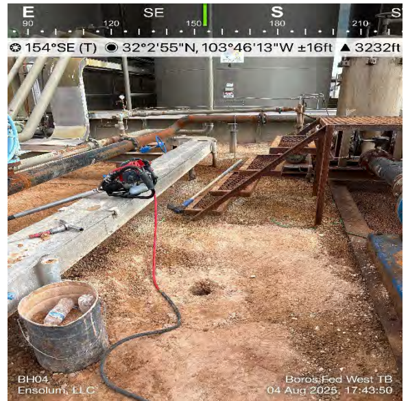
Photograph 8 Date: 8/4/2025 Description: BH04 View: Southeast
