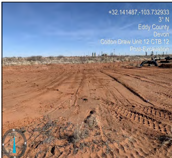
Photo taken post excavation facing north.
