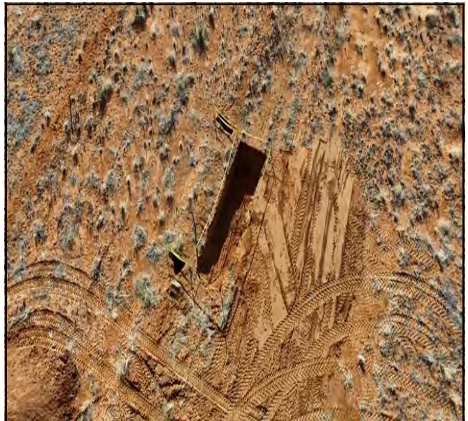
Aerial photo taken during the excavation process.
