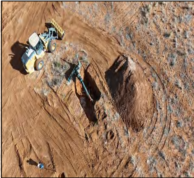
Aerial photo taken during the excavation process.
