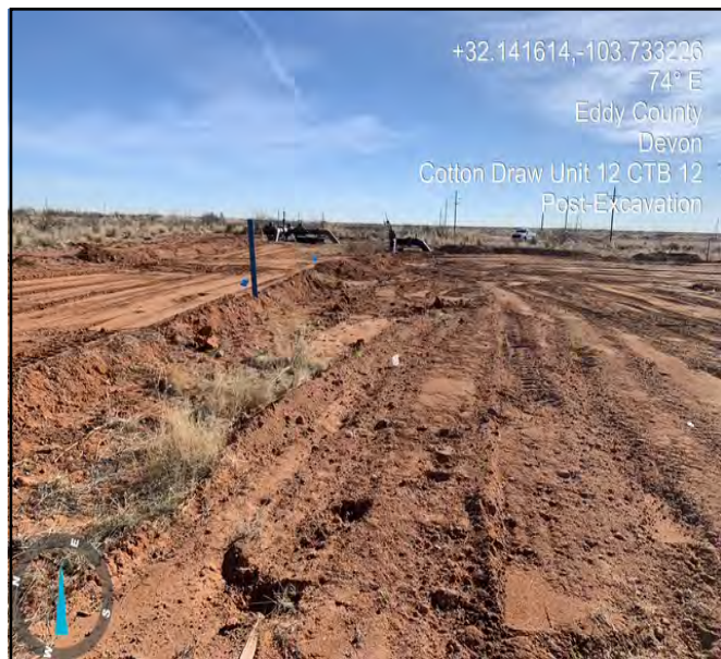
Photo taken post excavation facing east.
