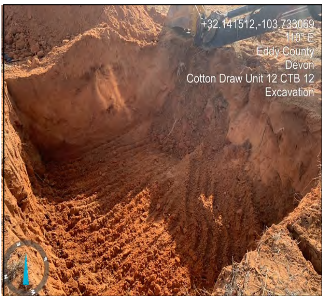
Photo taken during the excavation process facing east.
