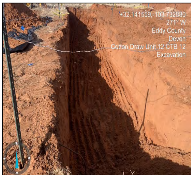
Photo taken during the excavation process facing west.
