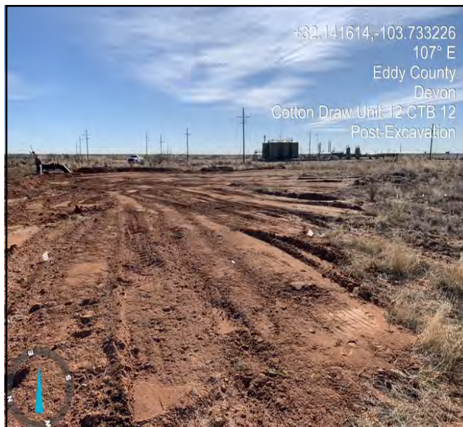
Photo taken post excavation facing east.
