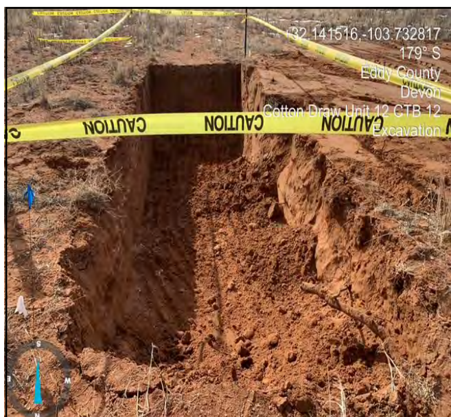
Photo taken during the excavation process facing south.
