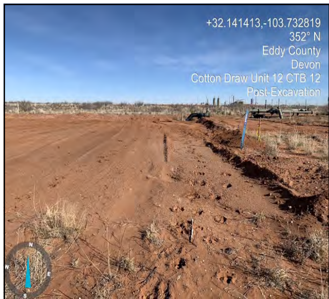
Photo taken post excavation facing north.
