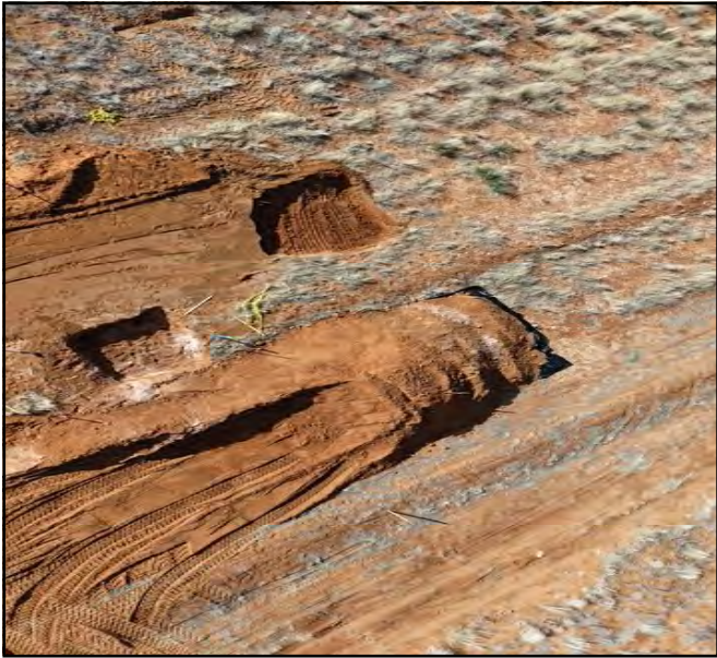
Aerial photo taken during the excavation process.
