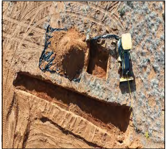
Aerial photo taken during the excavation process.
