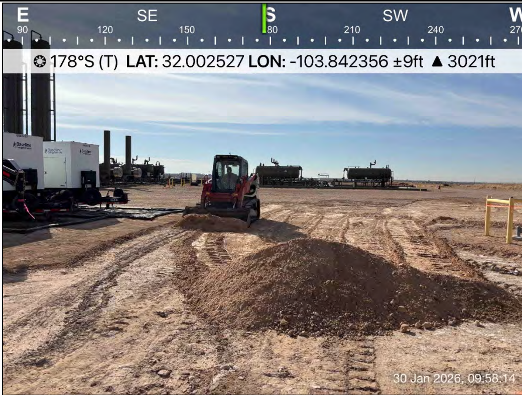
PHOTO 11: Southern view during excavation activities. 1/30/2026
