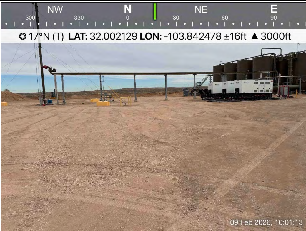
PHOTO 16: Northeastern view following restoration activities. 2/09/2026
