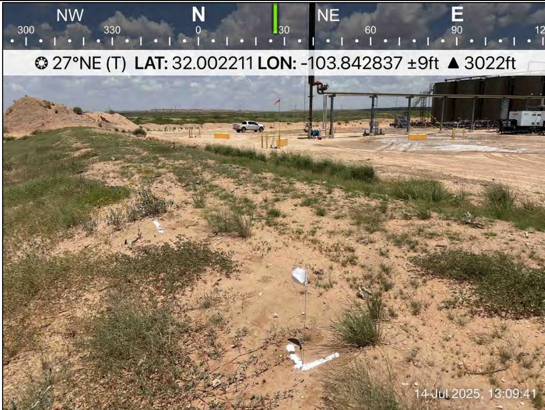
PHOTO 2: Northeastern view during initial site assessment activities. 7/14/2025
