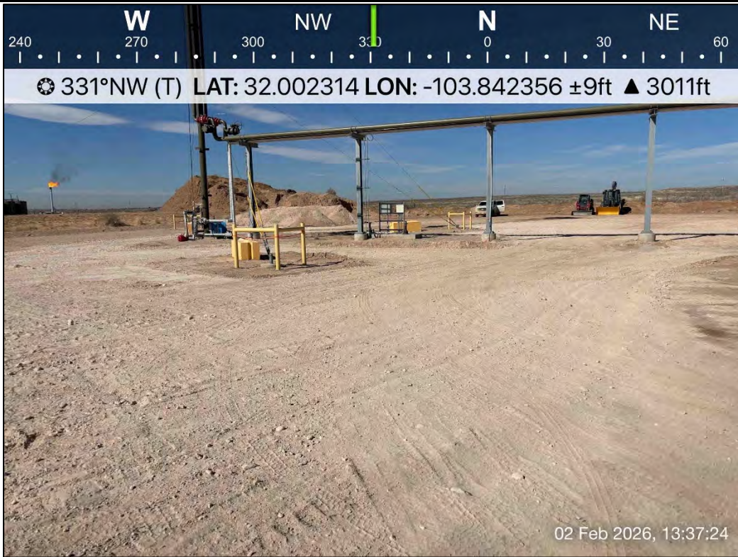
PHOTO 13: Northwestern view of excavation extent. 2/02/2026
