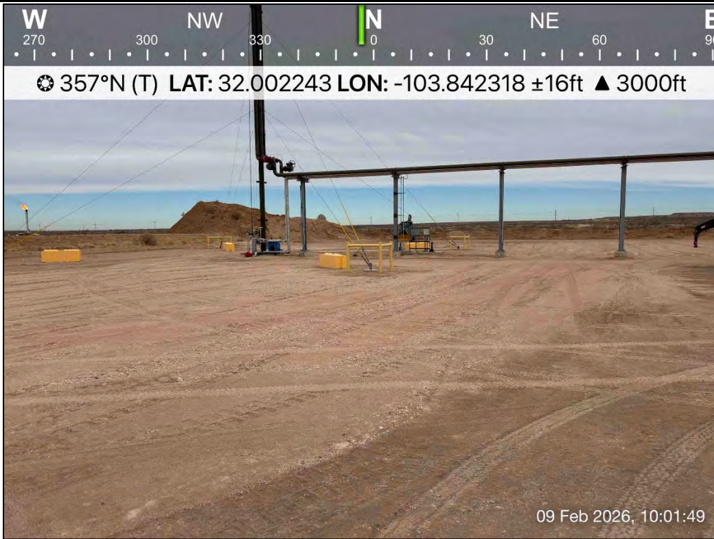
PHOTO 17: Northern view following restoration activities. 2/09/2026
