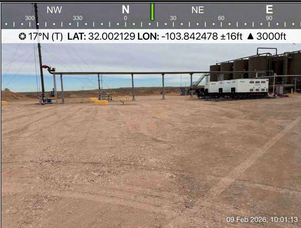
PHOTO 16: Northeastern view following restoration activities. 2/09/2026
