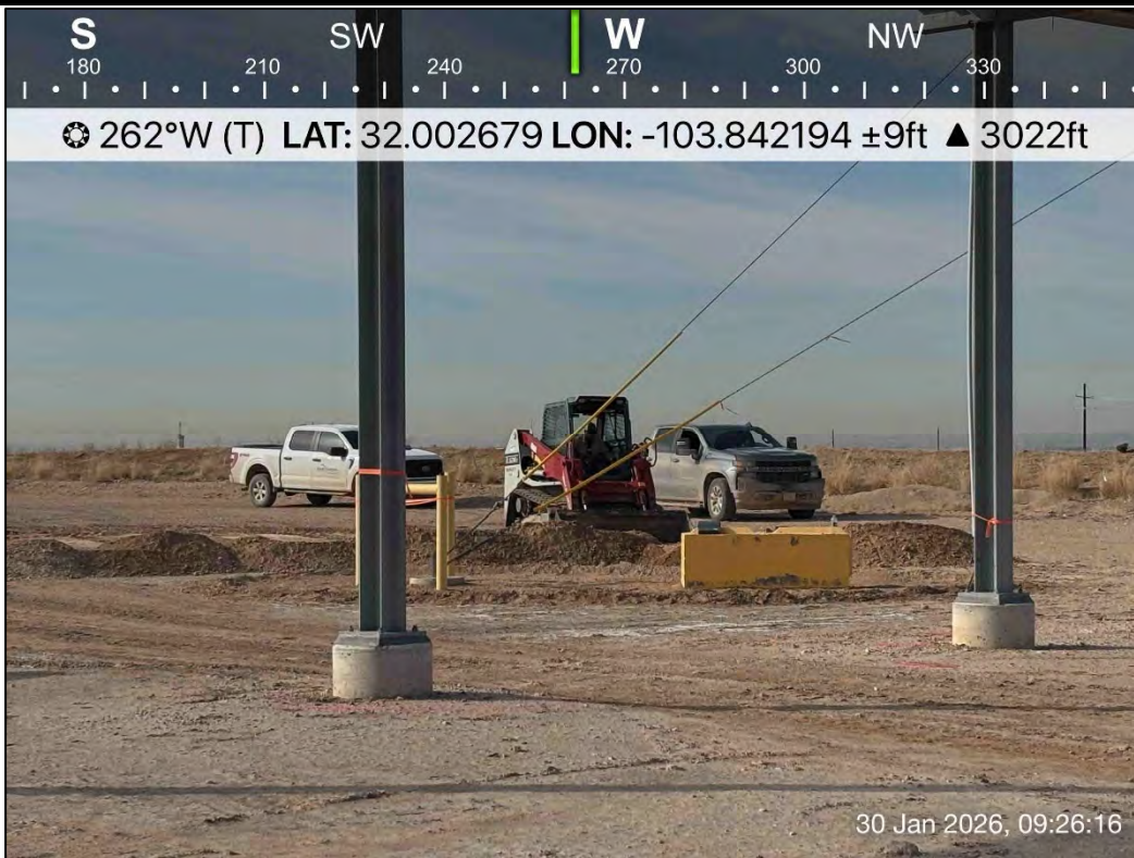
PHOTO 10: Southwestern view during excavation activities. 1/30/2026
