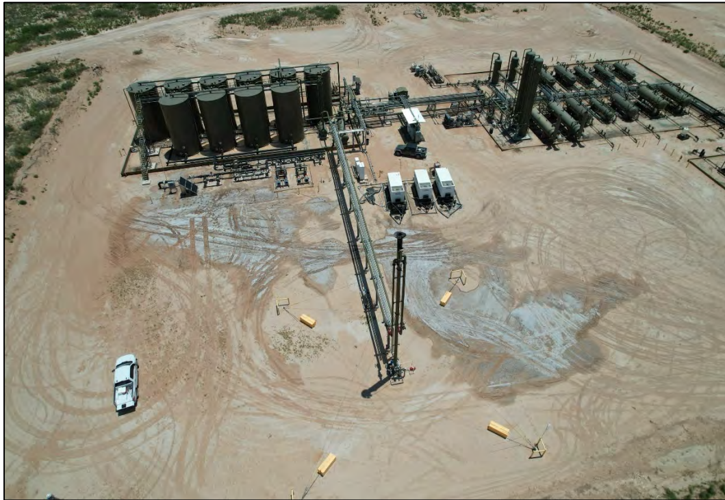
PHOTO 1: Eastern aerial view during initial site assessment activities. 7/14/2025
