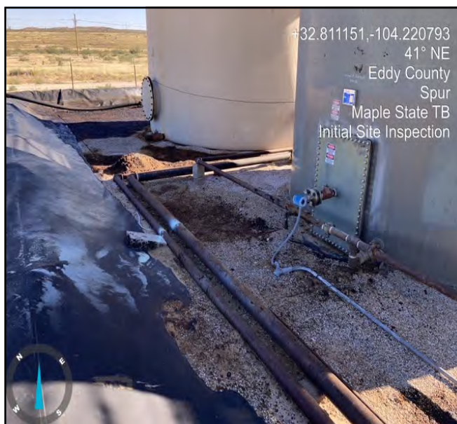
Photo of liner taken during initial liner inspection facing northeast.
