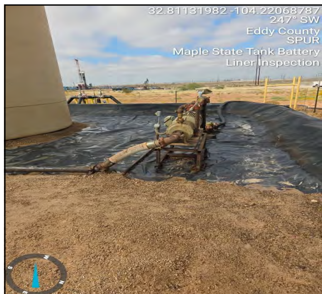
Photo taken pursuant to power washing. Facing southwest.
