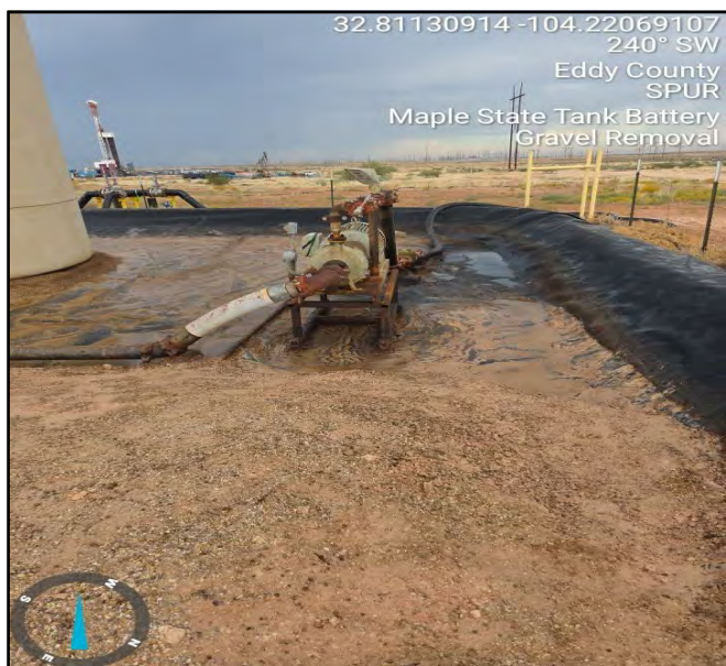
Photograph taken prior to gravel removal, facing southwest.
