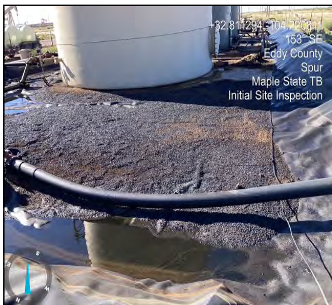
Photo of liner taken during initial liner inspection facing southeast.
