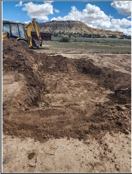
Photo 1 Initial Excavation. Looking east, buried pipe is exposed during the excavation.
