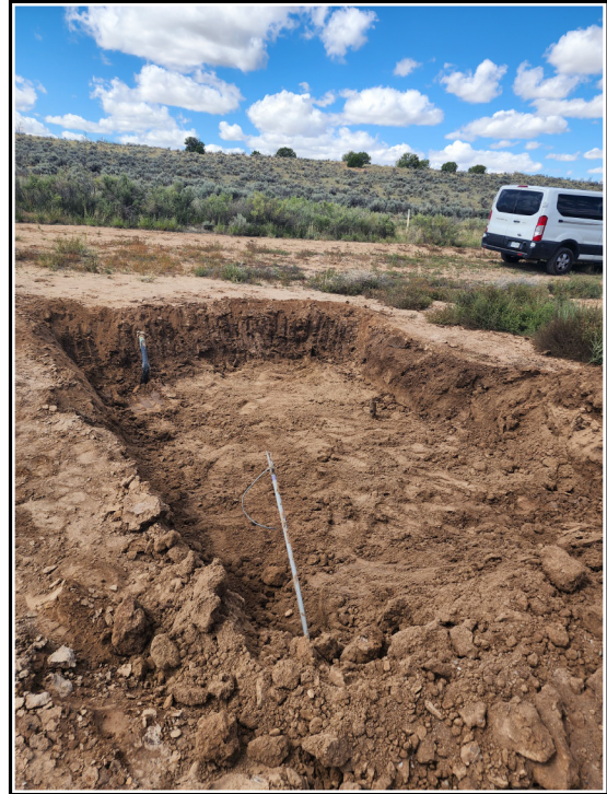
Photo 2 Initial Excavation. Looking west, buried pipe is exposed during the excavation.
