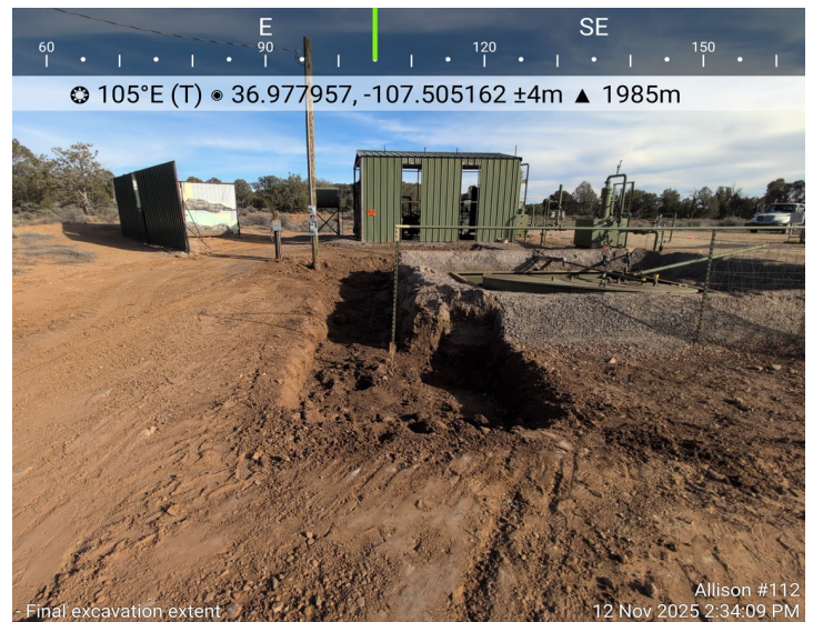
Photograph: 16 Description: Final Excavation Extent
