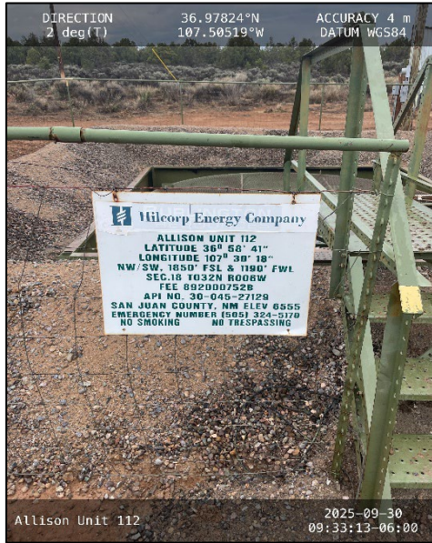
Photograph: 1 Description: API informational sign. View: North Date: 09/30/2025
