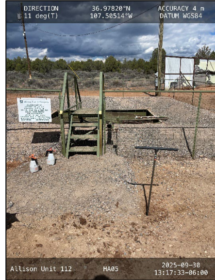
Photograph: 6 Date: 09/30/2025 Description: HA05, South of BGT. View: West
