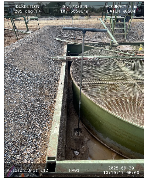
Photograph: 10 Date: 09/30/2025 Description: HA01, advanced within the BGT pit.. View: South
