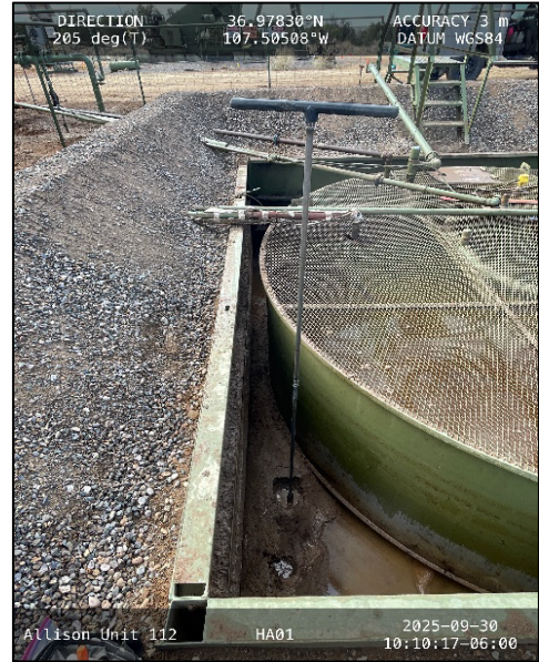
Photograph: 2 Description: HA01, advanced within the BGT pit. View: South Date: 09/30/2025
