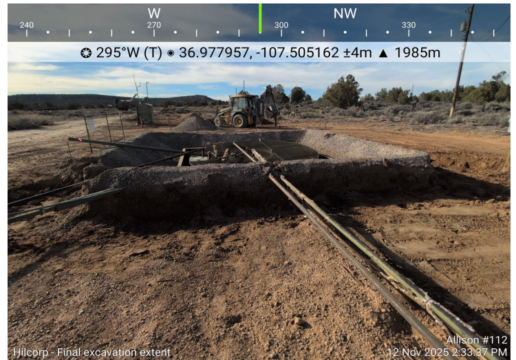
Photograph: 14 Description: Final Excavation Extent
