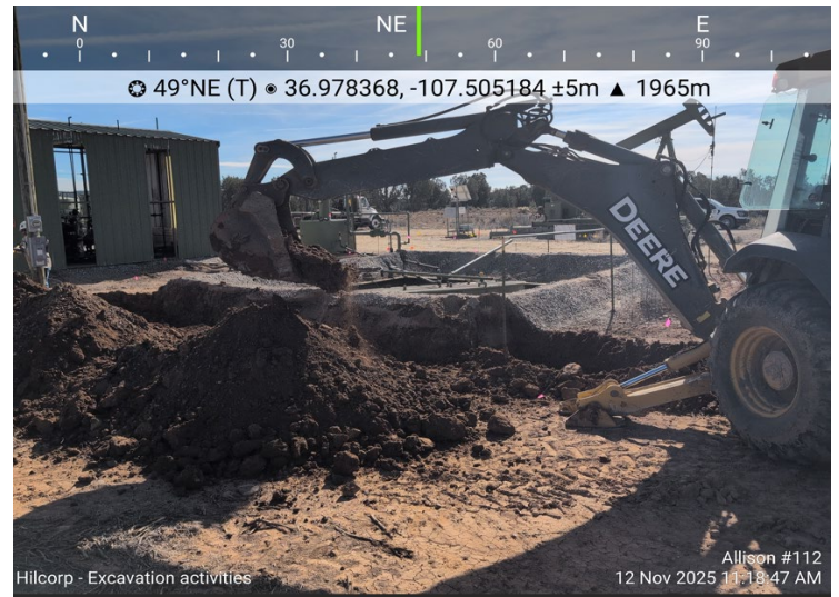
Photograph: 12 Date: 11/12/2025 Description: SS02, Southwest of BGT berm. View: Northeast
