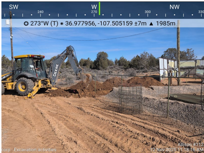
Photograph: 11 Date: 11/12/2025 Description: Excavation Activities View: West
