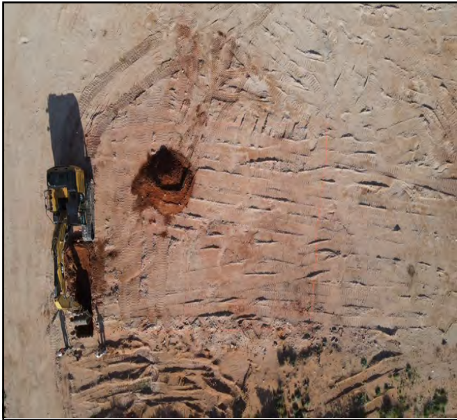
Aerial kickoff photos.
