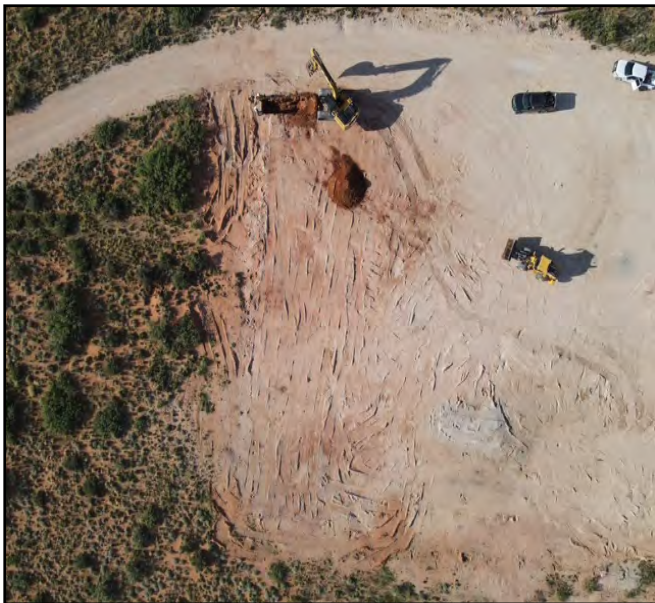
Aerial kickoff photos.
