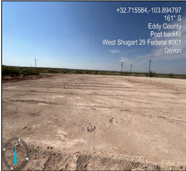
Photograph taken post excavation , facing south.
