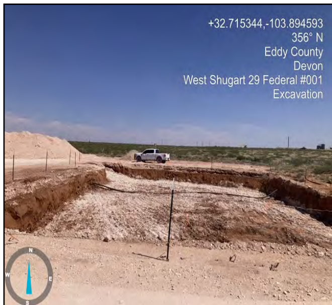
Photograph taken during the excavation process facing north.
