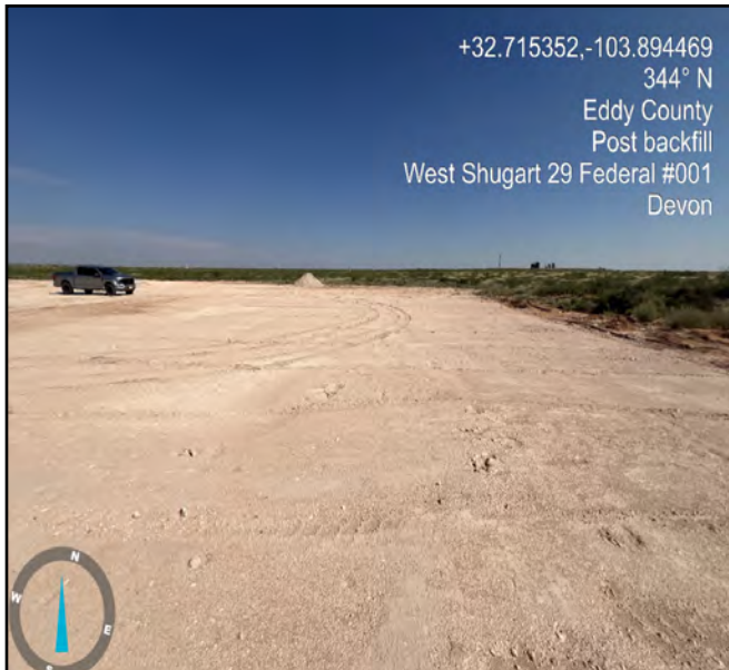
Photograph taken post excavation , facing north.
