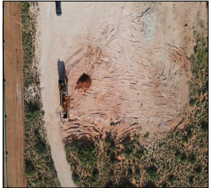
Aerial kickoff photos.
