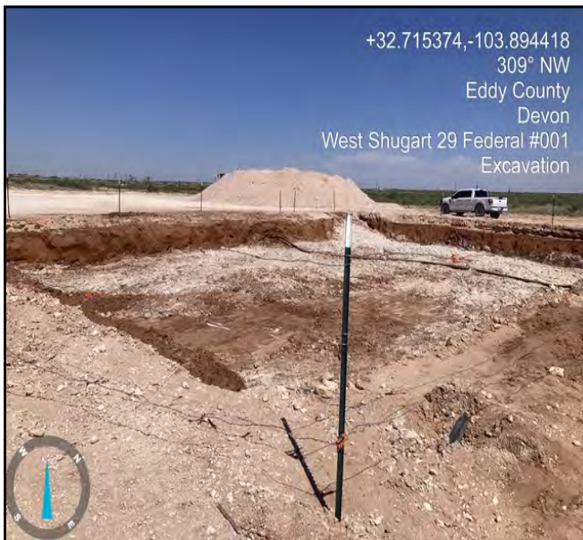
Photograph taken during the excavation process facing northwest.
