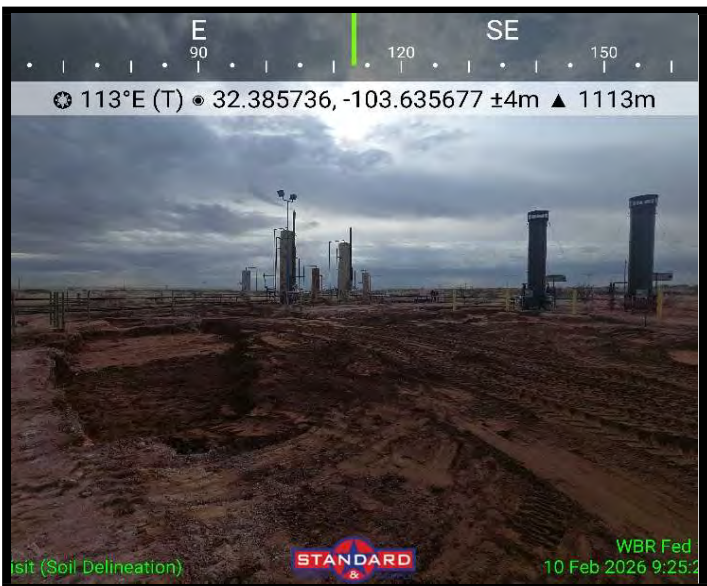
View of Excavation
