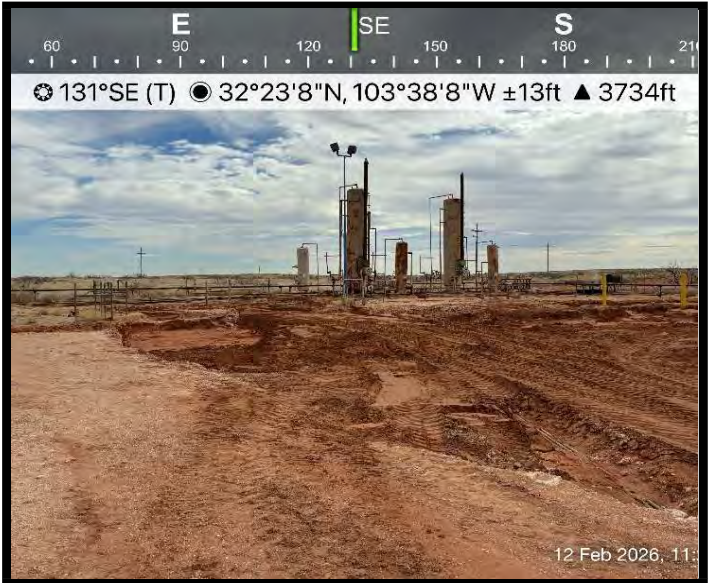
View of Excavation
