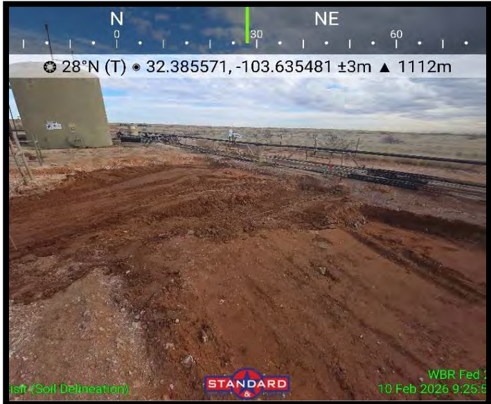
View of Excavation
