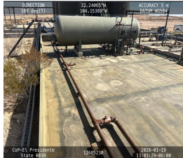
Photo 2 View of containment towards east.
