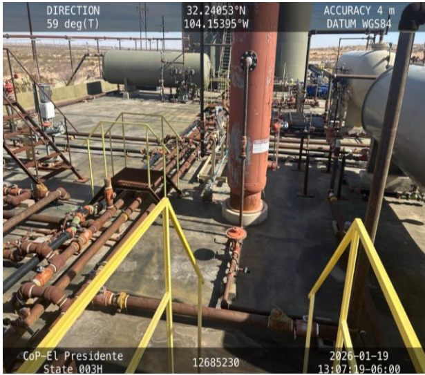
Photo 5 View of containment towards east.
