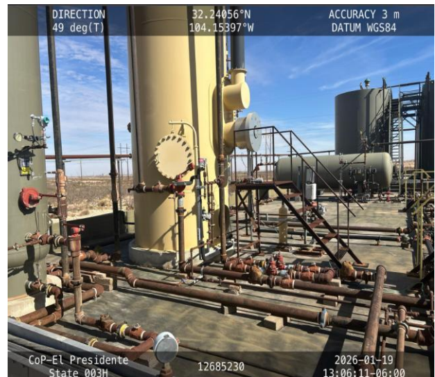
Photo 4 View of containment towards east.
