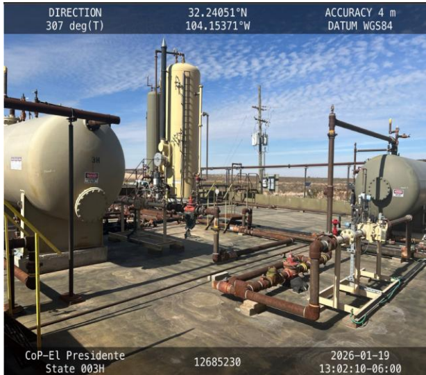
Photo 1 View of containment towards northwest.
