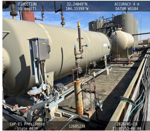
Photo 6 View of southeast corner of containment.
