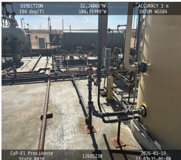
Photo 3 View of containment towards south.
