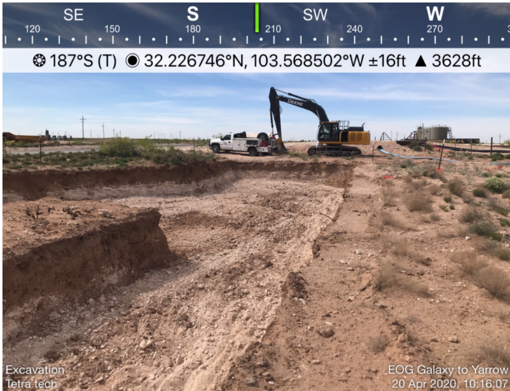
View South, area of Bottom holes 80-86
