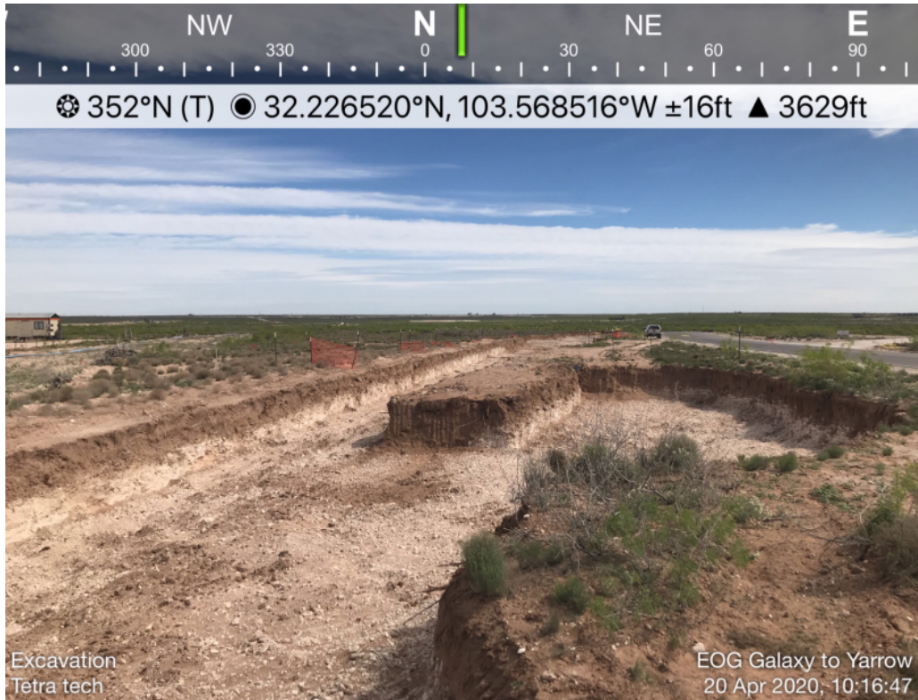
View North, area of Bottom holes 61-80
