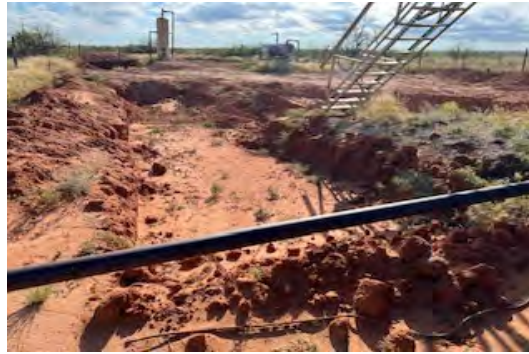
View to E of excavation N of tank (10/15/25).
