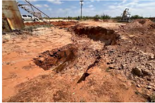
View to NE of excavation S of tank (4/23/25).
