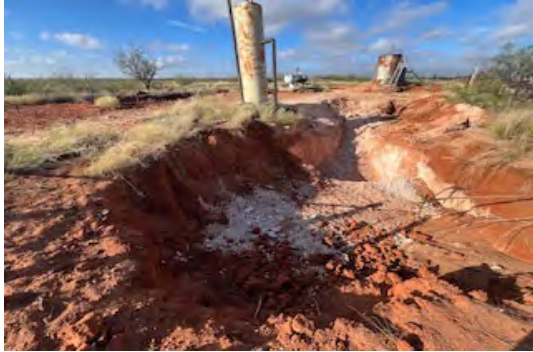
View to W of excavation N of treater (10/15/25).
