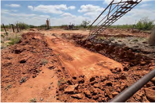
View to E of excavation N of tank (4/23/25).
