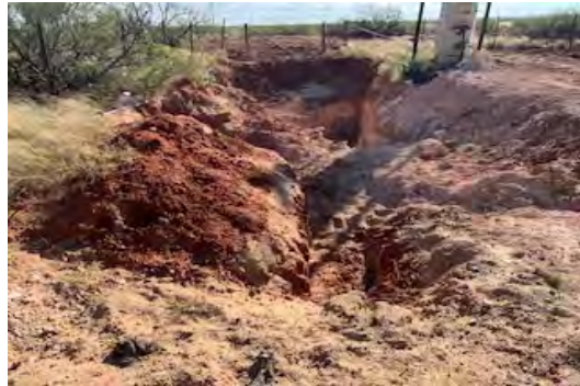
View to E of excavation N of treater (10/15/25).
