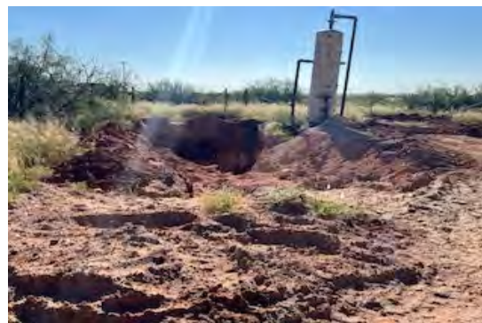
View to E of excavation N of treater (8/21/25).
