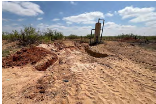
View to E of excavation N of treater (4/23/25).
