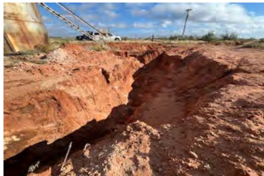
View to N of excavation E of tank (10/15/25).
