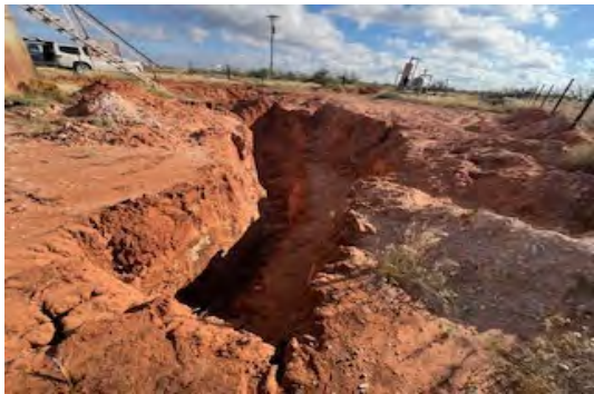
View to NE of excavation at tank (10/15/25).
