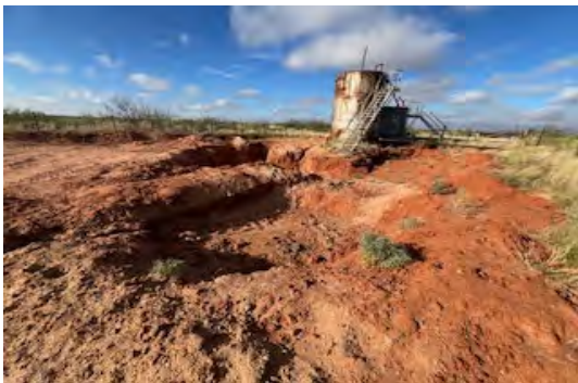
View to SW of excavation at tank (10/15/25).
