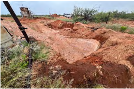
View to W of excavation N of treater (6/25/25).
