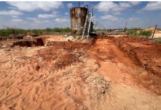
View to W of excavation at tank (4/23/25).
