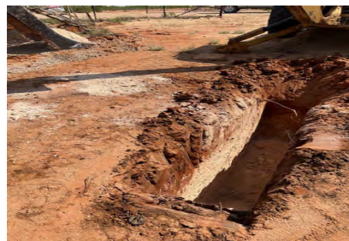
View of sample location S-2 (7/25/24).
