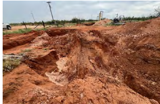
View to E of excavation around tank (6/25/25).
