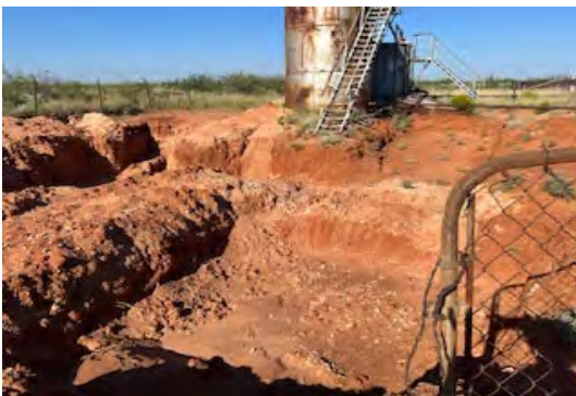
View to W of excavation around tank (8/21/25).
