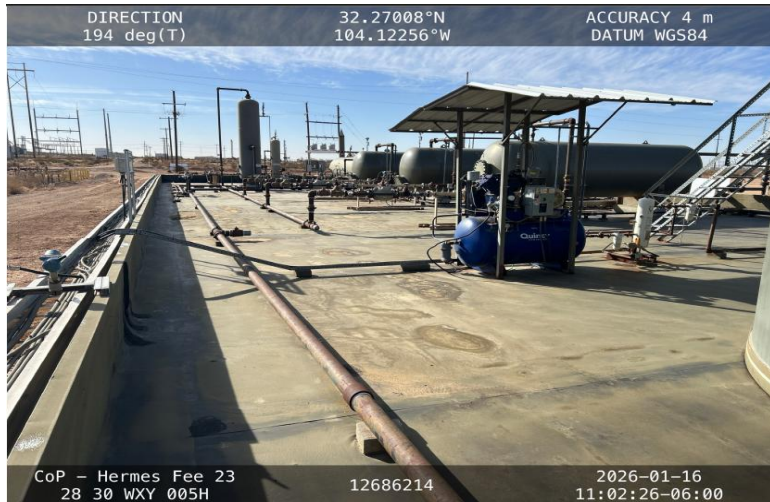
Photo 5 View of east side secondary containment towards south.
