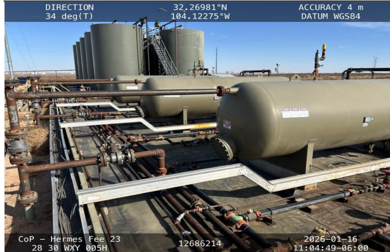
Photo 8 View of west side secondary containment towards north.
