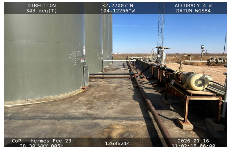
Photo 4 View of east side secondary containment towards north.
