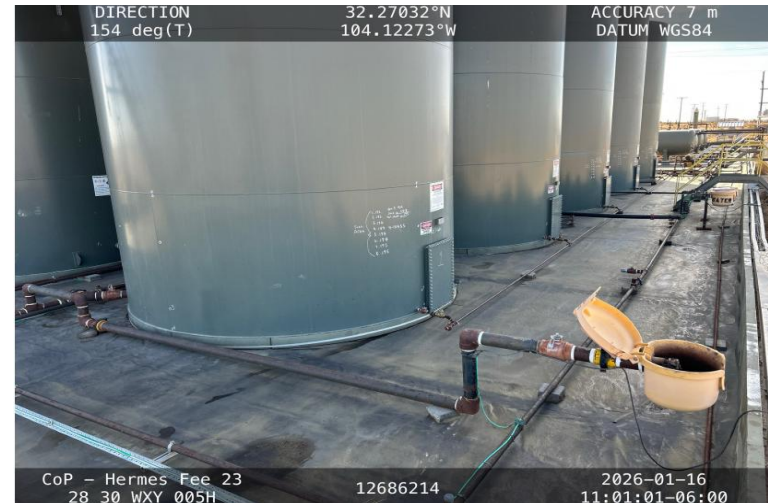
Photo 2 View of west side secondary containment towards south.
