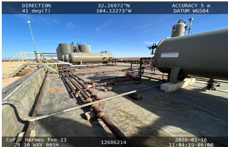
Photo 7 View of west side secondary containment towards north.
