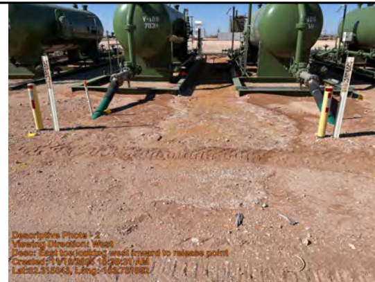
Viewing Direction: West
