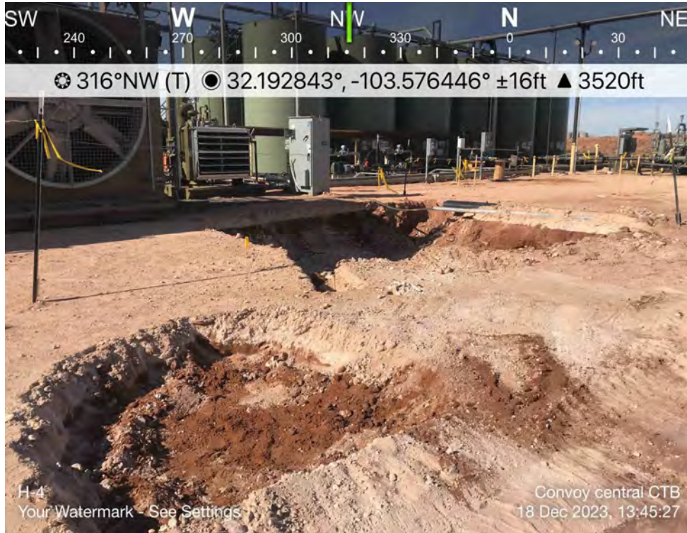
View of Remediation Activities – View Northwest
