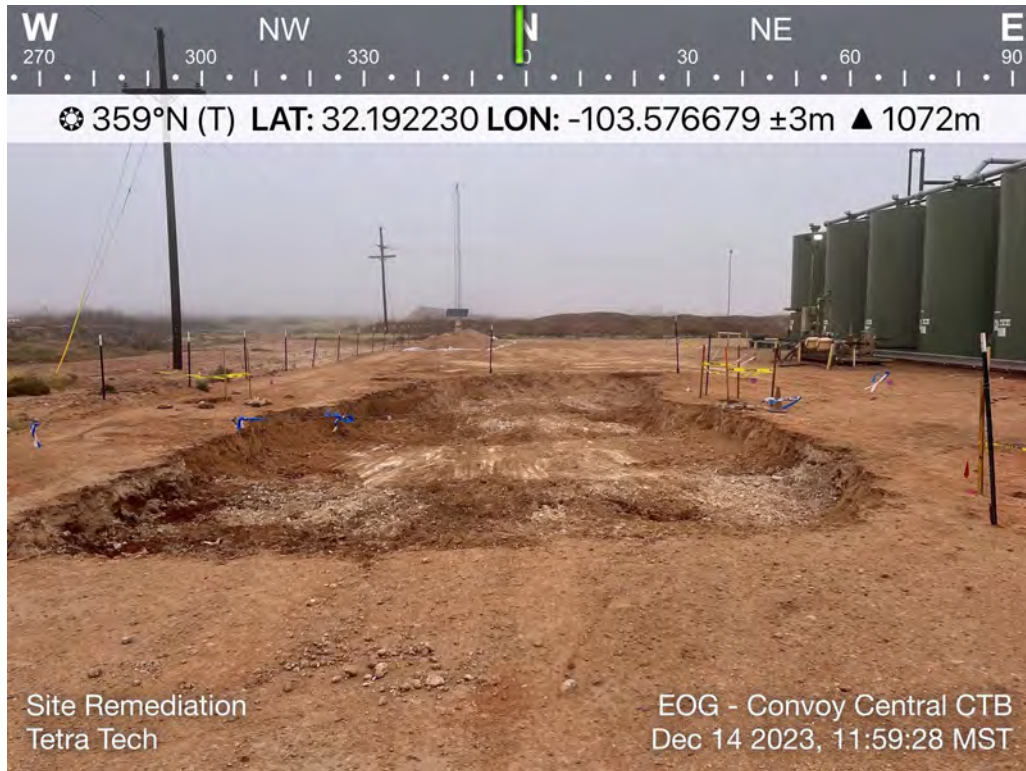
View of Remediation Activities – View North
