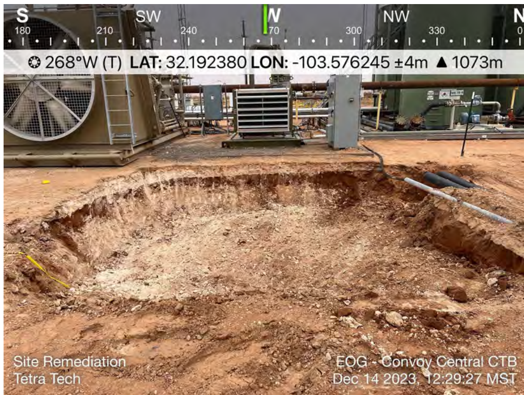
View of Remediation Activities – View West
