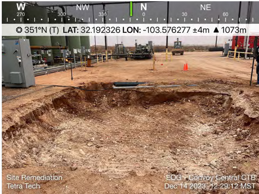
View of Remediation Activities – View North
