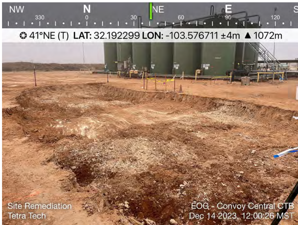
View of Remediation Activities – View Northeast
