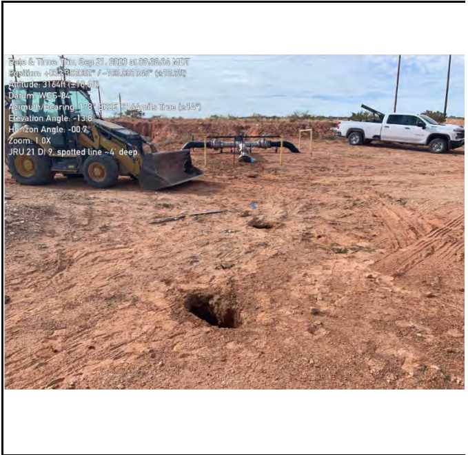
Photograph 2 Date: 9/21/2023 Description: Hydro-vac spotting produced water pipeline View: South
