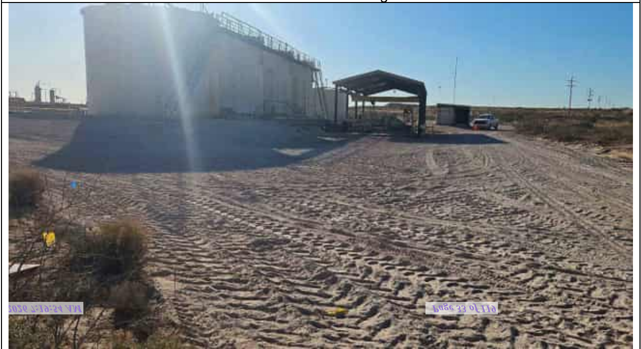
Photos of the site backfilled following the remediation
