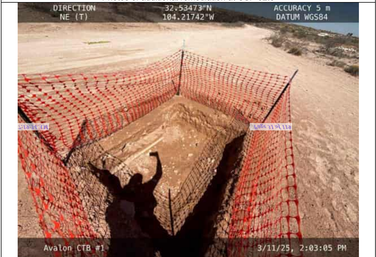
Photos of additional remediation at S-SW-01.2
