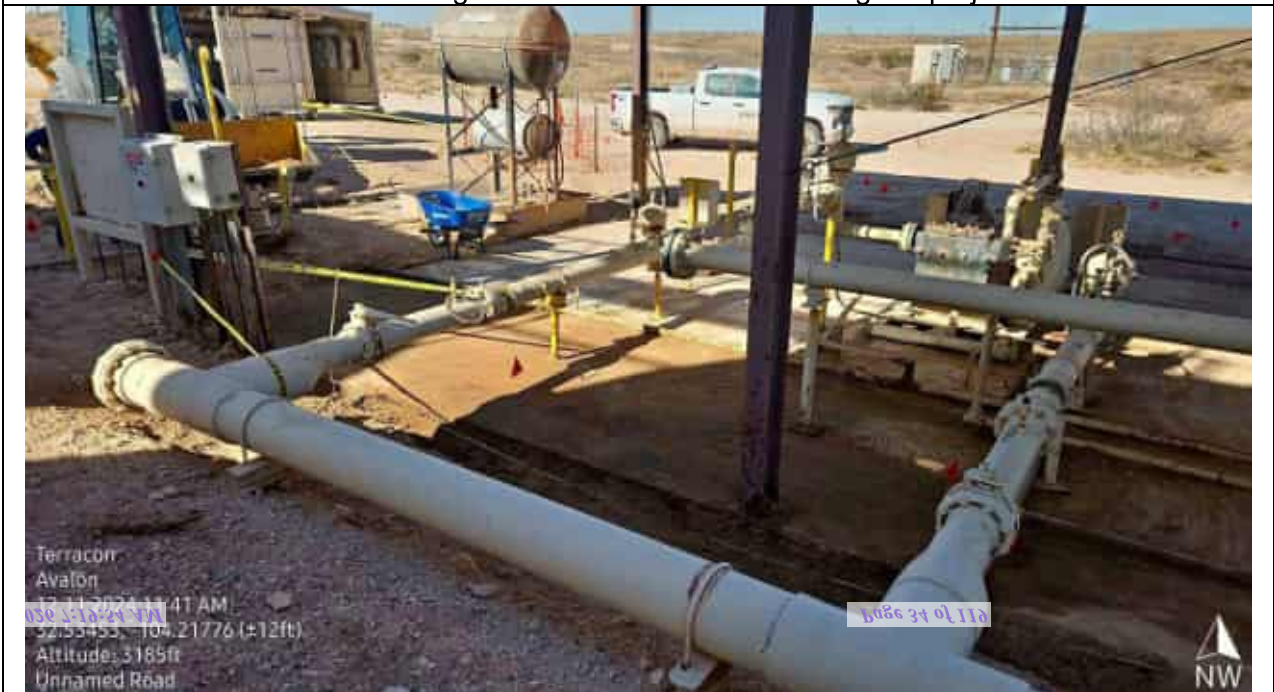
Photo demonstrating concrete coverage following additional Hydro-excavation / cleaning.
