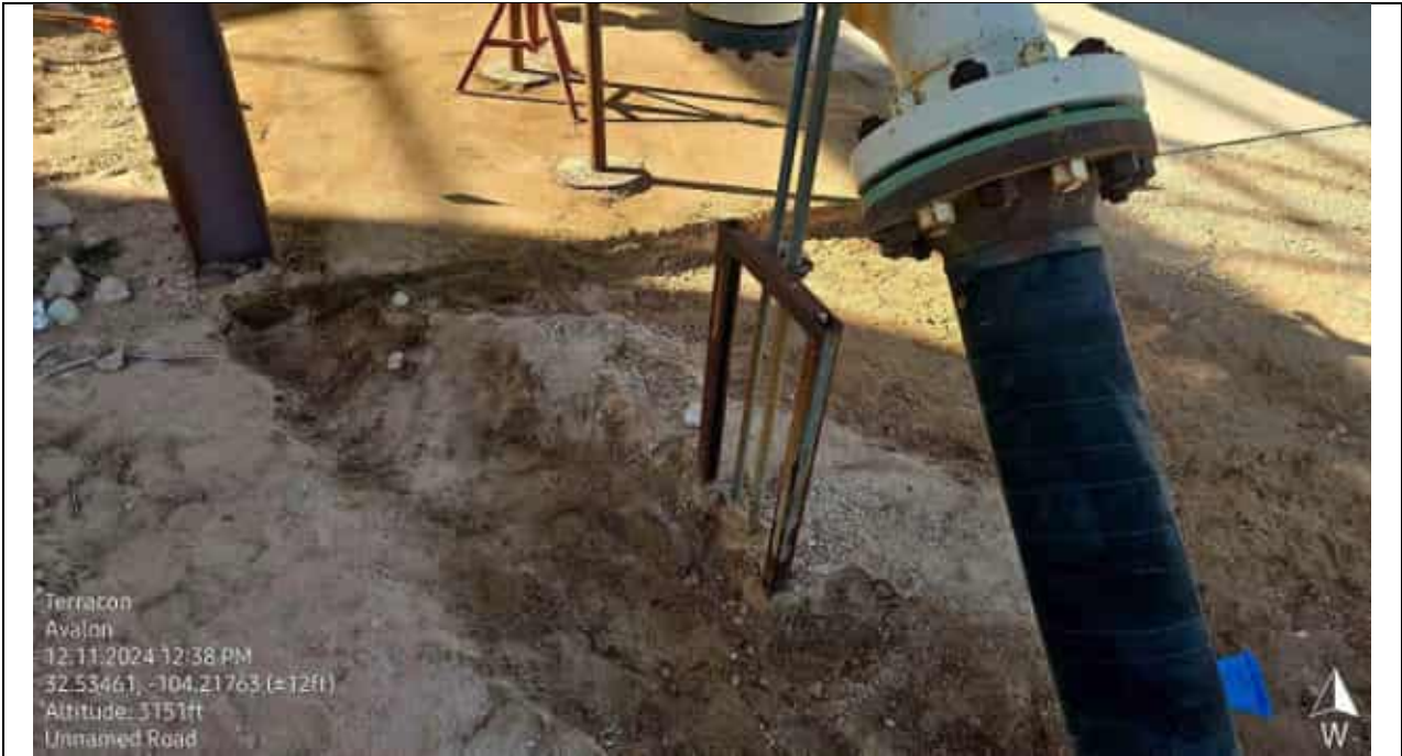
Photo demonstrating the extent of concrete coverage at project site.
