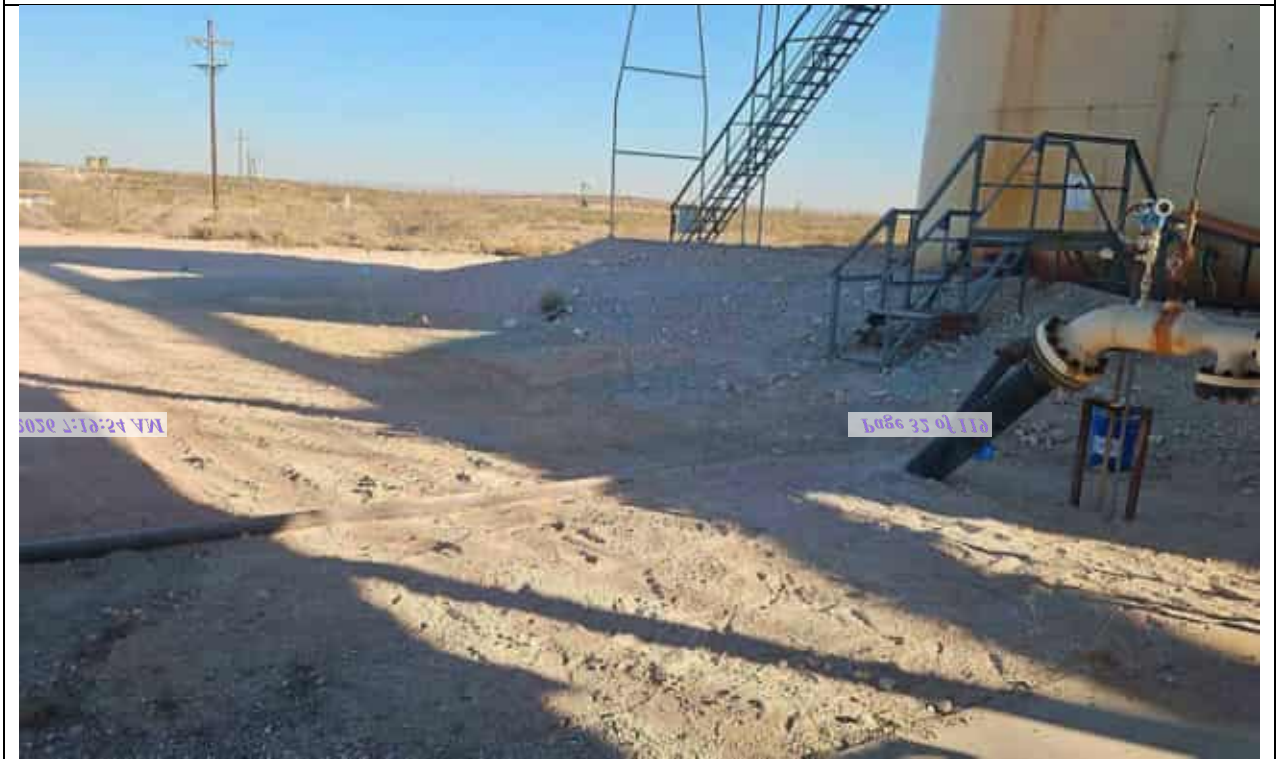
Photos of the site backfilled following the remediation
