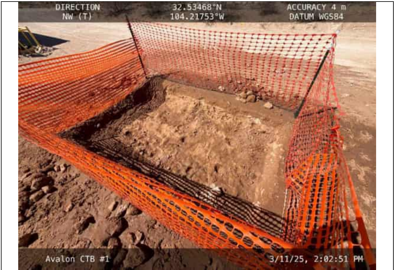
Photos of additional remediation at CSF-02.3
