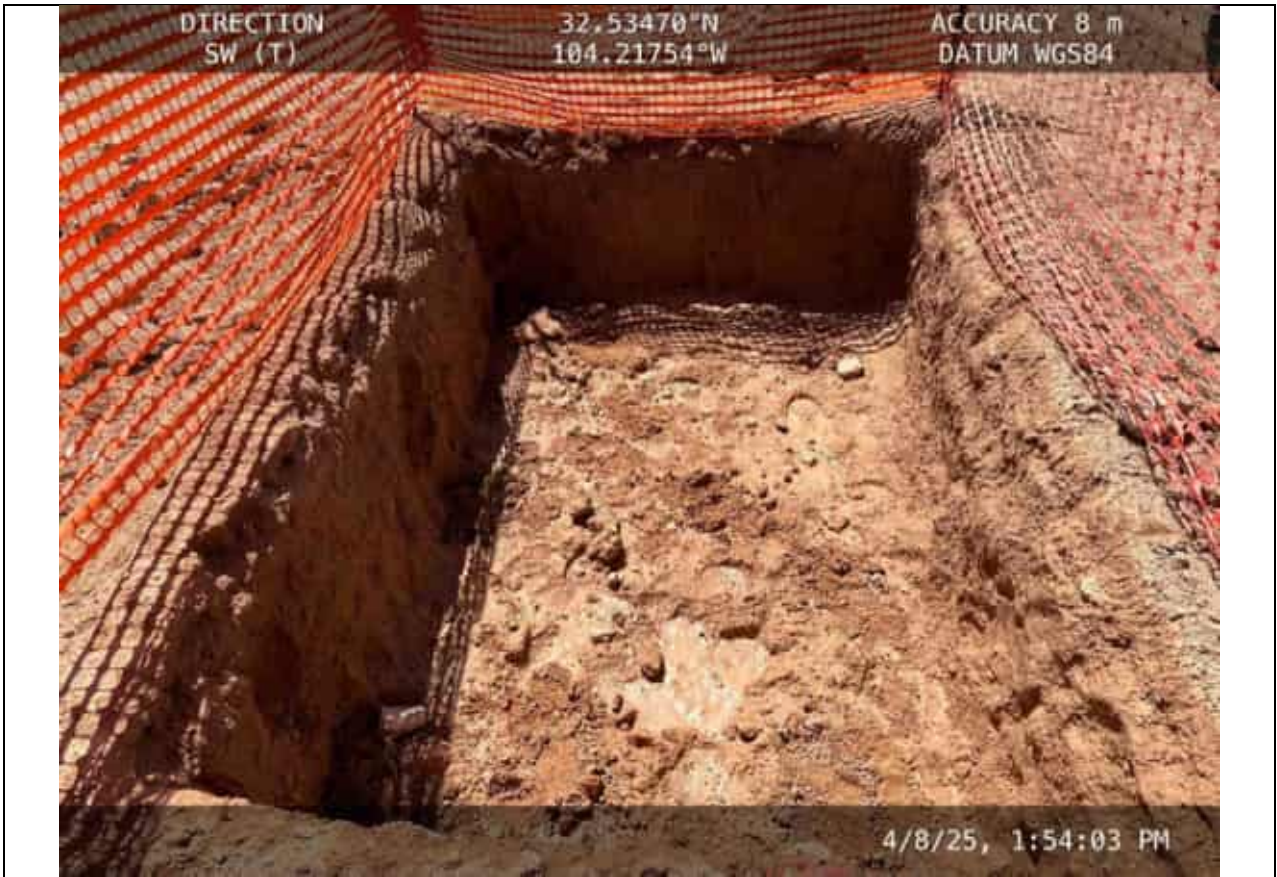
Photos of additional remediation at CSF-02.3
