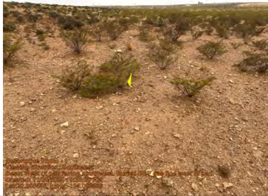
West of pad facing southwest. Buried DCP gas line west of pad.
