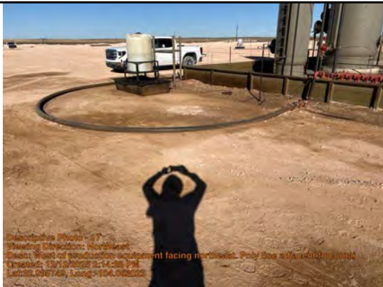
West of production equipment facing northeast. Poly line adjacent to containment.
