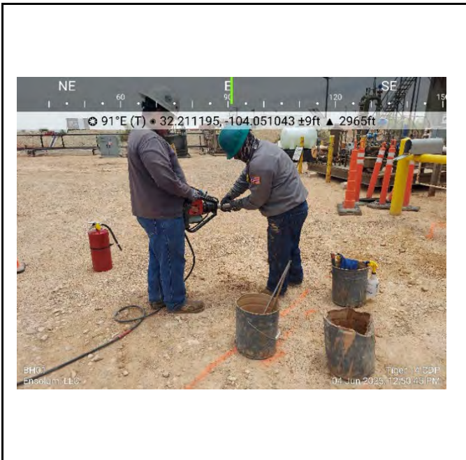
Photograph 7 Date: 6/4/2025 Description: Delineation (BH01) View: East
