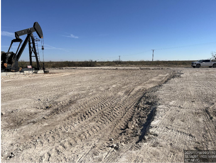
Excavated area, viewing northeast.
