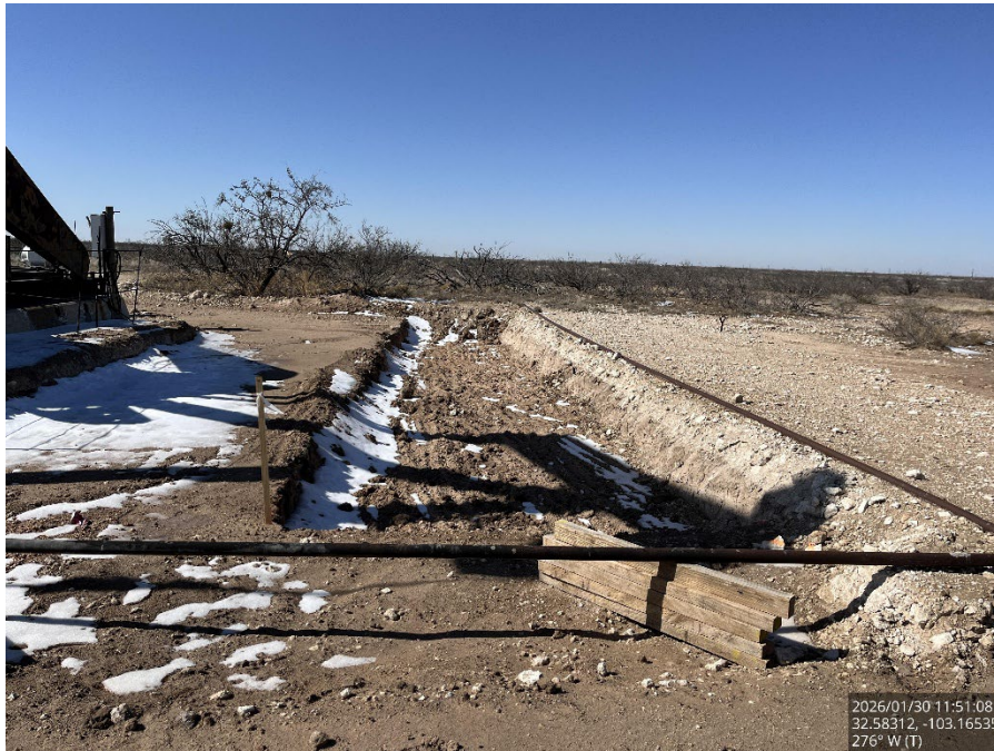
Excavated area, viewing west.
