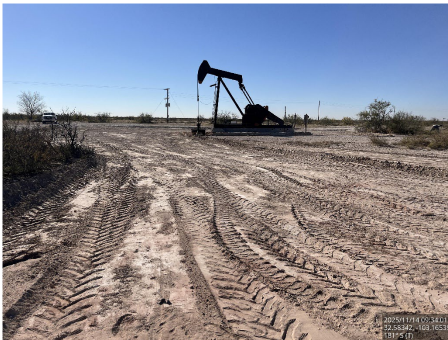
Excavated area, viewing south.
