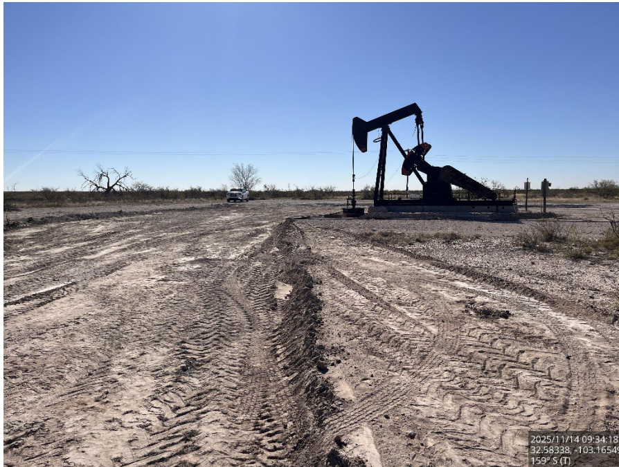
Excavated area, viewing south.
