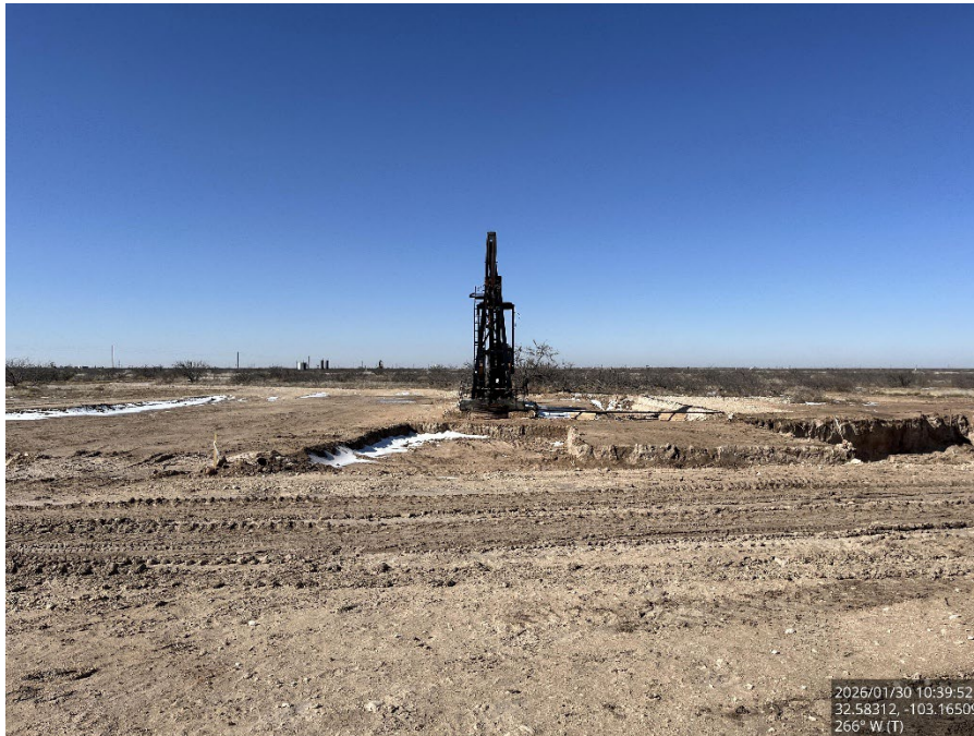
Excavated area, viewing west.
