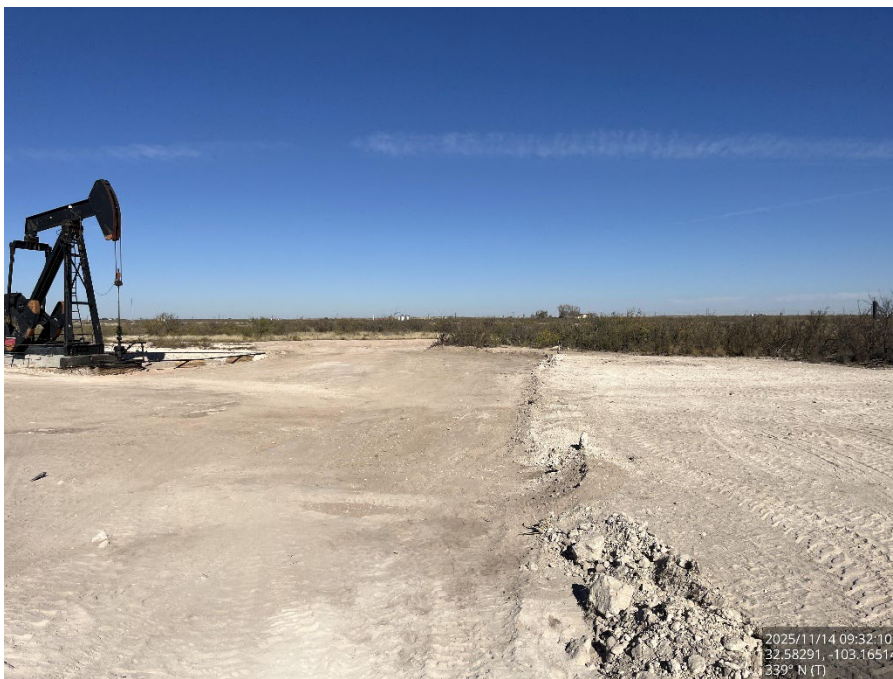
Excavated area, viewing north.
