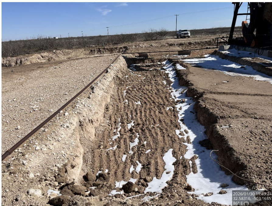
Excavated area, viewing east.
