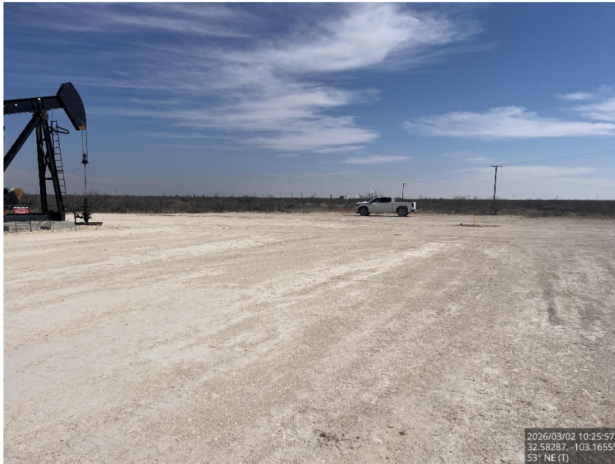
Backfilled excavation, viewing northeast.
