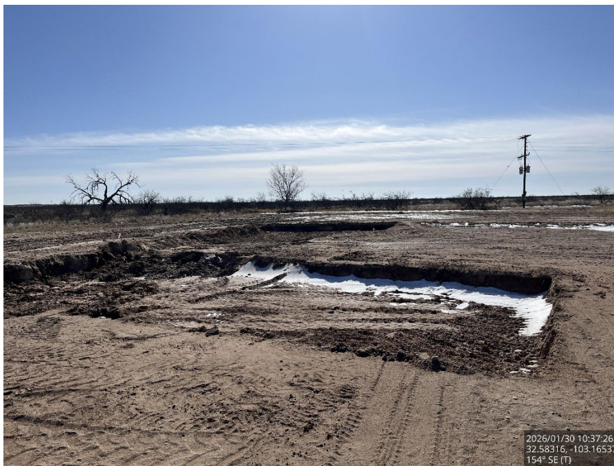
Excavated area, viewing southeast.
