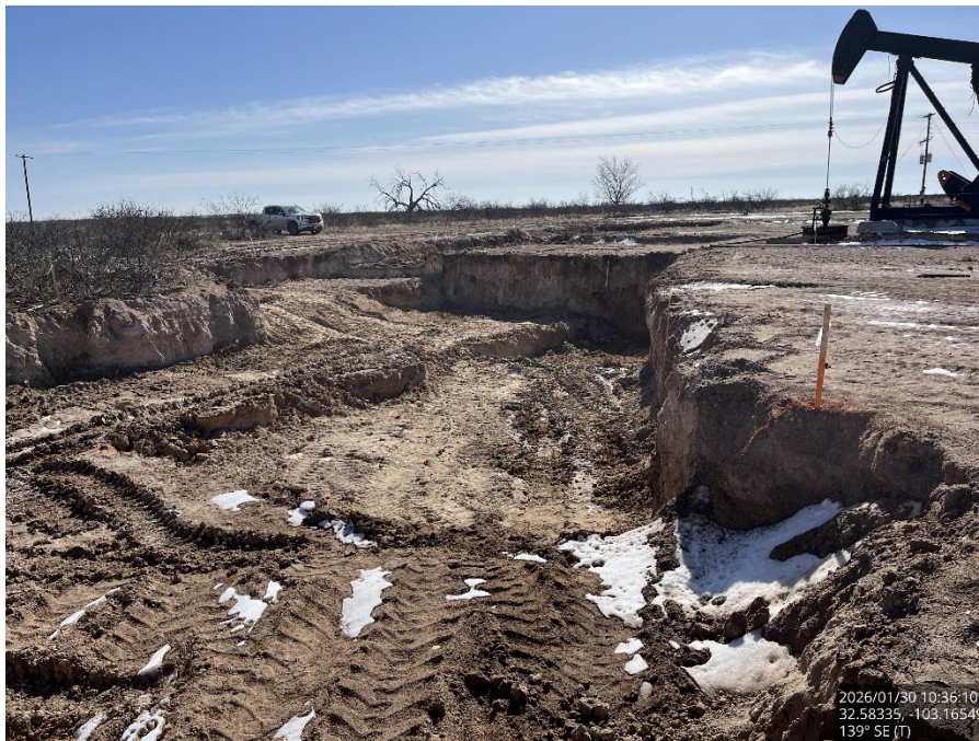
Excavated area, viewing southeast.
