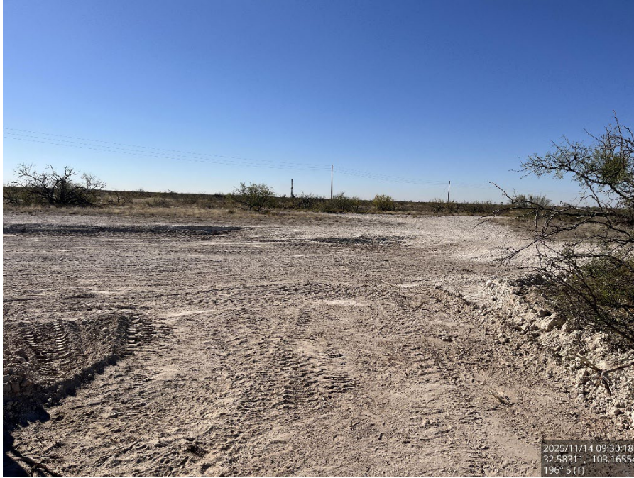
Excavated area, viewing south.
