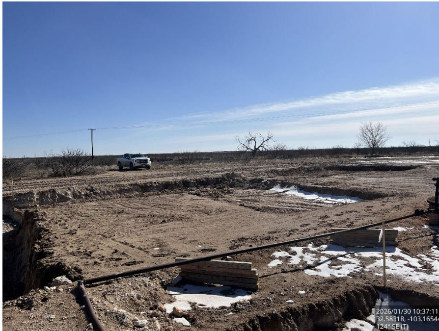
Excavated area, viewing southeast.
