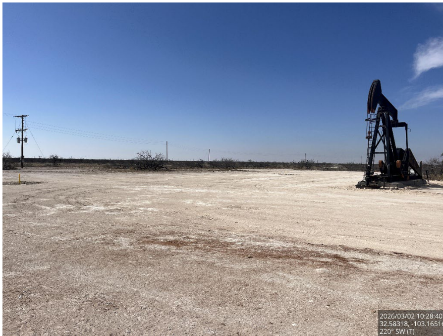
Backfilled excavation, viewing southwest.
