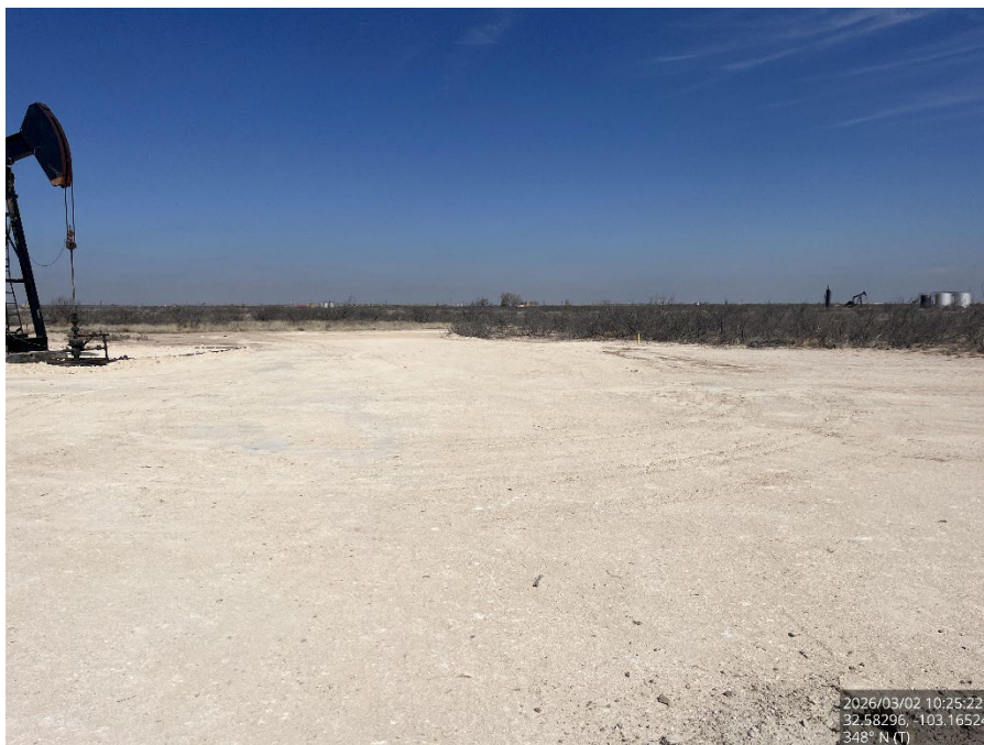
Backfilled excavation, viewing north.
