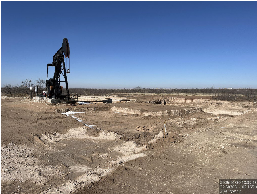
Excavated area, viewing northwest.
