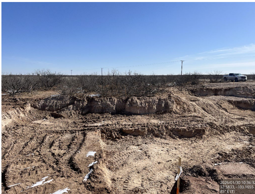
Excavated area, viewing east.
