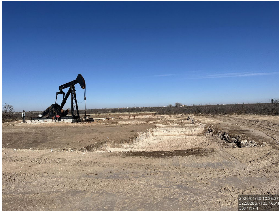
Excavated area, viewing north.
