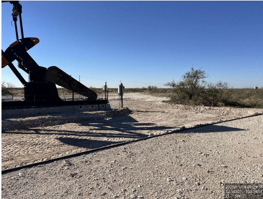
Excavated area, viewing southwest.
