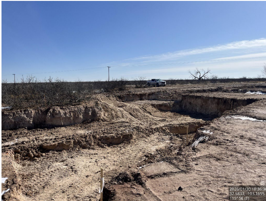
Excavated area, viewing southeast.
