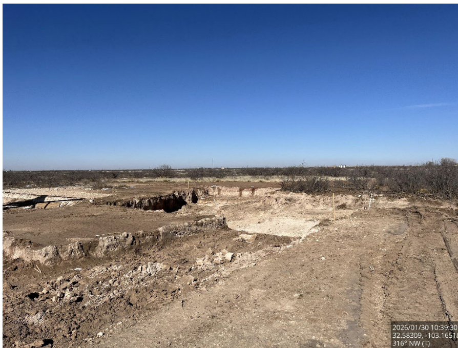
Excavated area, viewing northwest.
