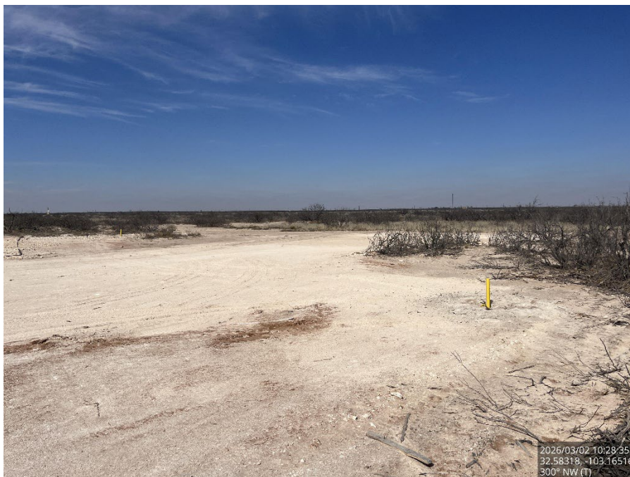
Backfilled excavation, viewing northwest.
