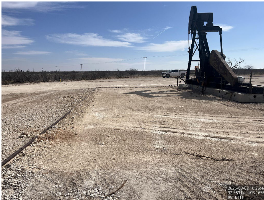
Backfilled excavation, viewing east.
