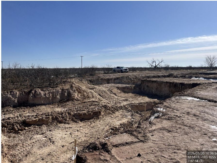
Excavated area, viewing southeast.
