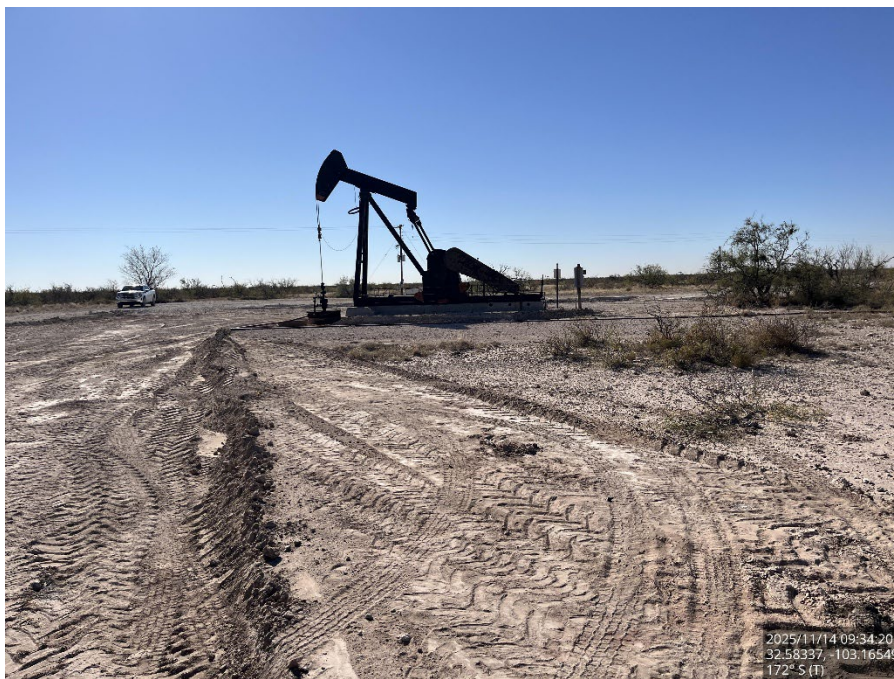
Excavated area, viewing south.
