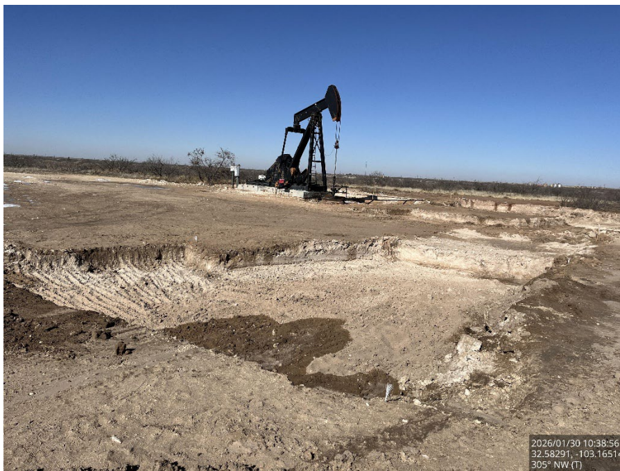
Excavated area, viewing northwest.
