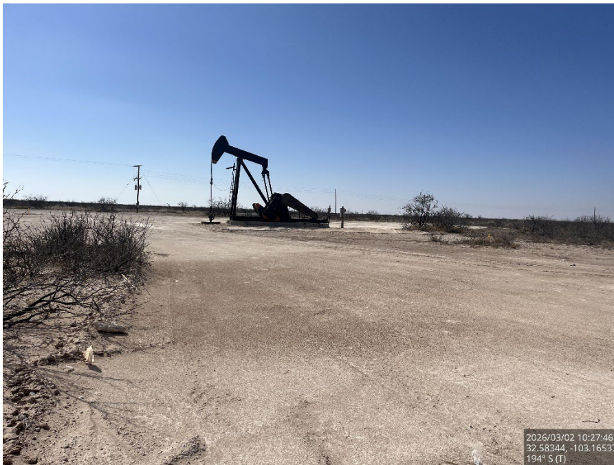
Backfilled excavation, viewing south.
