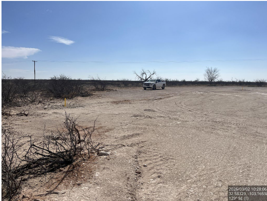
Backfilled excavation, viewing southeast.
