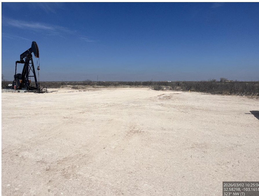
Backfilled excavation, viewing northwest.
