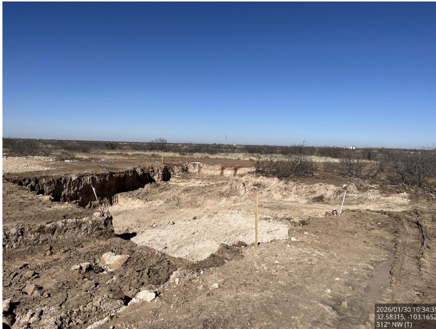
Excavated area, viewing northwest.
