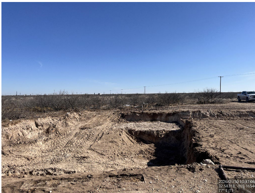
Excavated area, viewing east.
